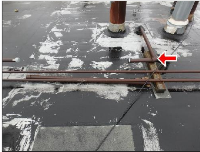
Abandoned Piping Should Be Removed
