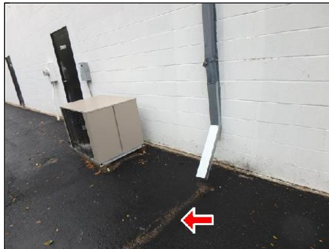
Premature Failure of Seal Coating
