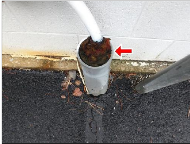
Improper and Inadequate Sealant
