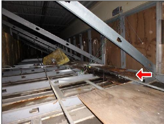
Active Moisture Penetration Inside Mansard Overhang
