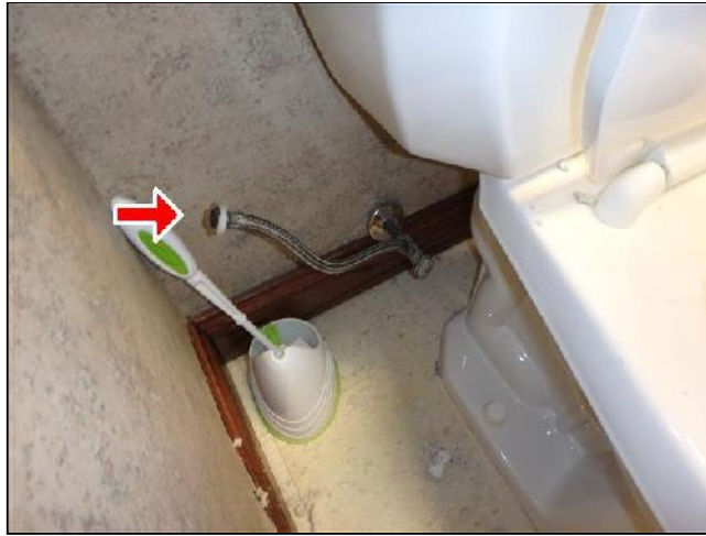
Disconnected Toilet Water Supply
