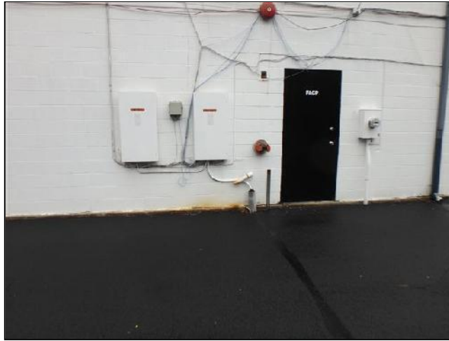
Sloppy Low Voltage Wiring
