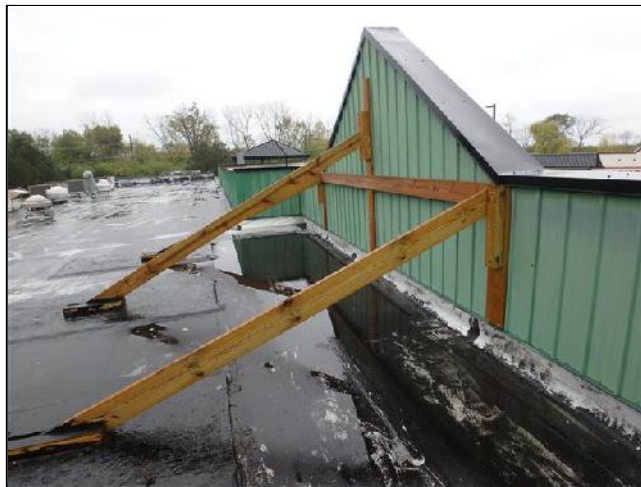
False Parapet Support System
