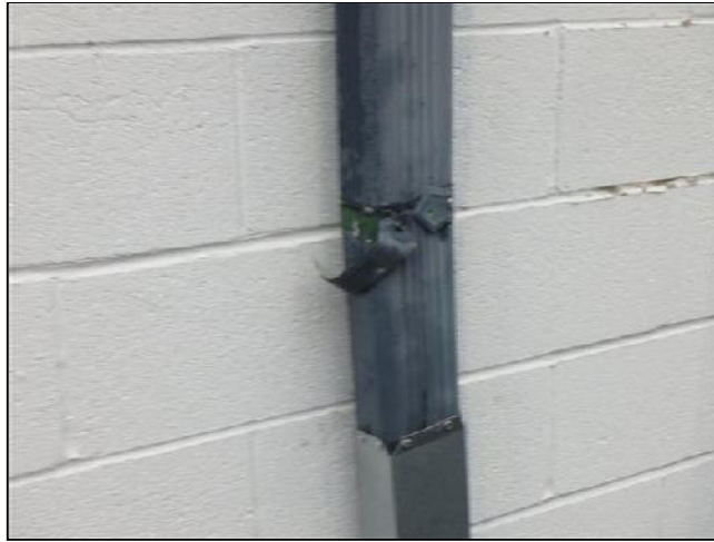
Loose and Damaged Downspout
