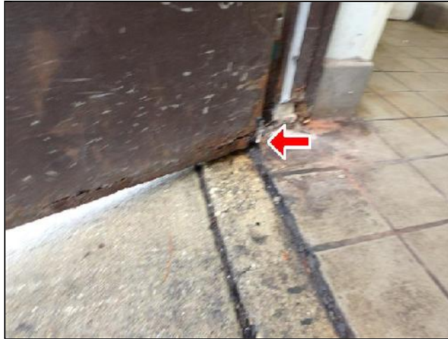
Badly Corroded Exterior Door
