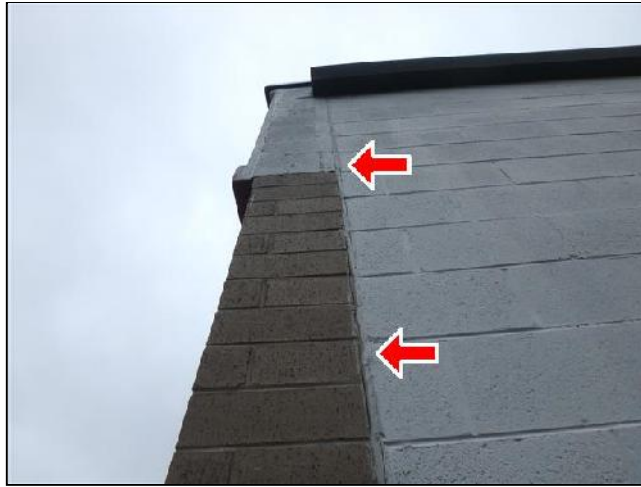
Caulking Failure
