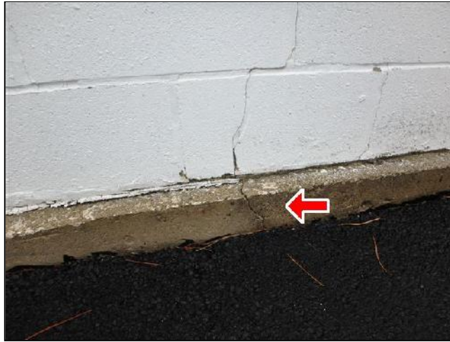
Typical Shrinkage/Settling Crack
