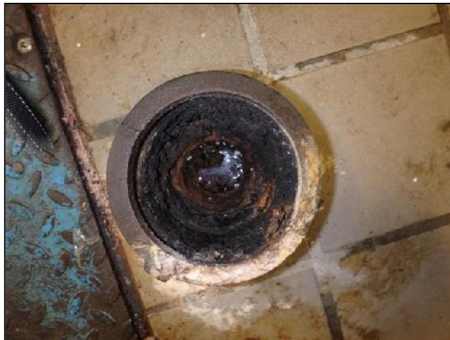
Caked On Grease at Floor Drain
