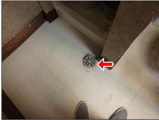
Taped Over Floor Drain
