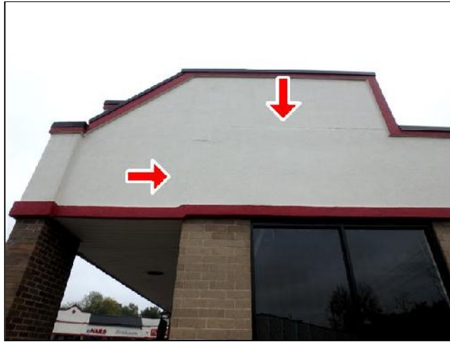
Cracking at EIFS Wall Cladding
