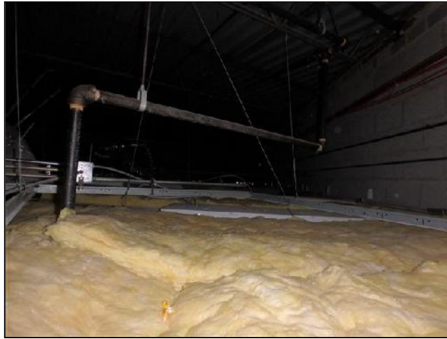
Insulation Above Suspended Ceiling
