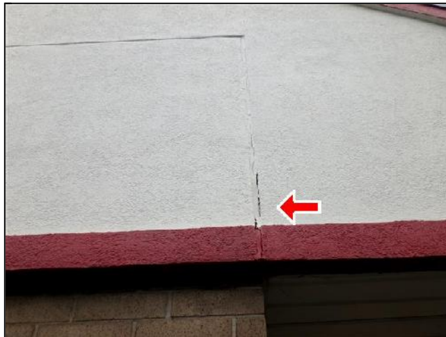
EIFS Cracking at Opposite Corner
