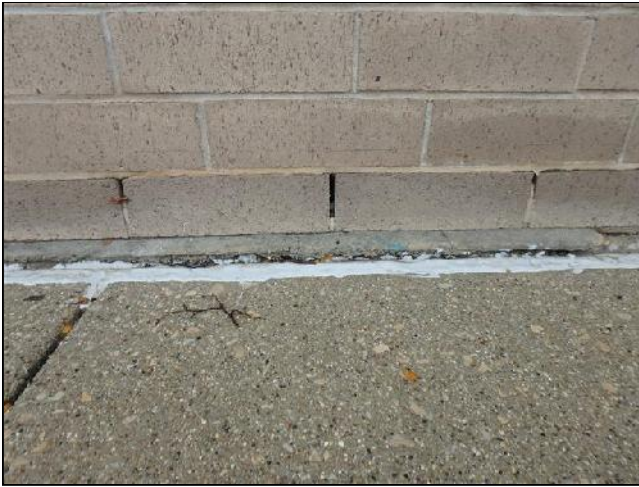
Open Masonry Wall Weep Holes
