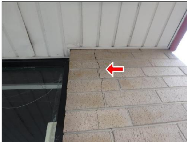
Cracking Through Multiple Brick Units
