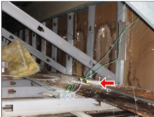
Exposed and Dangerous Wiring
