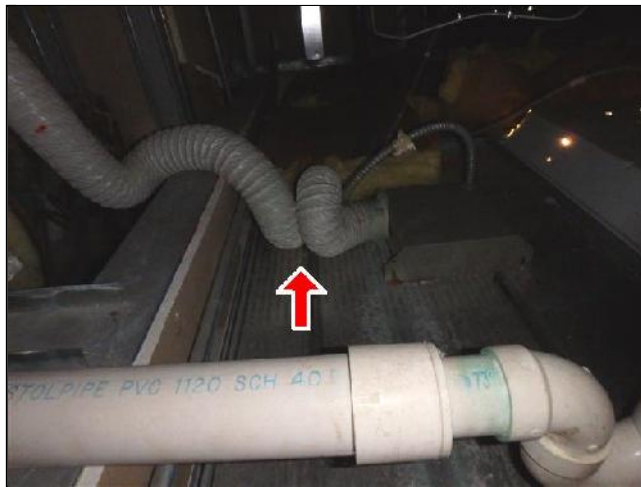
Woefully Inadequate Airflow
