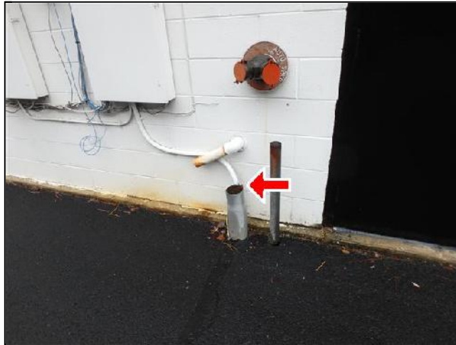
Exterior Rated Sealant Material Needed
