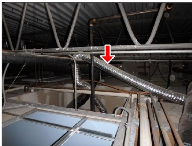
Poor Airflow Characteristics and Prohibited Material
