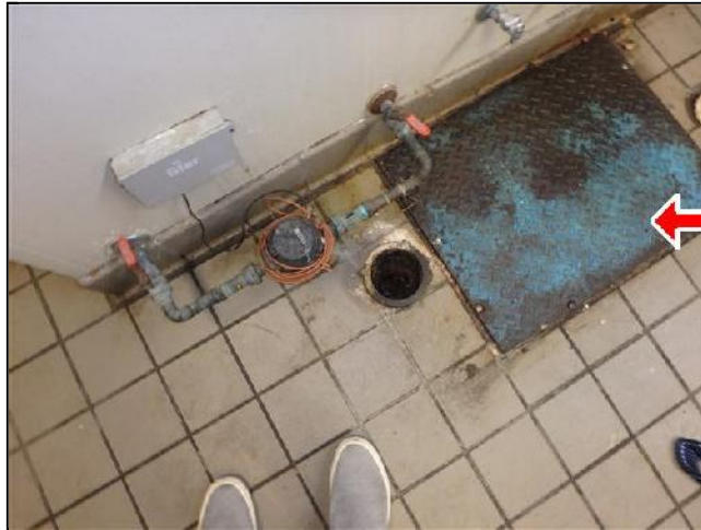
Grease Interceptor Cleaning Recommended
