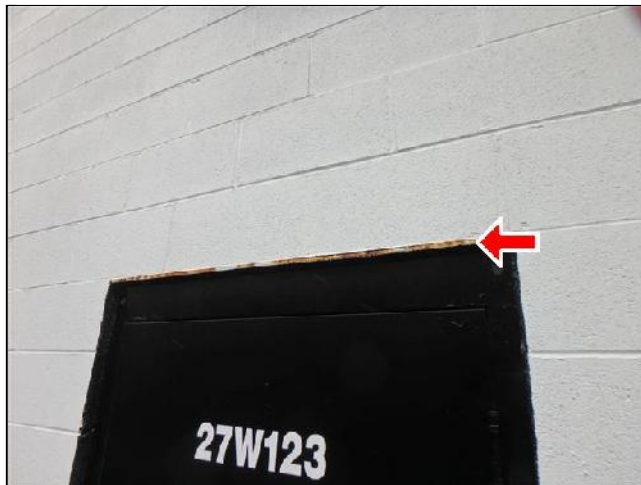
Lintel Corrosion from Moisture Exposure
