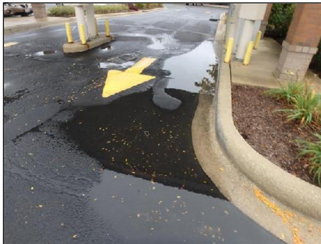
Pavement Ponding
