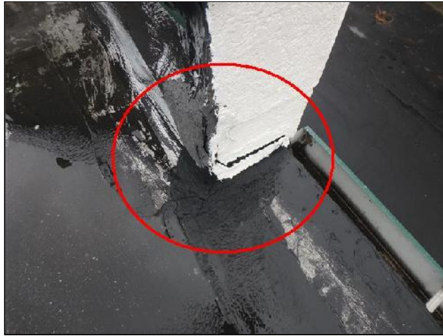
Parapet Wall Breaches
