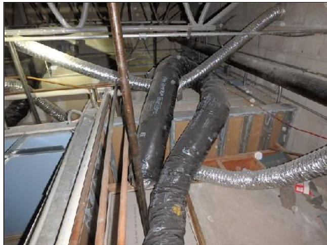
Seriously Defective Flex Duct Installation
