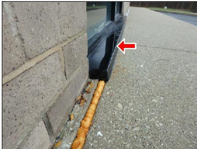
Failure to Slope
