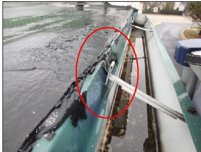
Loose Gutter Support System
