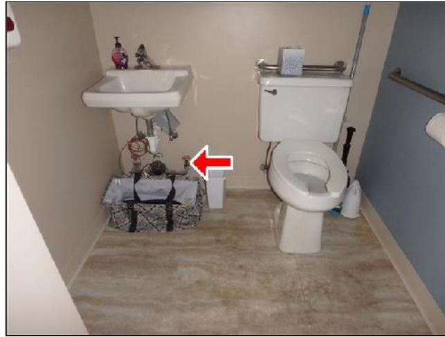
Missing Insulation and Inadequate Access
