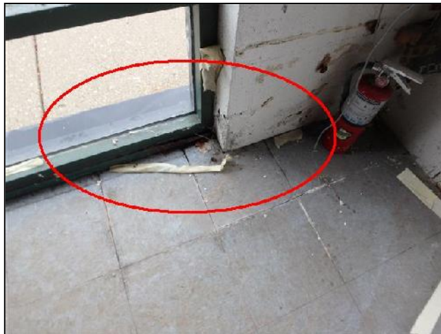
Moisture Damage
