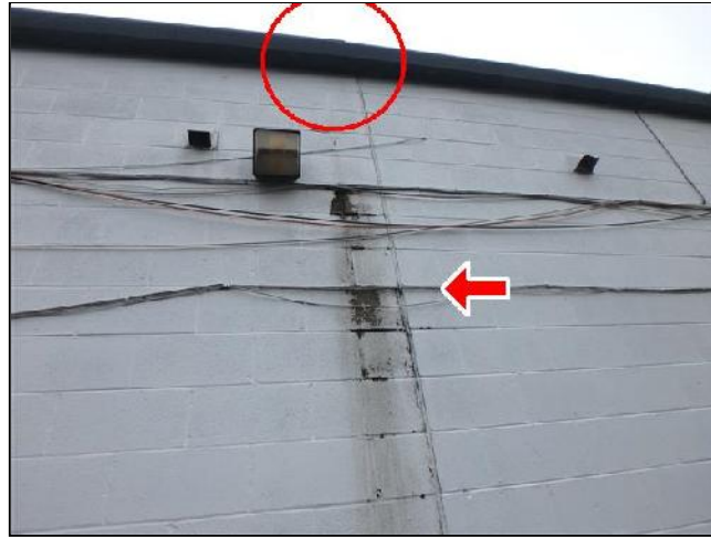
Leaking Gutter Causing Masonry Damage
