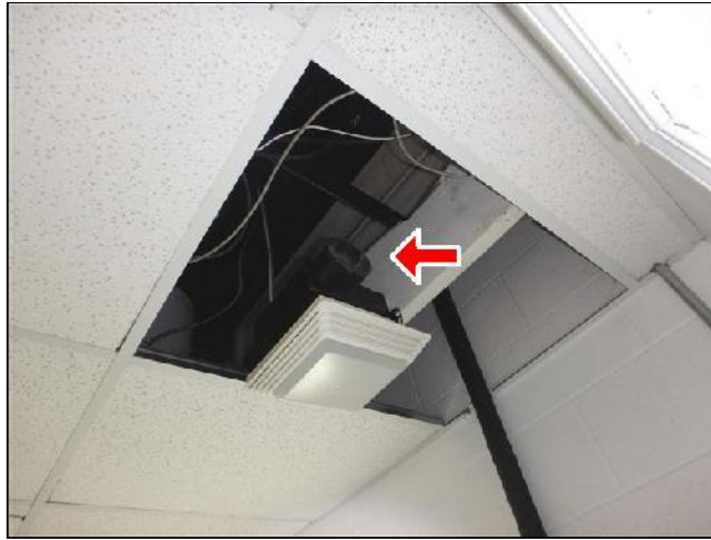
Missing Vent Tubing
