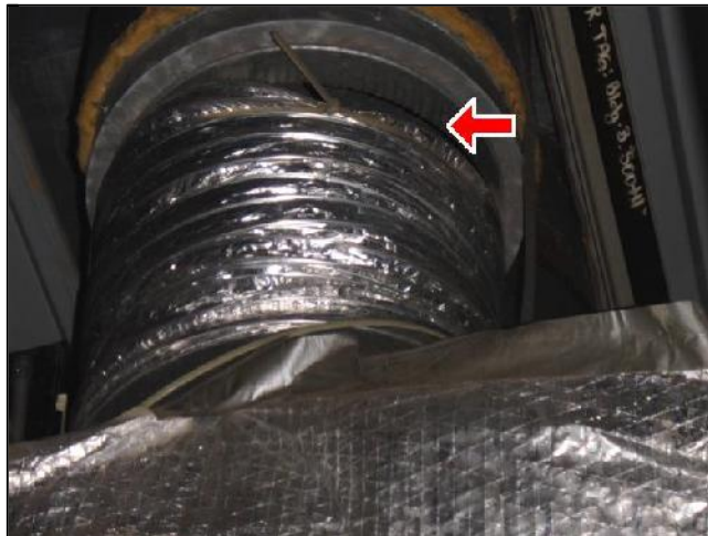
Partially Disconnected Duct Connection
