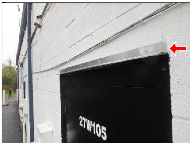
Drip Cap Flashing
