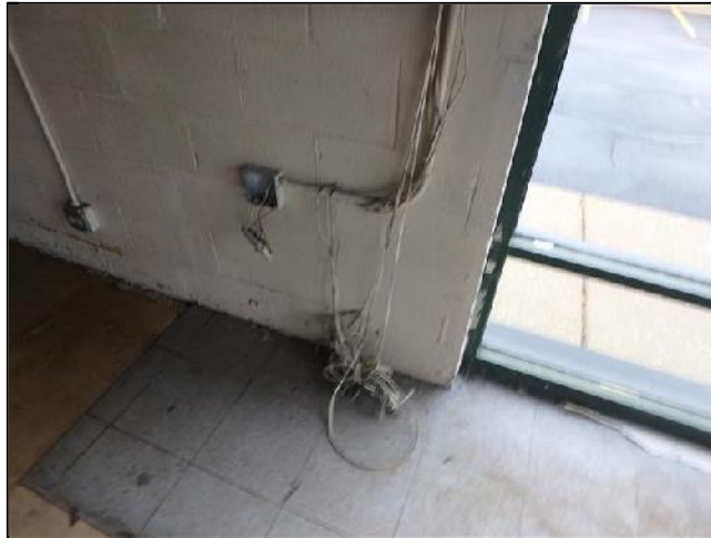
Defective Wiring
