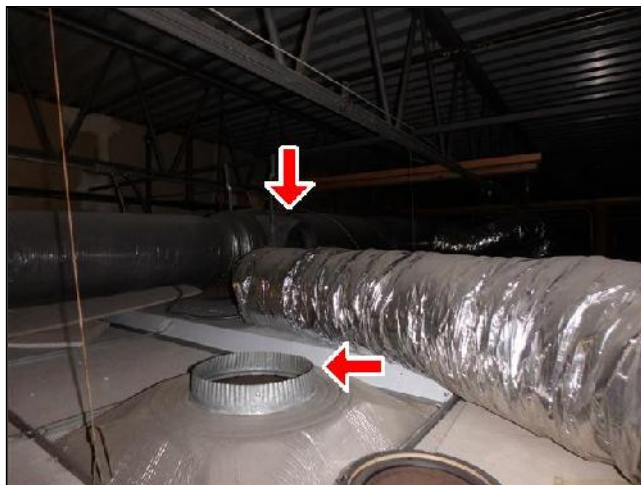
Disconnected Duct
