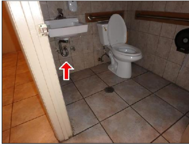
Missing Pipe Insulation
