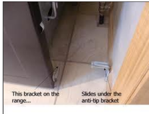
L. Item 2(Picture) Kitchen Range Anti-Tipping Bracket
