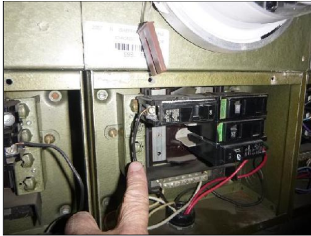
E. Item 8(Picture) over fused circuit
