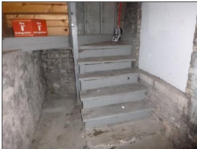
J. Item 1(Picture) missing handrail
