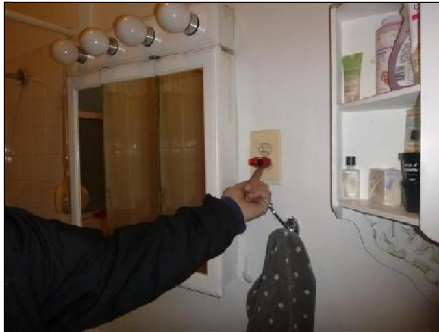
E. Item 21(Picture) Missing Shock Protection
