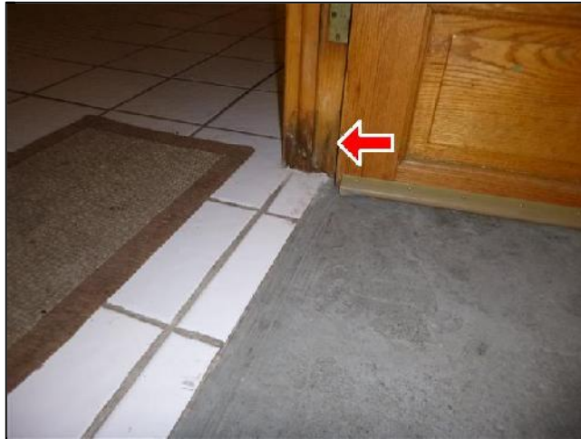
D. Item 7(Picture) evidence of previous moisture events
