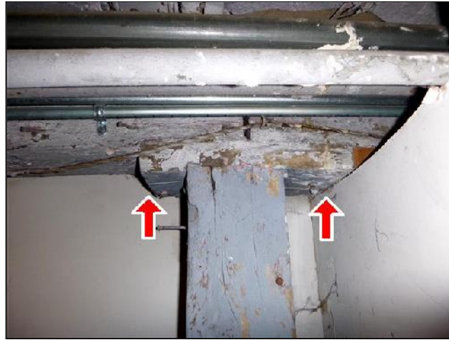
D. Item 1(Picture) wood fibers being crushed
