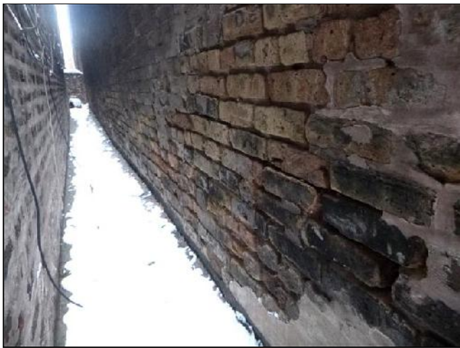
A. Item 1(Picture) exterior wall mortar erosion
