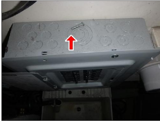
E. Item 18(Picture) improper electrical panel cover fastener
