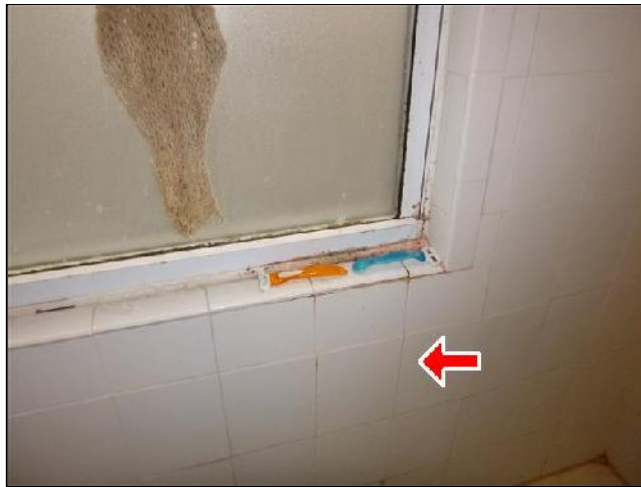
J. Item 4(Picture) moisture damaged tile and tile substrate
