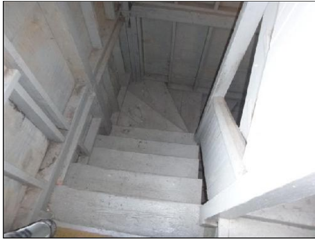
J. Item 3(Picture) Missing Handrail
