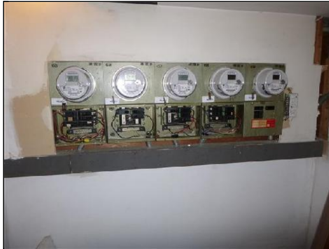
E. Item 9(Picture) undersized panels
