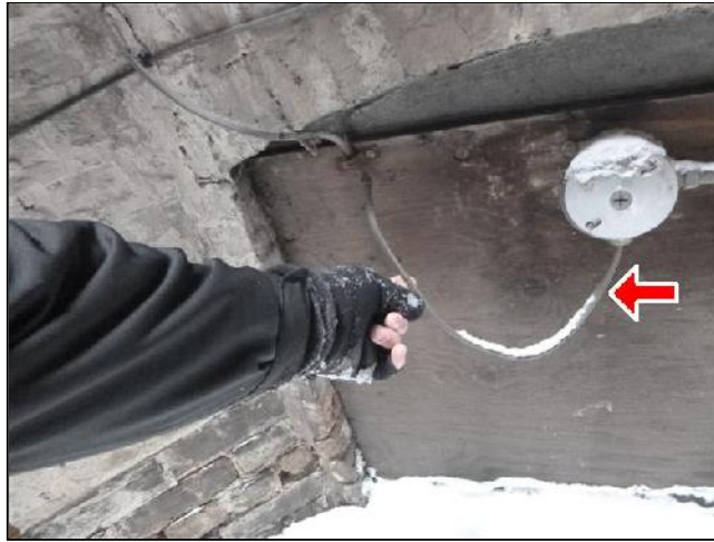
E. Item 4(Picture) dangerous wiring
