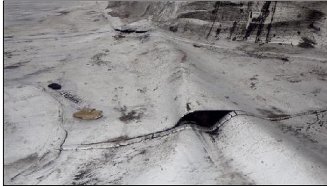
C. Item 3(Picture) extreme blistering/buckling of modified bitumen roof covering with resulting seam failure
