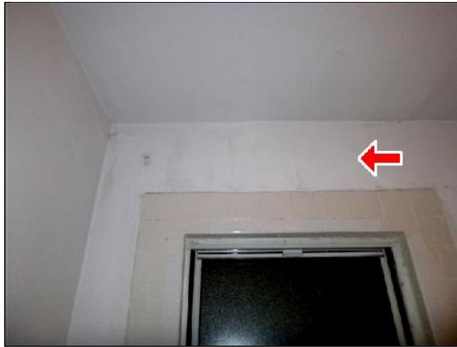
H. Item 5(Picture) Mold Growth Due to Inadequate Ventilation
