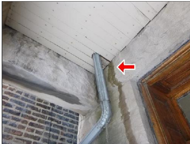
C. Item 1(Picture) leaking gutter/downspout
