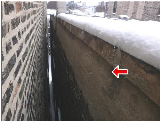
A. Item 5(Picture) parapet wall parging
