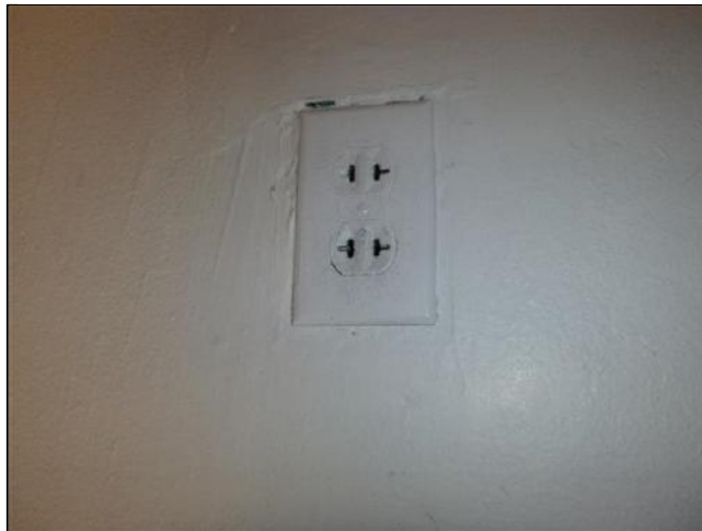
E. Item 12(Picture) obsolete two-pronged receptacle
