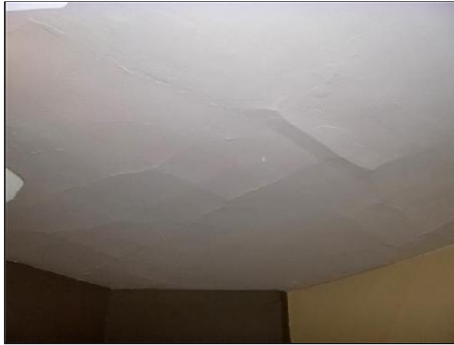
J. Item 6(Picture) Plaster is Heavy and Dangerous When Loose!
