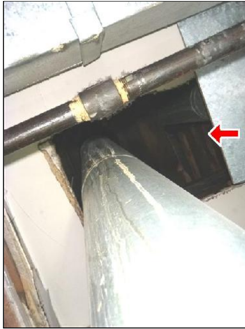
H. Item 6(Picture) missing insulation and air/fire barrier
