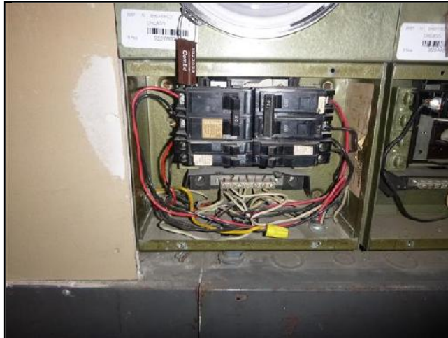
E. Item 7(Picture) half-size breakers
