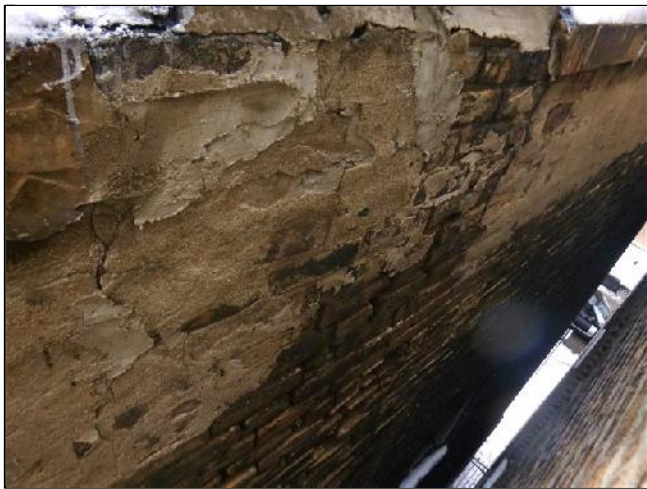
A. Item 2(Picture) deteriorated and improperly patched masonry parapet wall
