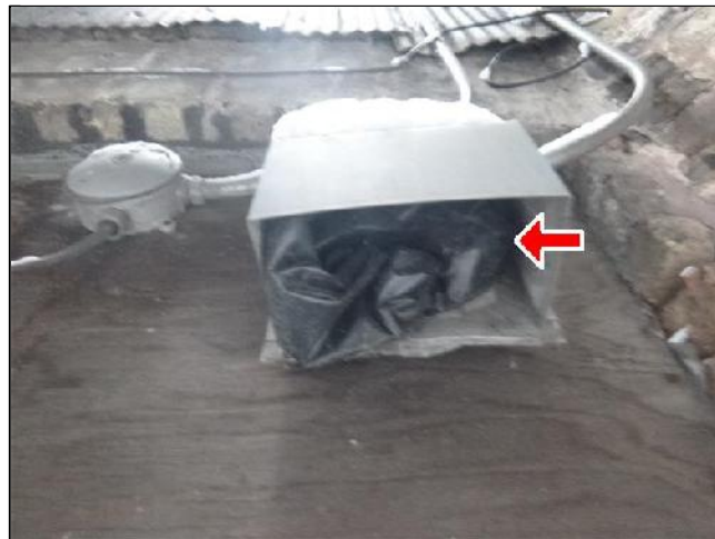
H. Item 3(Picture) blocked vent damper
