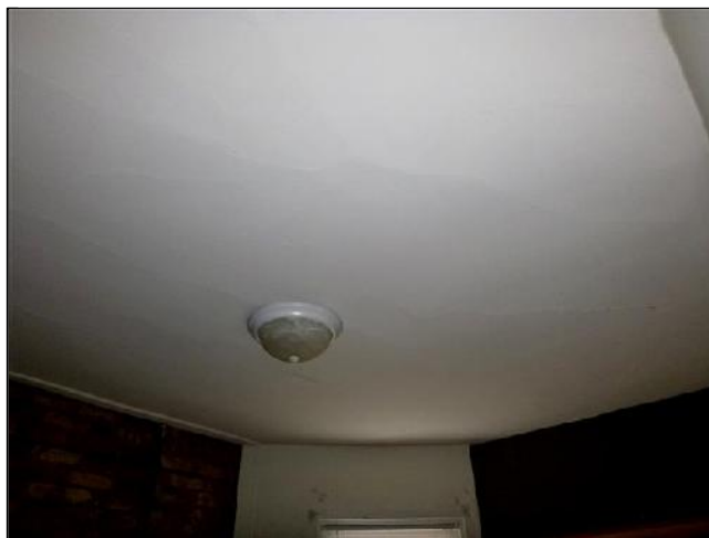
J. Item 5(Picture) badly deteriorated ceiling plaster
