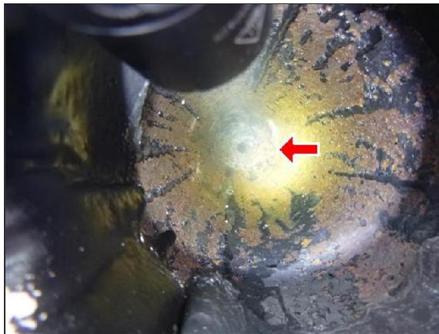
F. Item 2(Picture) blocked vent stack
