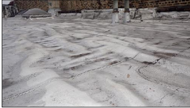
C. Item 8(Picture) the modified bitumen roof covering is no longer adhered to the substrate
