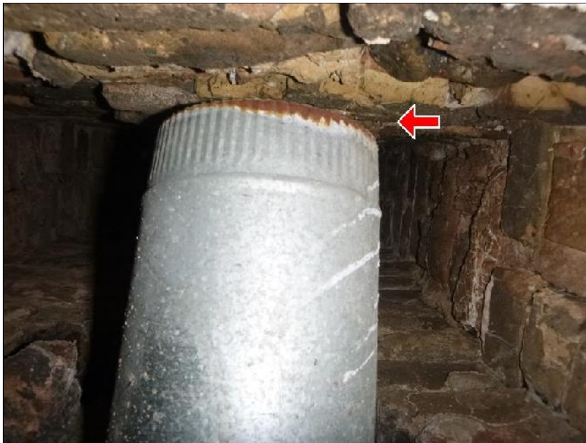
G. Item 2(Picture) dangerous gas exhaust venting
