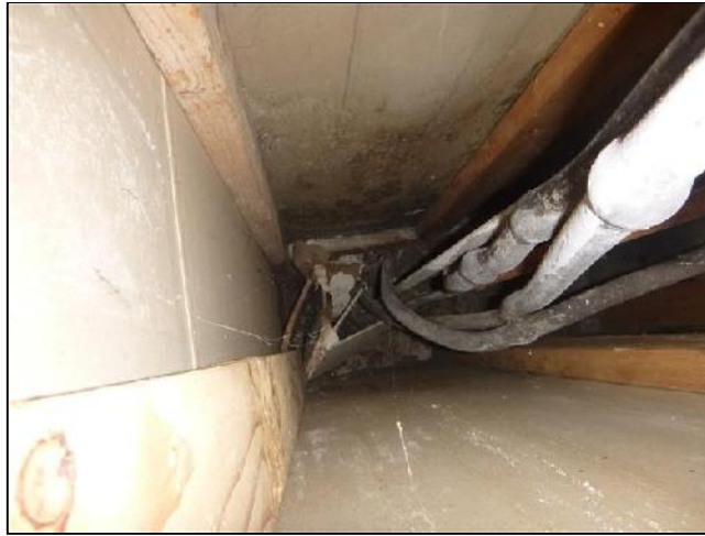
F. Item 5(Picture) lead pipe water supply piping
