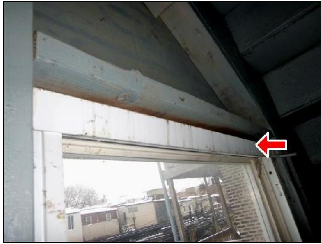
A. Item 12(Picture) evidence of ongoing water penetration
