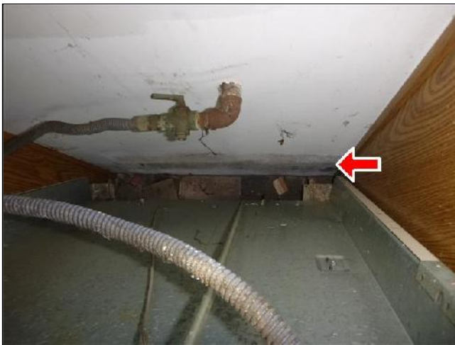
L. Item 1(Picture) missing safety bracket
