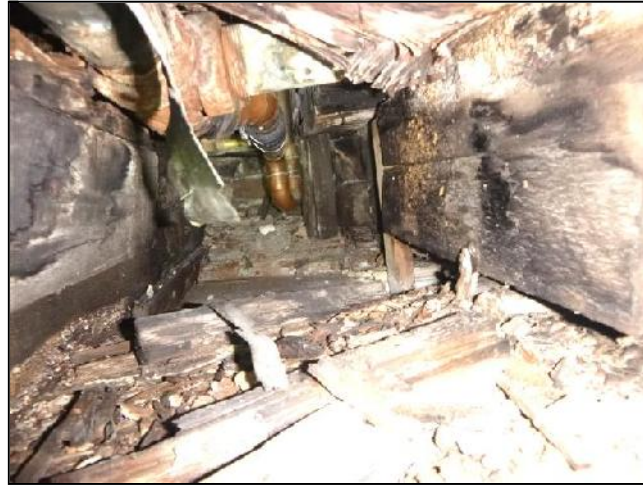
M. Item 3(Picture) deterioration within basement ceiling joist channels
