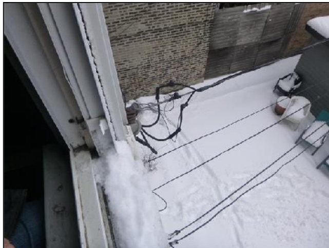
E. Item 3(Picture) inadequate safety clearance
