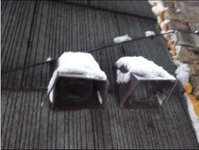
H. Item 1(Picture) dryer vent terminations
