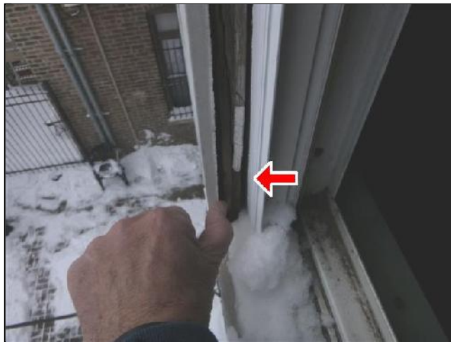
A. Item 13(Picture) ongoing moisture penetration and rot at enclosed rear porch walls
