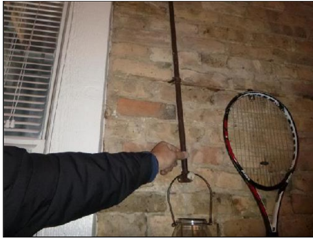
G. Item 7(Picture) antiquated gas piping
