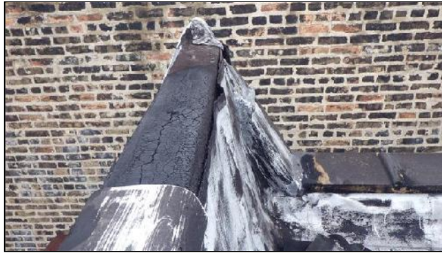
C. Item 7(Picture) failed/displaced area of modified bitumen roof covering
