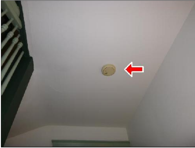
M. Item 5(Picture) Antiquated Detector
