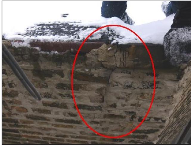
A. Item 3(Picture) masonry wall cracking and improper patching
