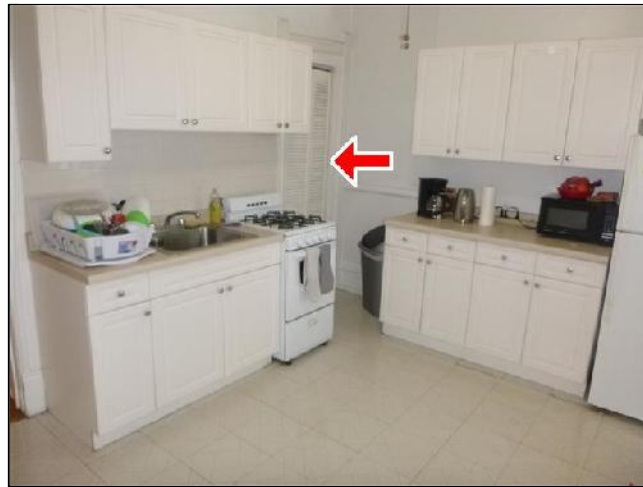
H. Item 7(Picture) No Mechanical Ventilation in Kitchen
