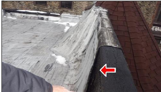
C. Item 9(Picture) missing/failed modified bitumen roof covering at front parapet
