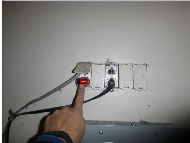
E. Item 11(Picture) defective electrical receptacle
