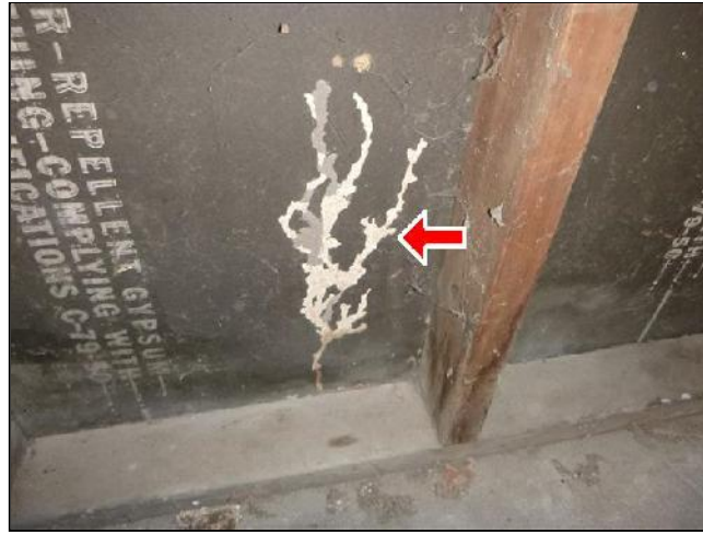
M. Item 8(Picture) Evidence of Termite Activity
