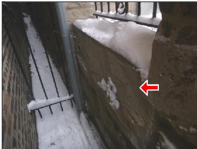
A. Item 4(Picture) failing cement parging
