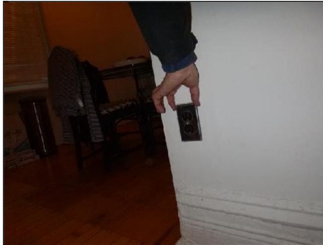
E. Item 14(Picture) Dangerously Loose Receptacle
