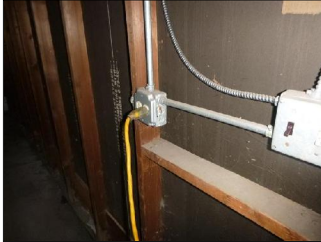
B. Item 1(Picture) Missing Shock Protection
