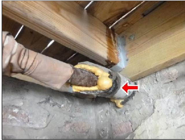
M. Item 1(Picture) possible asbestos containing building material
