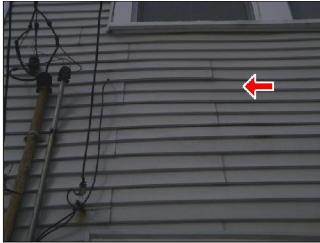
A. Item 8(Picture) buckling siding
