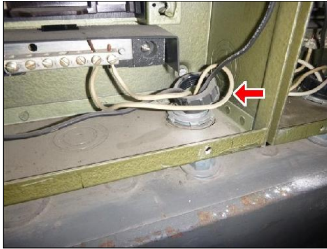
E. Item 6(Picture) defective bushing
