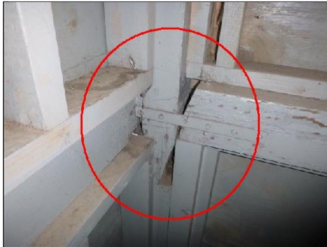
A. Item 11(Picture) suspect structural connection
