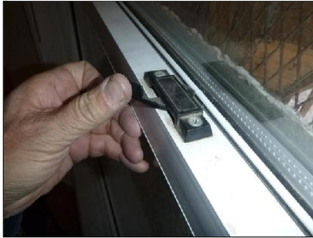
K. Item 6(Picture) Failure to Latch
