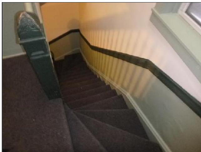
J. Item 2(Picture) missing railing
