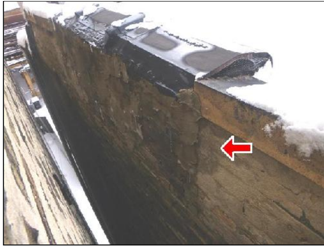
A. Item 6(Picture) failing and deteriorating parapet wall parging
