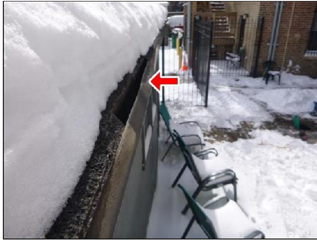
B. Item 3(Picture) Missing Drip Edge Flashing
