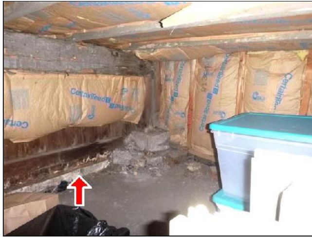
A. Item 10(Picture) moisture staining and wood rot at base of North enclosed porch exterior wall
