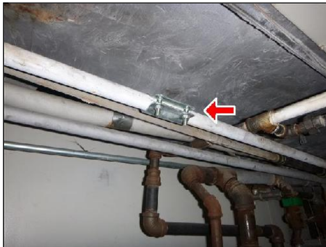
F. Item 6(Picture) galvanized water supply piping patch
