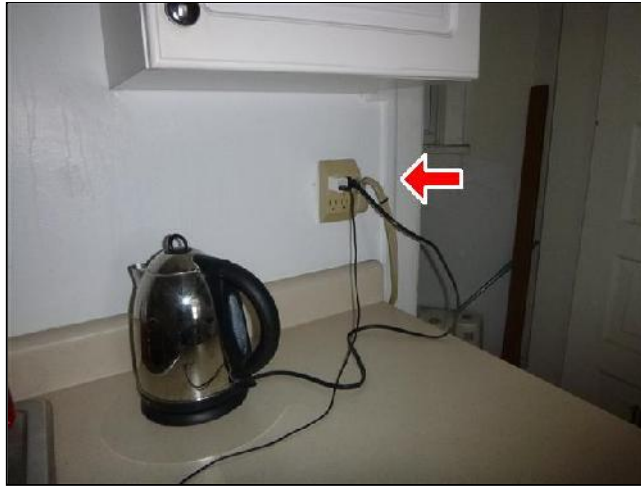
E. Item 20(Picture) missing shock protection at kitchen countertop
