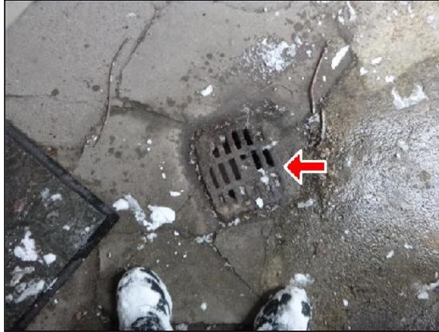
F. Item 1(Picture) blocked drain
