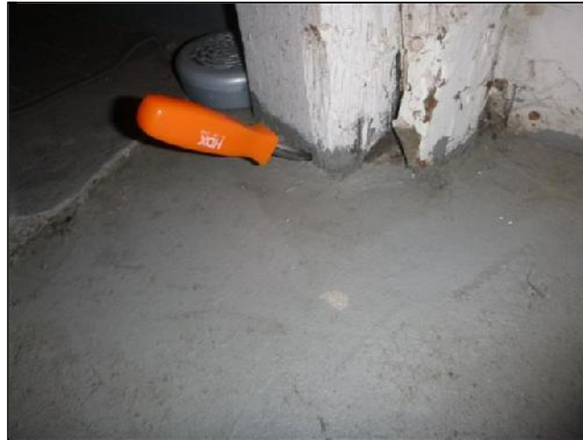
D. Item 2(Picture) deterioration at base of 6 x 6 support posts
