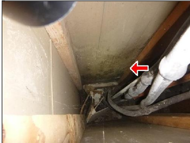
M. Item 2(Picture) moldy drywall
