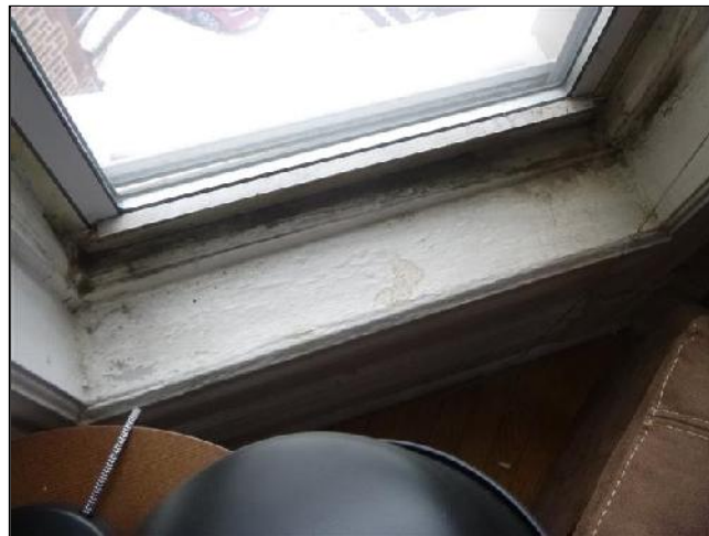
M. Item 4(Picture) Deteriorated Painted Surfaces
