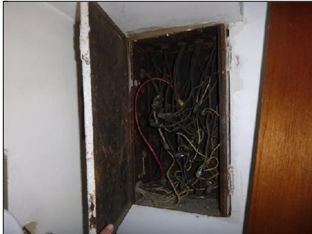
E. Item 5(Picture) extensive cloth insulated wiring
