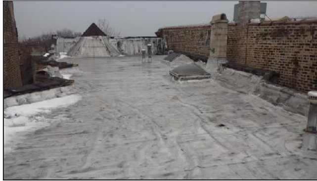
C. Item 4(Picture) widespread blistering/buckling
