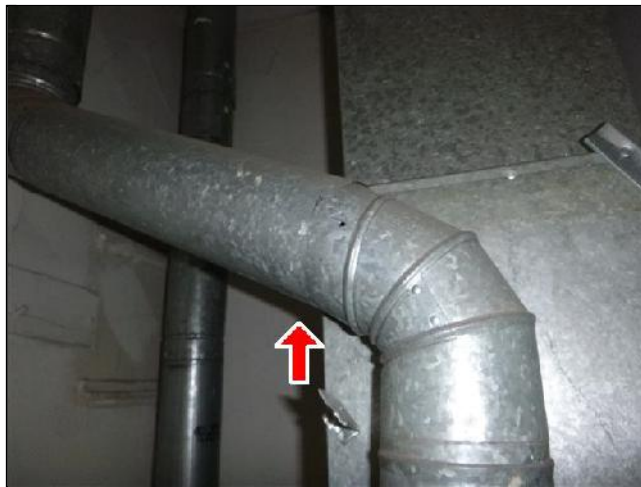
G. Item 6(Picture) unsecured piping sections
