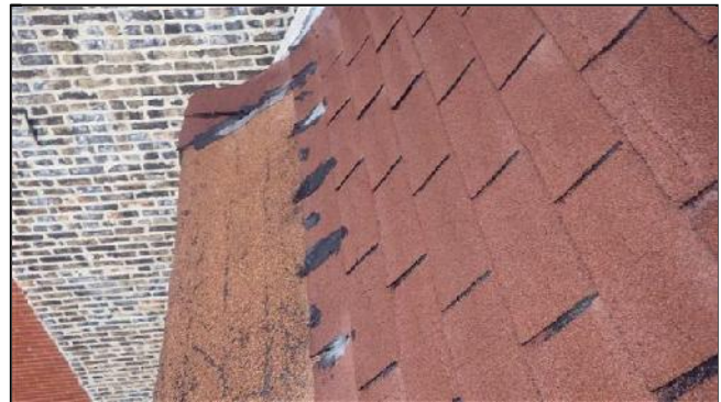
C. Item 6(Picture) badly deteriorated and heavily patched shingle roof covering
