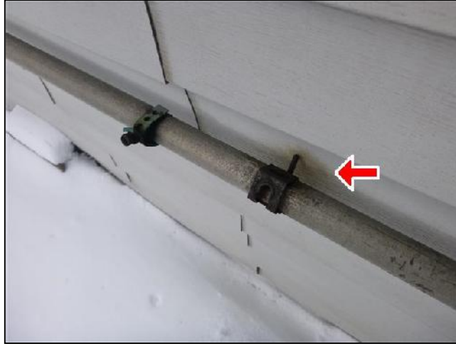
E. Item 1(Picture) in adequately secured conduit
