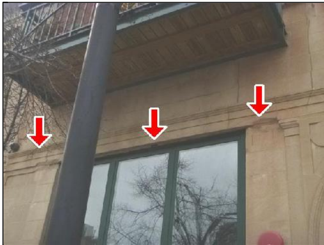
A. Item 1(Picture) Corroded Structural Steel and Resulting Masonry Damage
