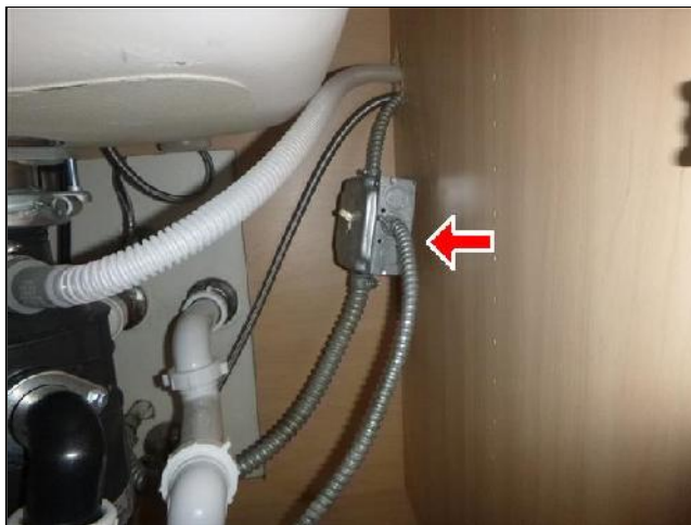
E. Item 2(Picture) Loose Electrical Equipment
