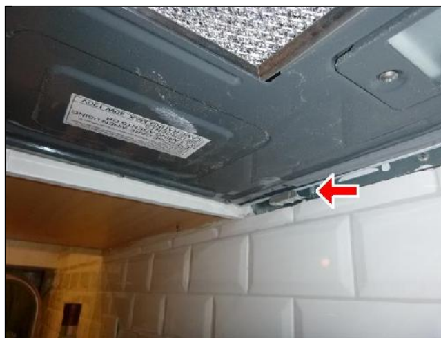
L. Item 7(Picture) Loose Microwave Oven
