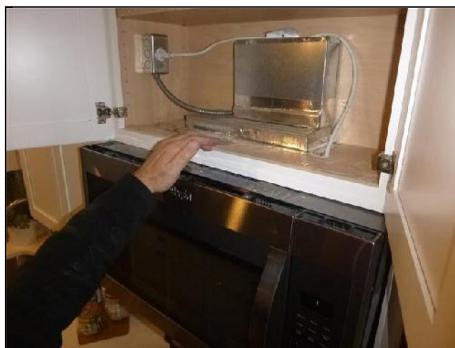
H. Item 1(Picture) Recirculating Range Hood
