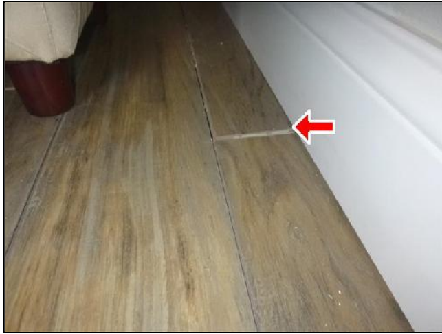
J. Item 7(Picture) Inadequately Secured Flooring
