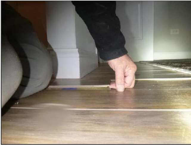
J. Item 5(Picture) Defective Tongue and Groove Installation
