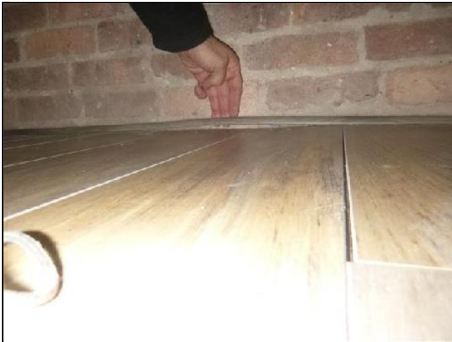
J. Item 6(Picture) Excessive Flooring Gaps and Improperly Installed Flooring Trim
