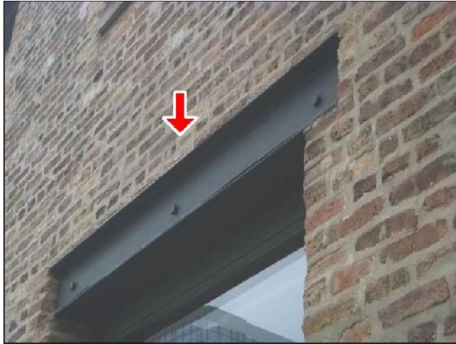
A. Item 3(Picture) No Masonry Wall Flashing Visible
