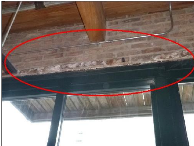
A. Item 4(Picture) Evidence of Possible Bulk Moisture Penetration Due to Missing Masonry Wall Flashing
