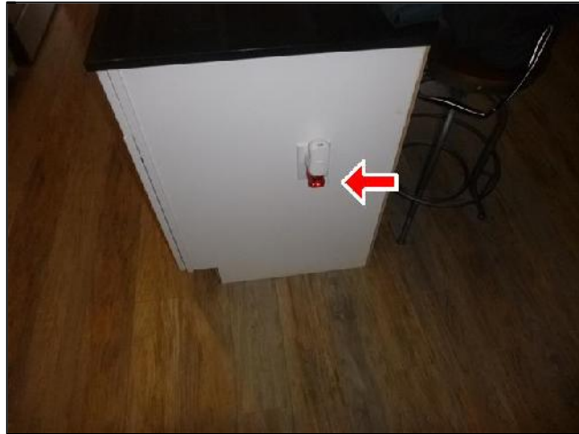
E. Item 3(Picture) Reverse Wired Receptacle
