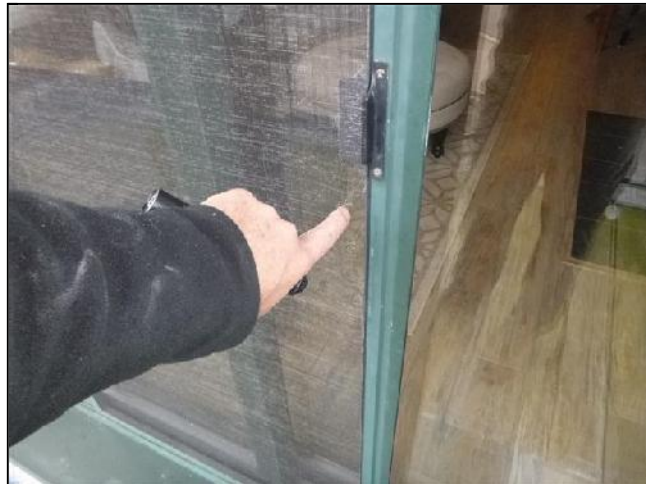
K. Item 2(Picture) Deteriorated Screening
