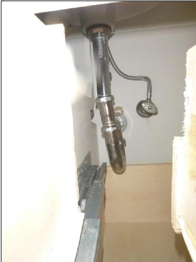
F. Item 4(Picture) Improperly Configured and Leaking Sink Drain
