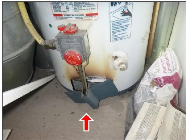
F. Item 12(Picture) Missing Drip Pan
