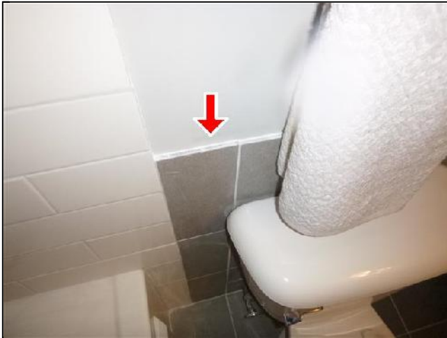
F. Item 6(Picture) Improperly Terminated Tile Edge
