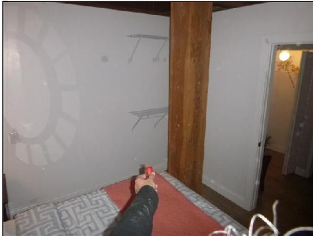
J. Item 10(Picture) Inadequate Electrical Receptacle Spacing
