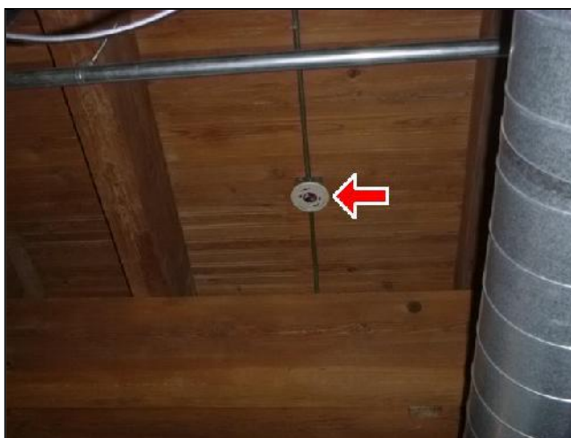
M. Item 3(Picture) Missing Detector
