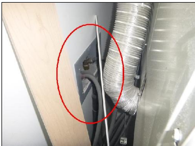
L. Item 3(Picture) Washing Machine Water Supply Hoses
