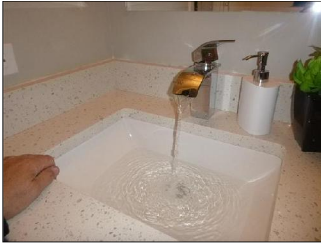
F. Item 8(Picture) Inadequate Water Flow And Loose Faucet
