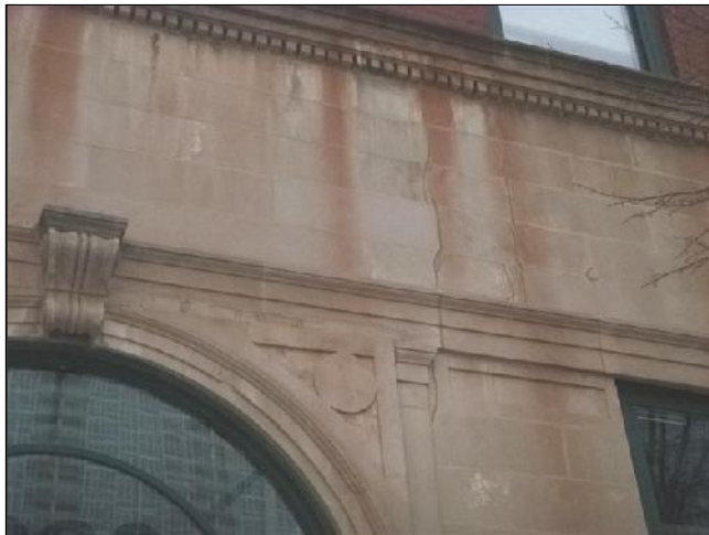
A. Item 2(Picture) Network of Patch Cracks in Exterior Stone
