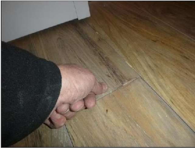
J. Item 3(Picture) Excess "Give" At Individual Pieces of MDF Flooring
