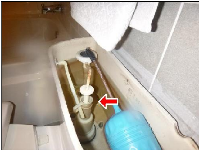
F. Item 7(Picture) Improperly Adjusted Toilet Tank Water Level
