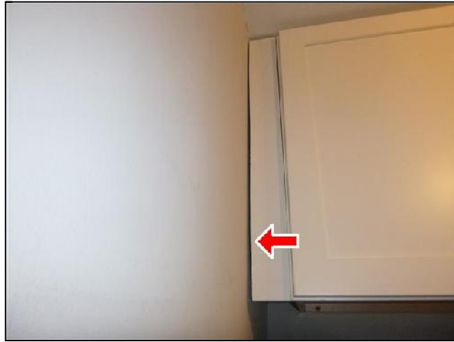
J. Item 14(Picture) Poorly Fitted Trim Piece
