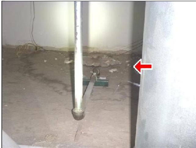
F. Item 14(Picture) Evidence of Dripping onto Area below Cast-Iron Drain Elbow
