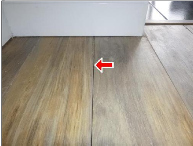
J. Item 8(Picture) Excessive Flooring Gap
