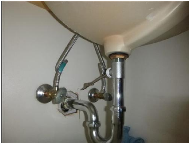
F. Item 9(Picture) Disconnected Drain Stopper
