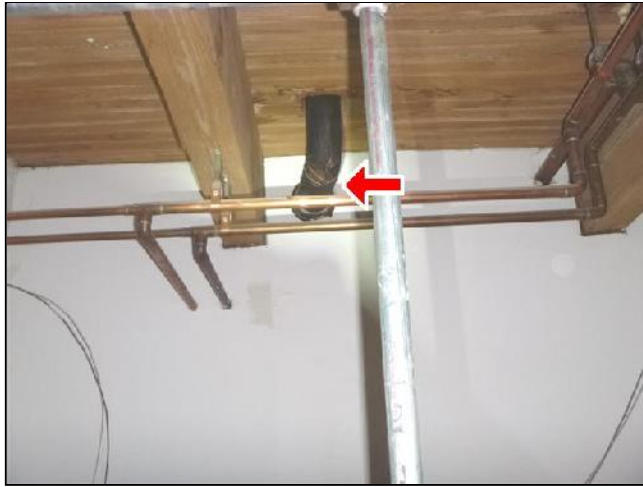
F. Item 13(Picture) Moisture Staining at Base of Cast-Iron Drain Elbow
