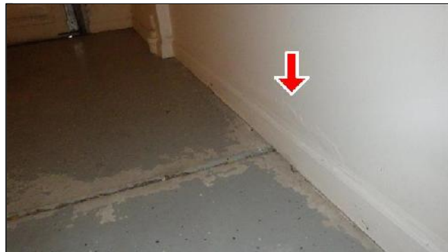
B. Item 5(Picture) Moisture Damaged Wallboard
