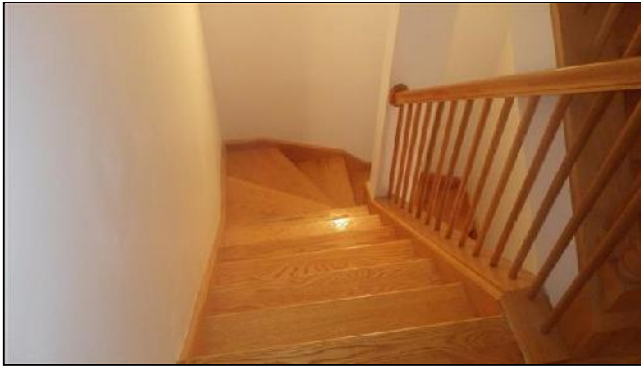
J. Item 4(Picture) Partial Handrail
