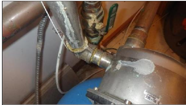
F. Item 3(Picture) Incipient Leaking
