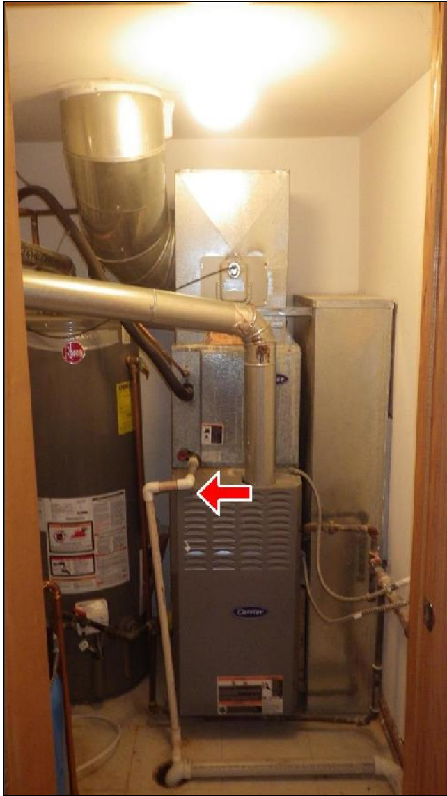
G. Item 2(Picture) Condensate Drain
