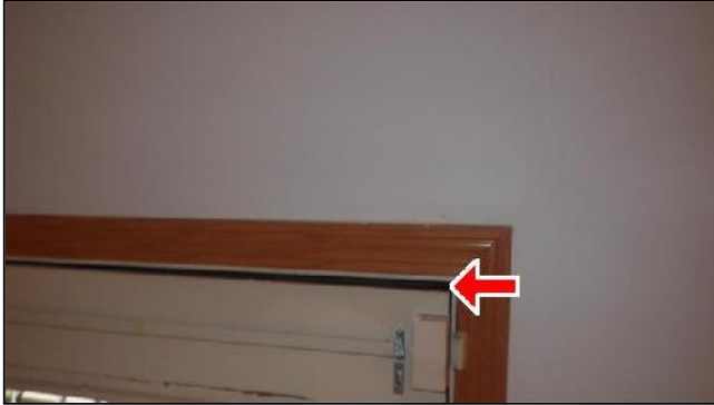
K. Item 2(Picture) Poorly Fitted Door
