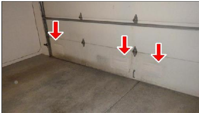
B. Item 2(Picture) Sealed Ventilation Openings
