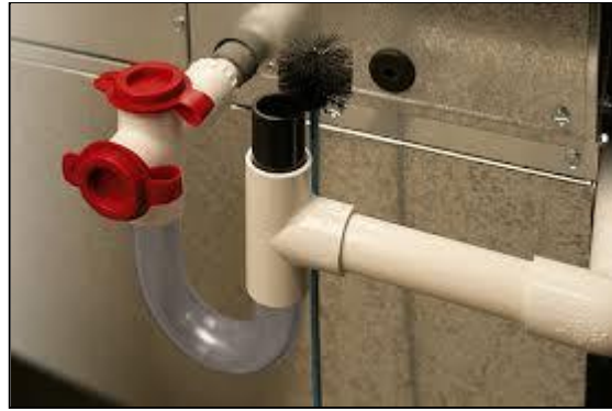
G. Item 3(Picture) Air Conditioning Condensate Drain Piping Trap
