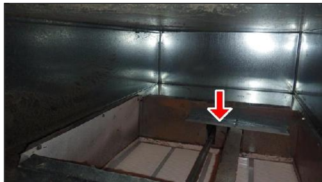
G. Item 6(Picture) Openings within the Return Air Plenum
