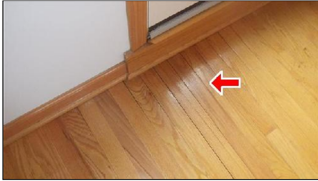
A. Item 8(Picture) Moisture Related Hardwood Flooring Damage
