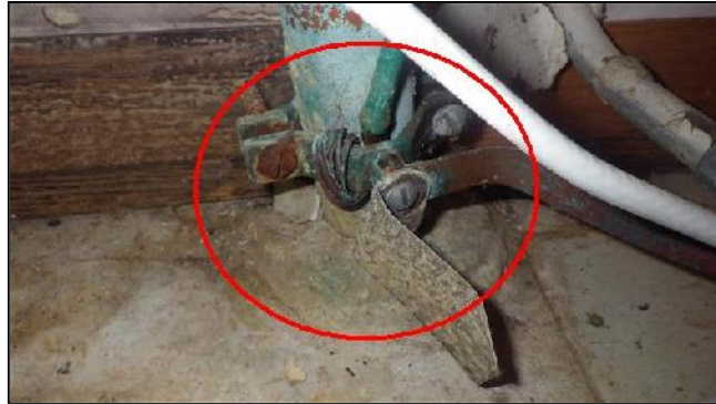
E. Item 3(Picture) Improper Grounding Connection
