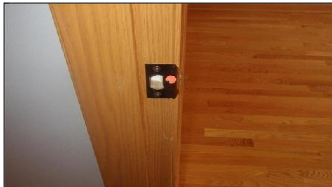
K. Item 6(Picture) Failure to Latch
