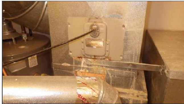
G. Item 1(Picture) Furnace Mounted Humidifier
