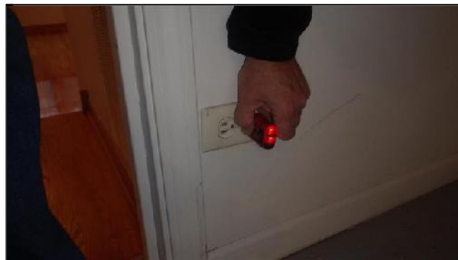
B. Item 6(Picture) Missing Shock Protection
