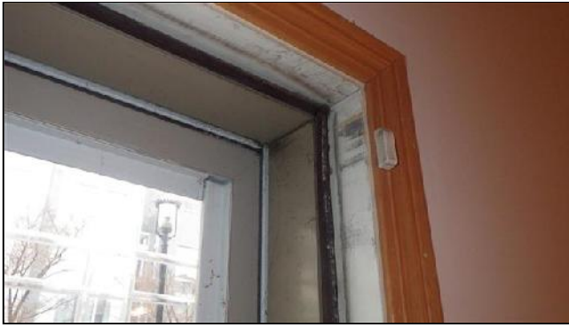
K. Item 1(Picture) Inadequate Clearance And Dust Accumulation from Continued Drafts
