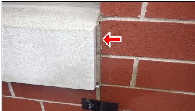
A. Item 13(Picture) Missing Caulking
