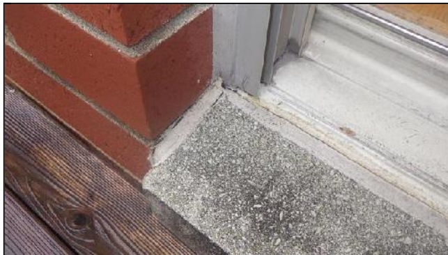
A. Item 12(Picture) Deteriorated Caulking
