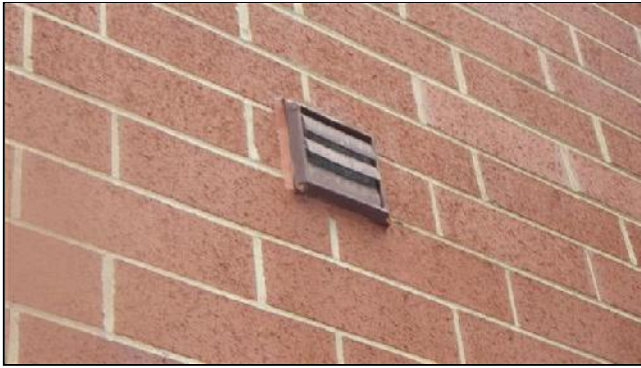
H. Item 1(Picture) Low Performance Vent Termination
