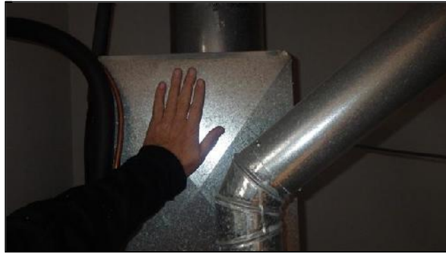
G. Item 10(Picture) Elevated Temperature
