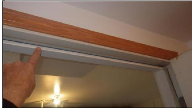
B. Item 7(Picture) Missing Weatherstripping at Garage Personnel Door
