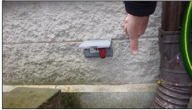
E. Item 2(Picture) Defective Receptacle
