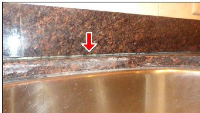
J. Item 12(Picture) Gap Between Backsplash and Countertop
