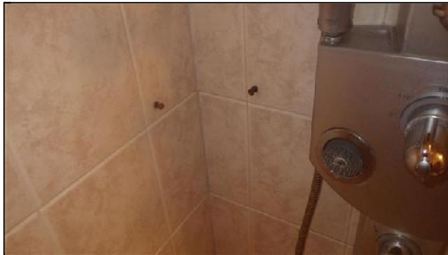
J. Item 8(Picture) Corroded and Abandoned Fasteners
