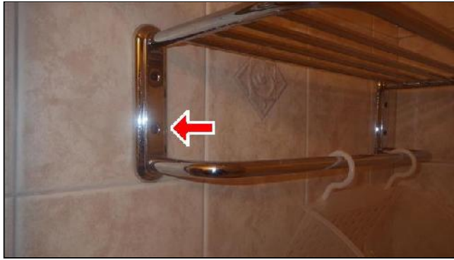
J. Item 7(Picture) Corroded Fasteners
