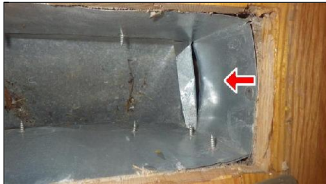
G. Item 12(Picture) Duct Leakage
