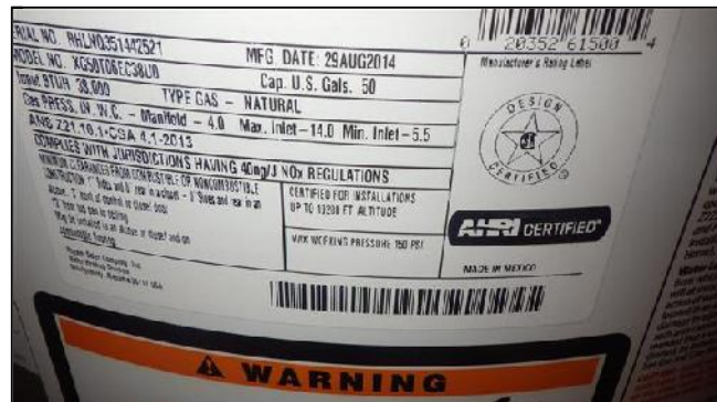
G. Item 4(Picture) Undersized Water Heater
