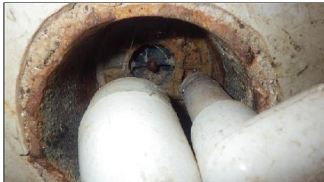
F. Item 4(Picture) Floor Drain Backup Prevention Device
