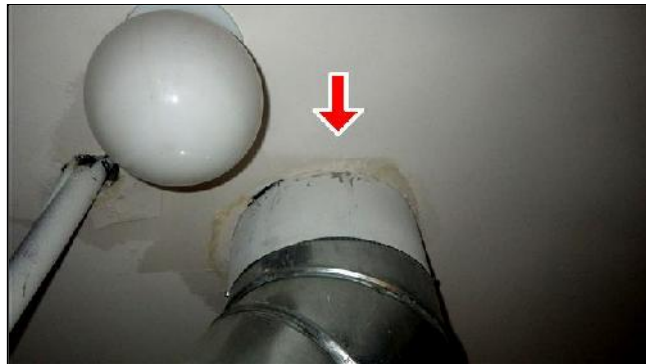
G. Item 9(Picture) Moisture Staining around Supply Ducts Penetration through Ceiling
