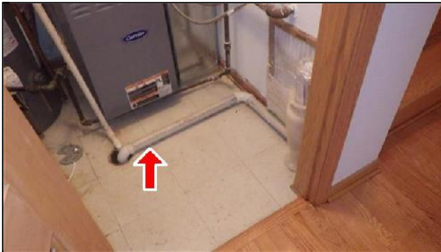
F. Item 2(Picture) Non-Conforming Sink Drain
