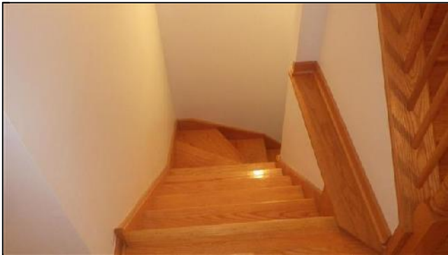
J. Item 5(Picture) Missing Railing
