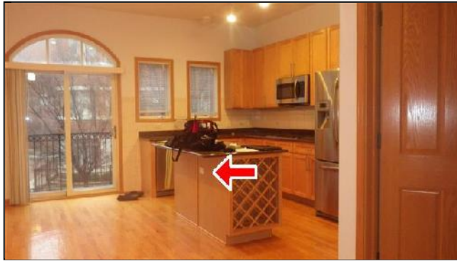
E. Item 12(Picture) Unsafe Receptacle Location
