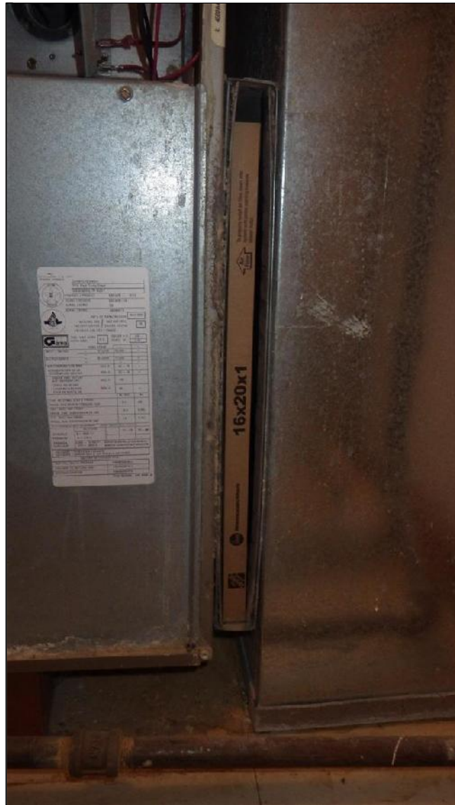
G. Item 5(Picture) Standard 1 Inch Filter
