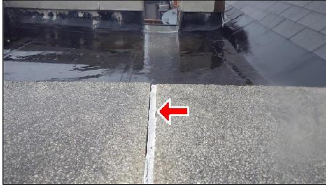
A. Item 5(Picture) Risk for Moisture Penetration and Moisture Damage
