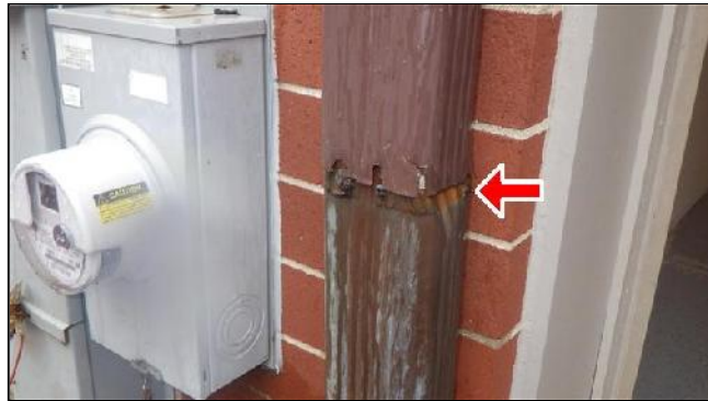
C. Item 1(Picture) Galvanic Corrosion
