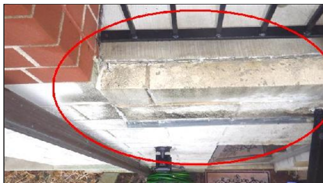
A. Item 14(Picture) Apparent Attempts to Stop Moisture Penetration
