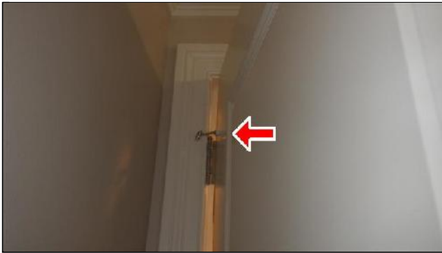
K. Item 2(Picture) Inadequate Doorstop
