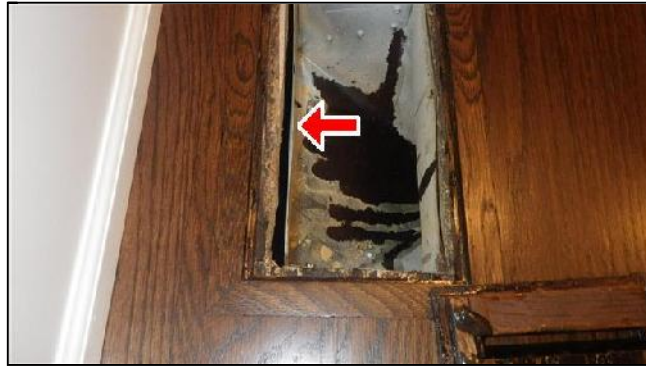
G. Item 10(Picture) Sloppy HVAC Duct Work
