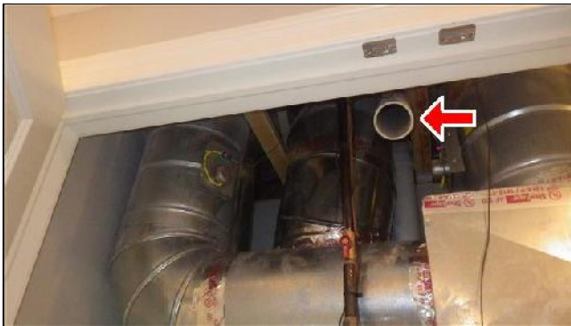
G. Item 1(Picture) Incomplete Furnace Installation
