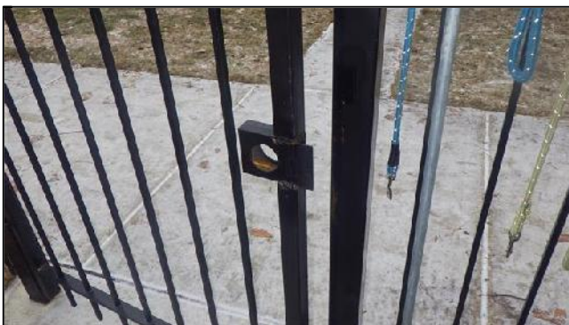
M. Item 8(Picture) Missing Hardware
