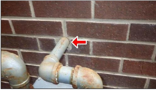
A. Item 3(Picture) Missing Caulking
