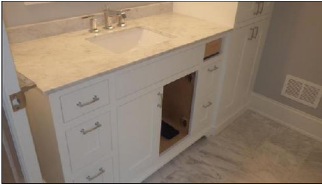
M. Item 5(Picture) Incomplete Cabinetry Installation
