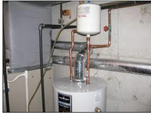
F. Item 2(Picture) Example of Expansion Tank Installation
