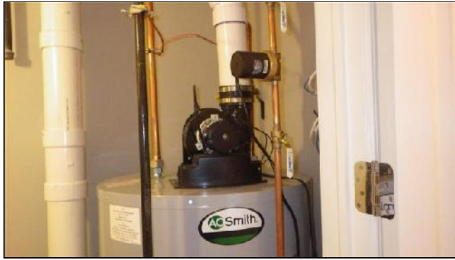
F. Item 1(Picture) Missing Expansion Tank
