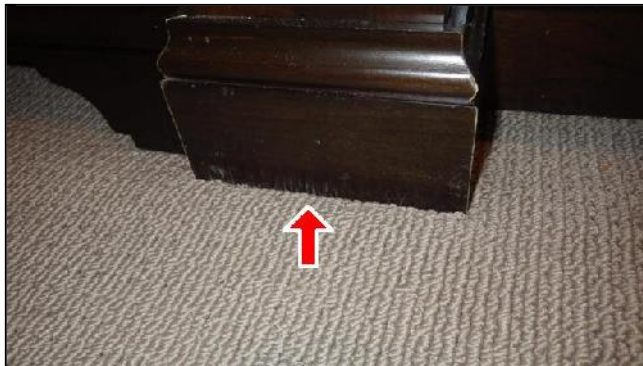
J. Item 3(Picture) Cabinetry Finish Damage
