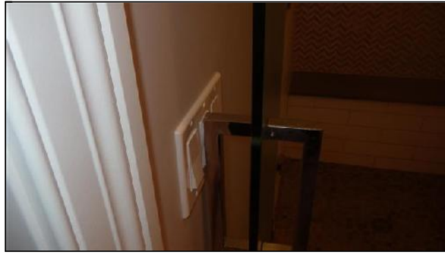
E. Item 5(Picture) Wall Switch Interference
