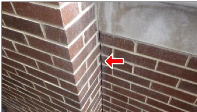
A. Item 1(Picture) Missing Caulking
