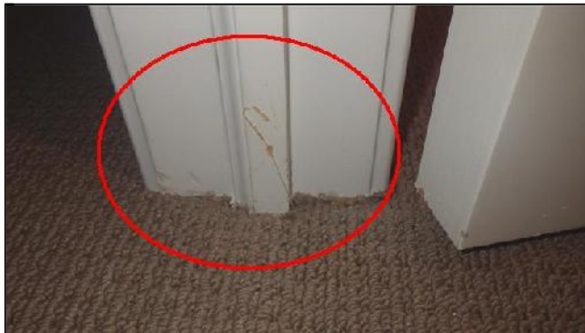
J. Item 4(Picture) Interior Trim Damage
