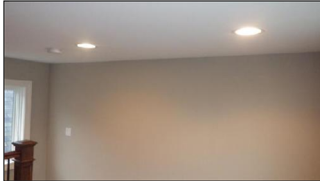
G. Item 9(Picture) Missing Return Air
