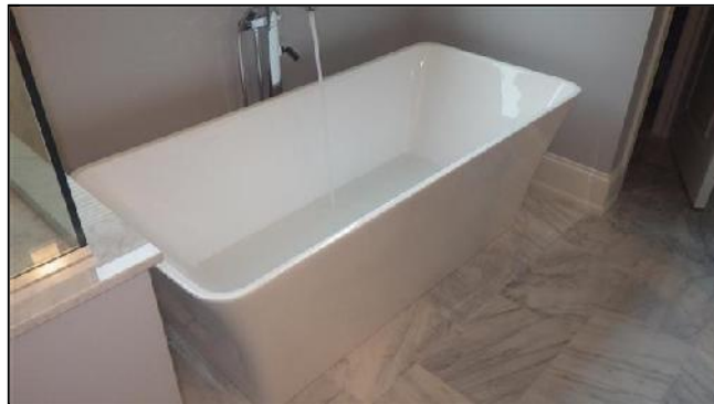
F. Item 7(Picture) Inadequately Secured Bathtub
