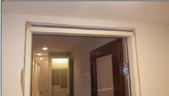
M. Item 4(Picture) Missing Interior Door Trim
