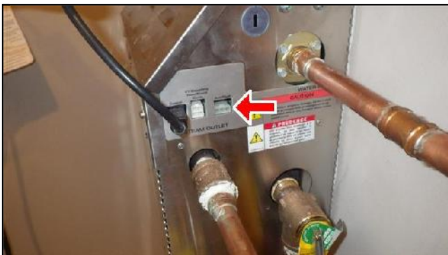
L. Item 3(Picture) Connection for Auto Flush Mechanism
