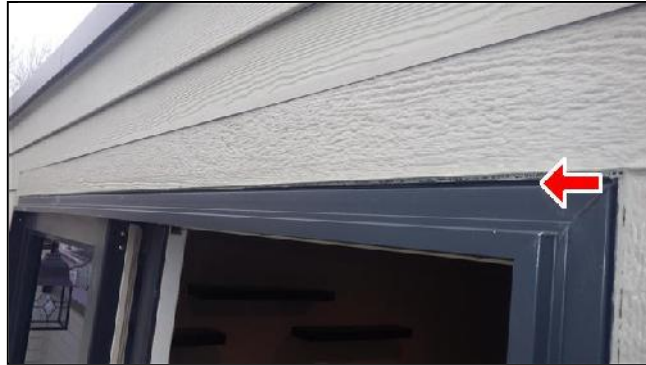
A. Item 8(Picture) Missing Flashing
