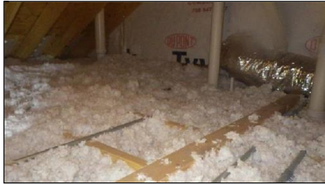
H. Item 4(Picture) Inadequate Insulation
