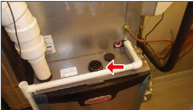
G. Item 2(Picture) Furnace Combustion Air Intake Opening
