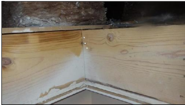
H. Item 5(Picture) Improperly Configured Attic Hatch
