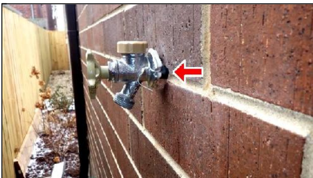
A. Item 6(Picture) Missing Caulking
