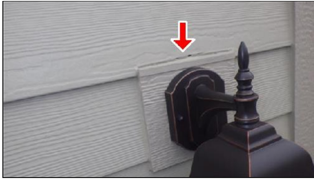
A. Item 11(Picture) Improper Siding Detail
