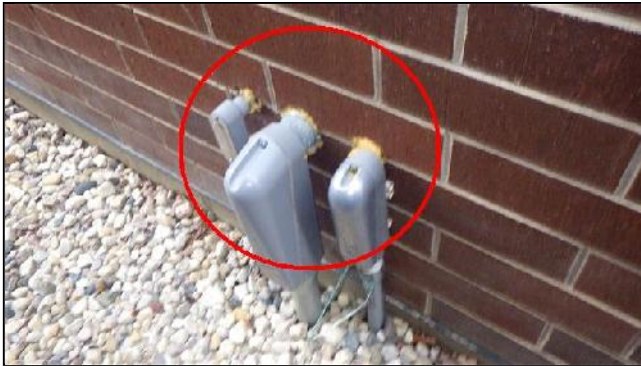
A. Item 5(Picture) Missing Caulking
