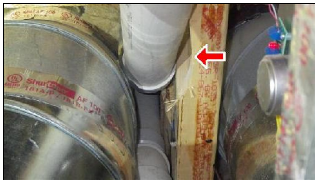
D. Item 1(Picture) Damaged Floor Truss
