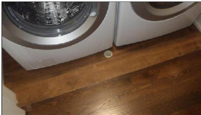
L. Item 5(Picture) Missing Drip Pan
