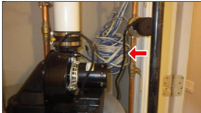
E. Item 4(Picture) Low-Voltage Wiring Should Be Organized and Secured
