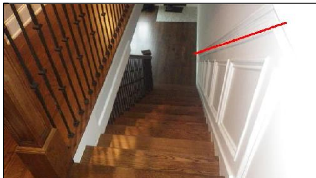
J. Item 5(Picture) Missing Railing
