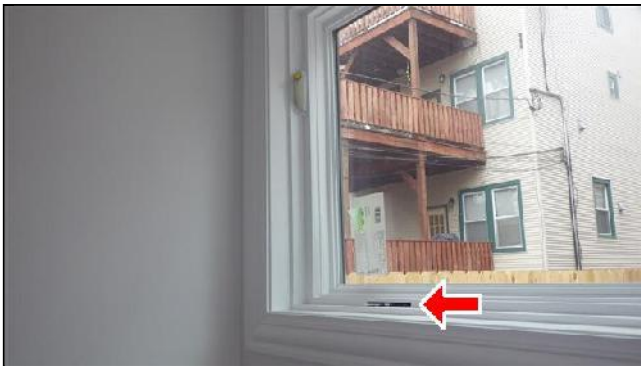
M. Item 7(Picture) Missing Window Hardware
