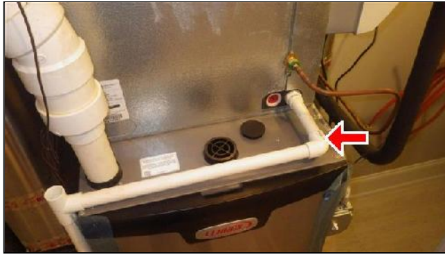
G. Item 3(Picture) Missing Condensate Drain Trap
