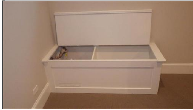
J. Item 2(Picture) Safety Hinge Recommended
