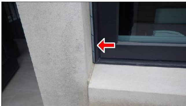
A. Item 2(Picture) Missing Caulking around Window Frame
