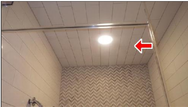
L. Item 1(Picture) Missing Slope at Ceiling
