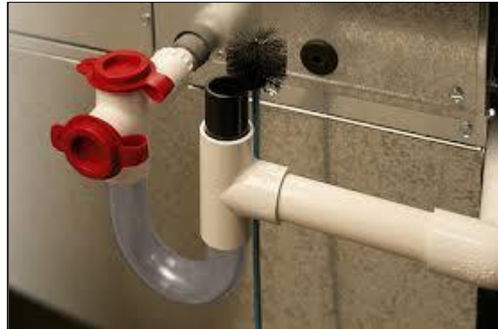
G. Item 4(Picture) Air Conditioning Condensate Drain Piping Trap
