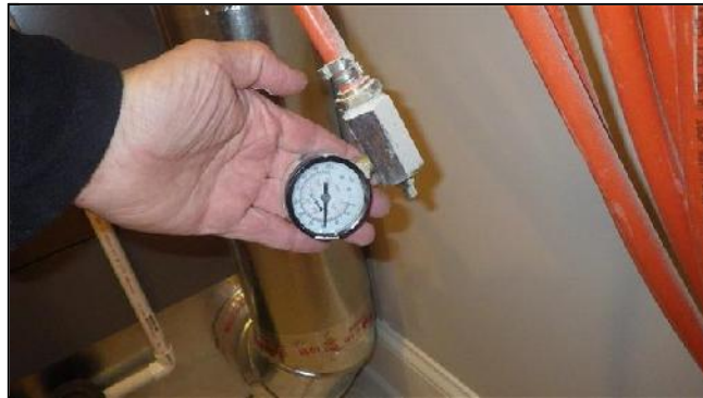
G. Item 7(Picture) Pressure Tested Hydronic Tubing System
