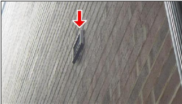
A. Item 4(Picture) Missing Caulking
