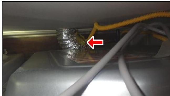
L. Item 4(Picture) Forbidden Vent Material
