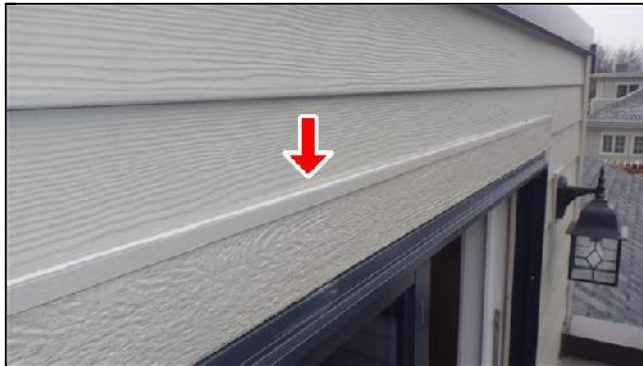
A. Item 12(Picture) Improper Siding Detail
