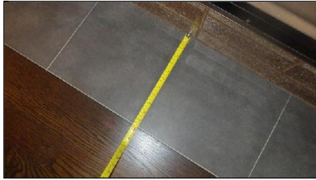
I. Item 1(Picture) Inadequate Hearth Extension Depth
