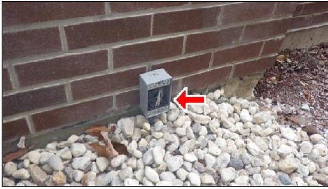
E. Item 1(Picture) Missing Junction Box Cover
