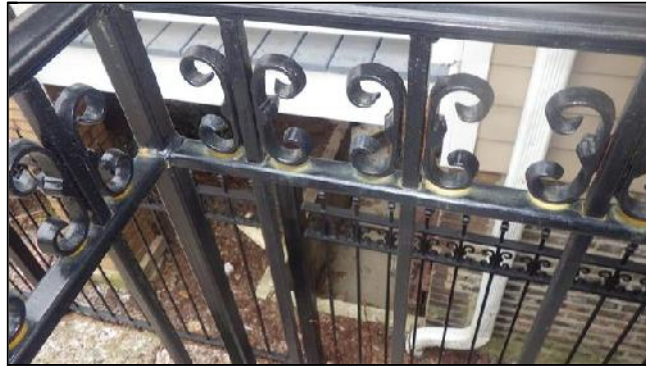
A. Item 14(Picture) Incipient Corrosion
