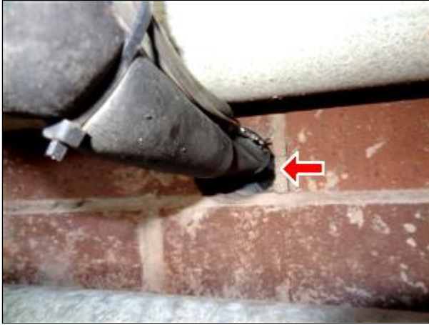
A. Picture 9 Unsealed Air-Conditioning Refrigerant Line Penetration
