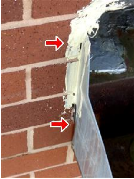
A. Picture 22 Missing and Smeared Caulk at Scupper Opening
