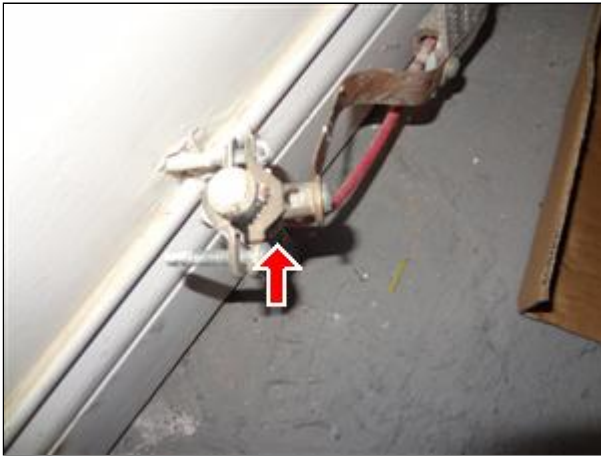
C. Picture 1 Improper Electrical Connection
