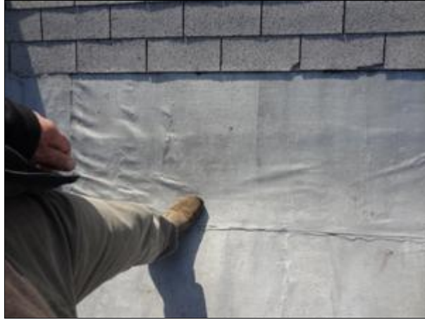
B. Picture 8 Spongy Roof Sheathing
