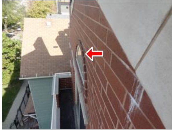
A. Picture 30 Projecting Soldier Course at Arch Top Window
