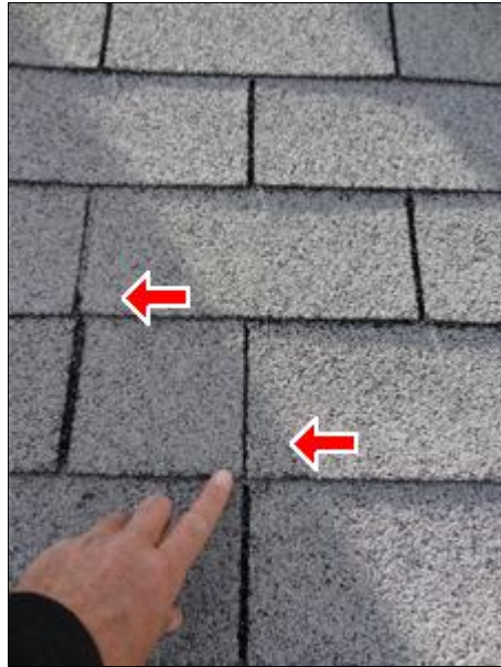
B. Picture 5 Improper Shingle Application
