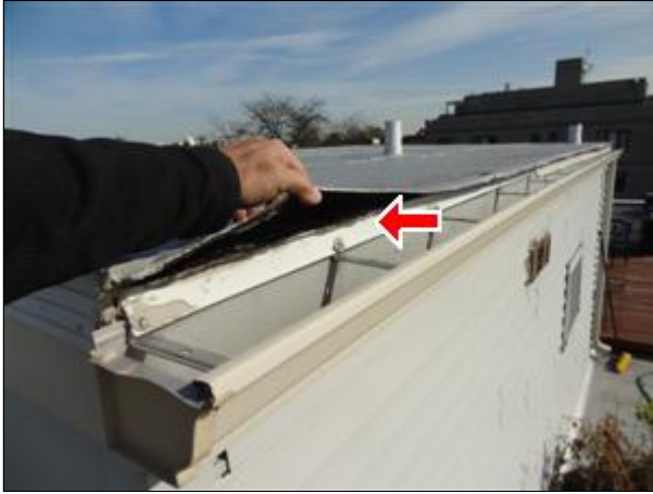
B. Picture 9 Unsealed Roof Membrane
