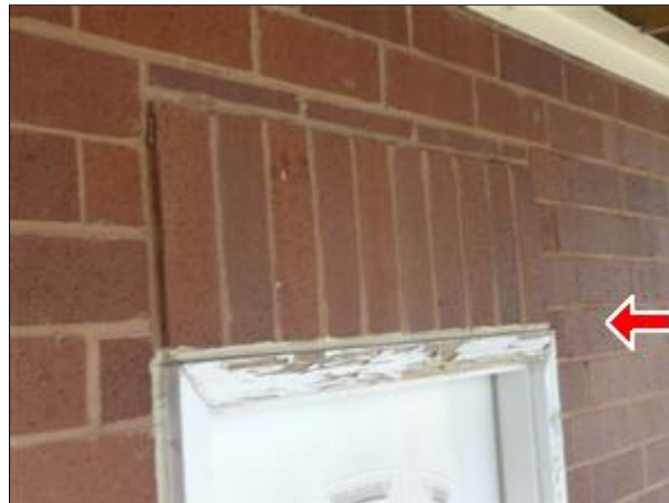
A. Picture 17 Improper Door Installation
