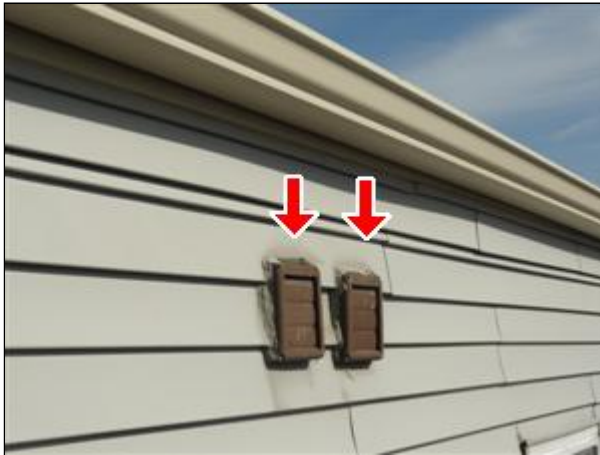
A. Picture 28 Improper Vinyl Siding Penetrations
