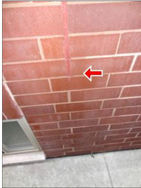
A. Picture 5 Incomplete Movement Joint
