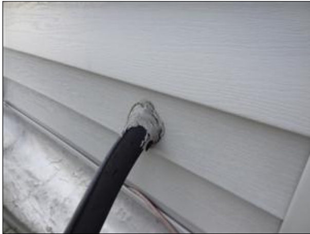
A. Picture 26 Improper Vinyl Siding Penetration
