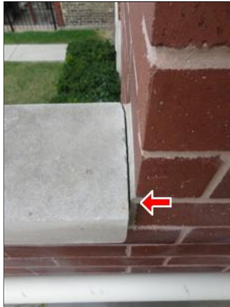
A. Picture 4 Limestone Mortar Joint
