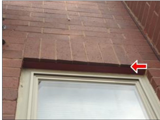
A. Picture 11 Missing Flashing
