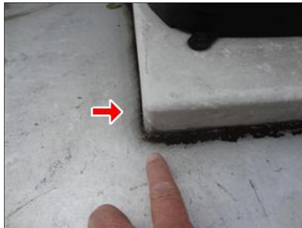
B. Picture 4 Risk for Damage to Roof Covering
