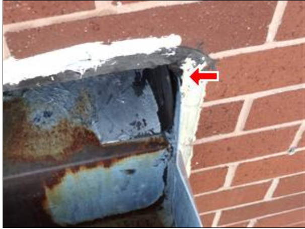
A. Picture 23 Loose Flap of Roofing Membrane At Scupper Opening
