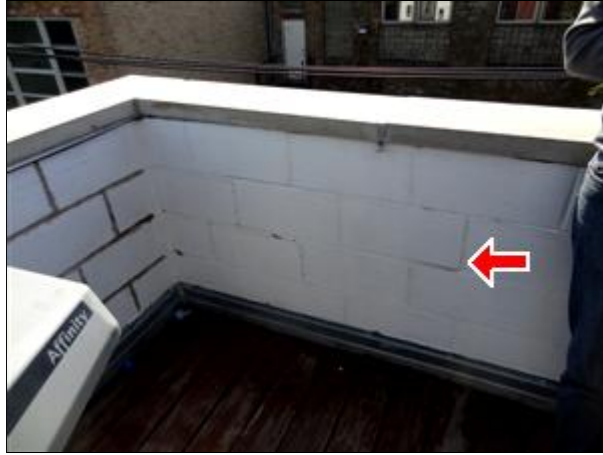
A. Picture 32 Mortar Cracking at Concrete Masonry Units Of the Inner Parapet
