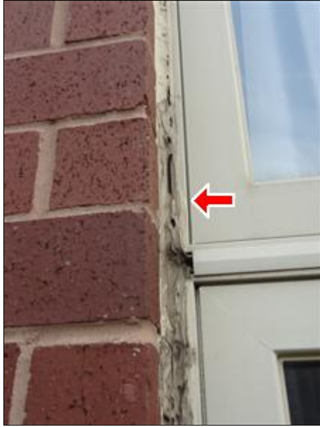
A. Picture 2 Aged and Deteriorated Caulking
