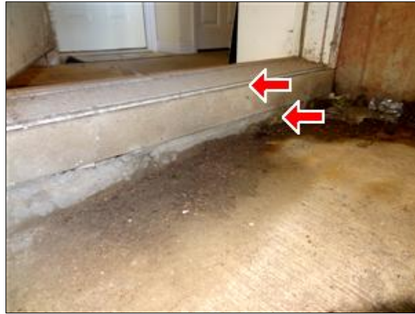
A. Picture 16 Rear Basement Entry Door
