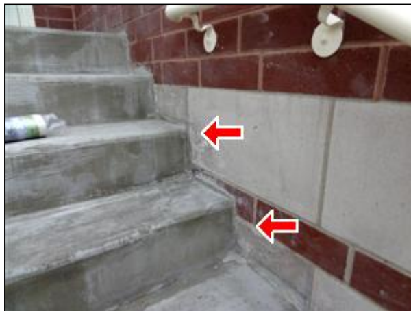
A. Picture 1 Front Exterior Stairs
