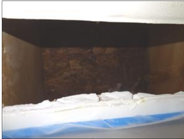
D. Picture 1 Mold-like Substances on Underside of Roof Sheathing
