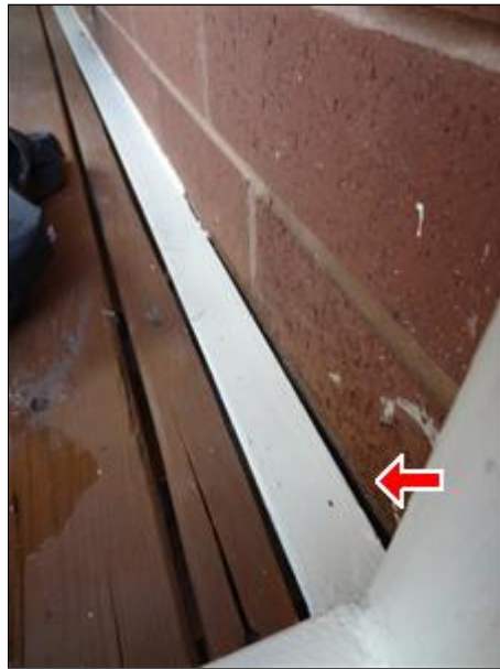
A. Picture 8 Incomplete Sealant Joint
