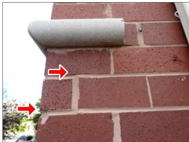
A. Picture 13 Substandard Cement Mortar
