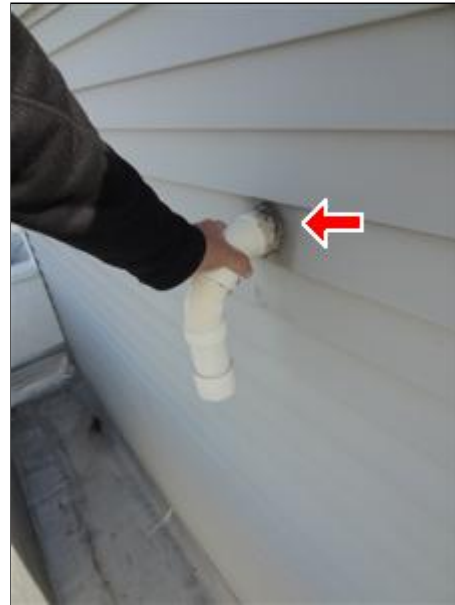
A. Picture 29 Installation of Vinyl Siding Mounting Blocks Recommended
