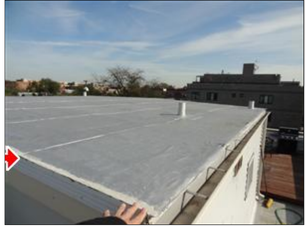
B. Picture 10 Improperly Detailed Edge Metal Flashing
