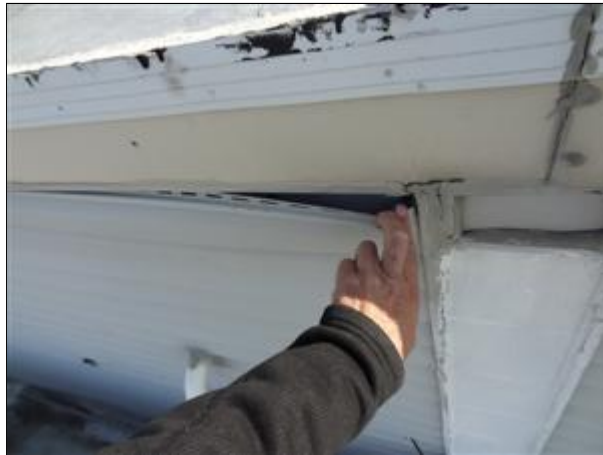
A. Picture 31 Loose Siding
