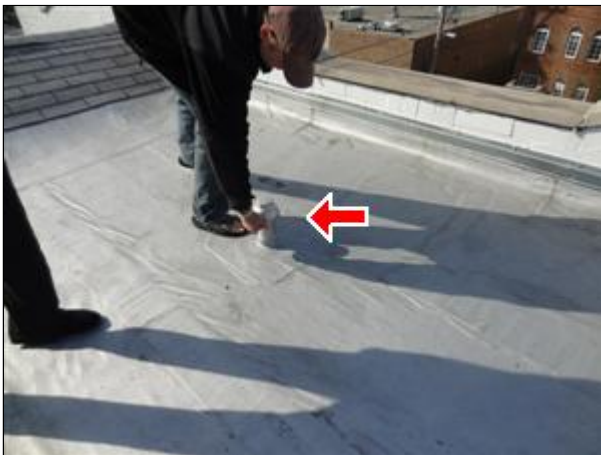
B. Picture 6 Inappropriate Installation
