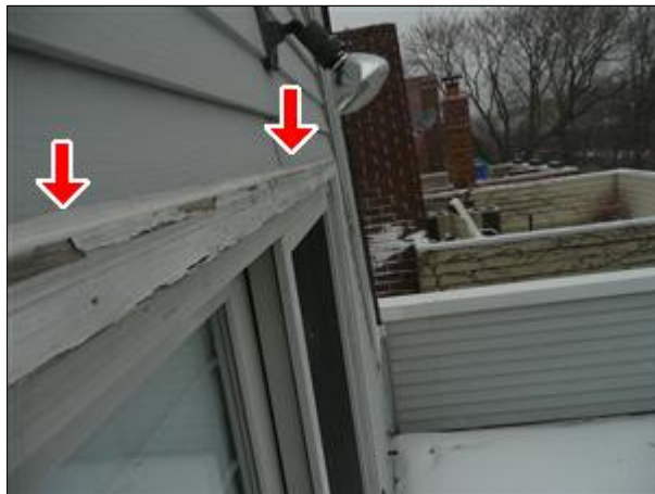
A. Picture 6 install head flashing, replace/repair aged trim
