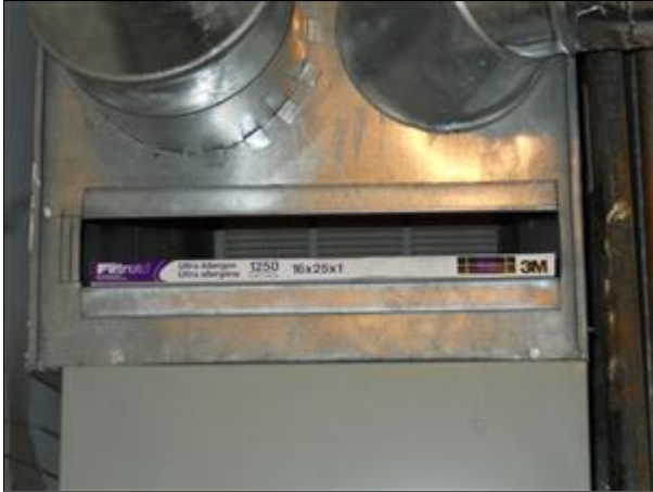
E. Picture 1 poor rack fitment
