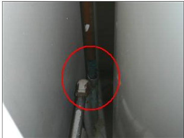
G. Picture 18 TPR piping should NOT route upward G. Picture 19 hidden TPR termination at south side of heater
