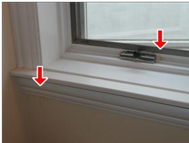
H. Picture 11 moisture staining at 2nd fl bath likely moisture control issue, not leaking
