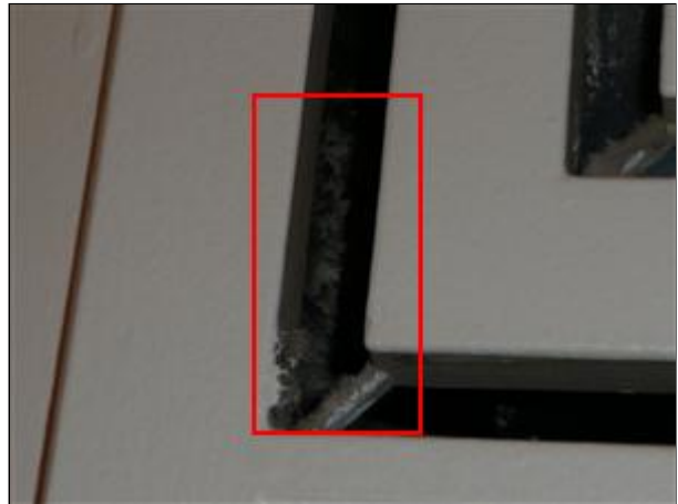
E. Picture 12 dirty fan interior, clean for increased fan performance
