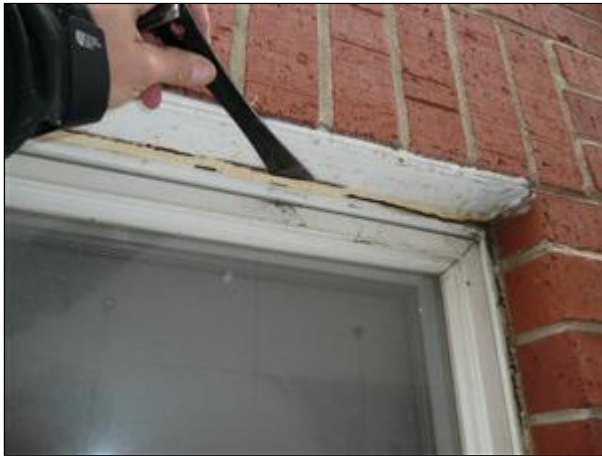
A. Picture 1 multiple, if not all windows, require sealant replacement
