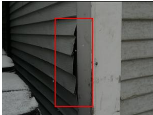
B. Picture 5 repair south siding
