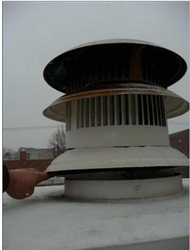
E. Picture 22 kitchen chimney prone to downdrafts but may be within acceptable installation limits
