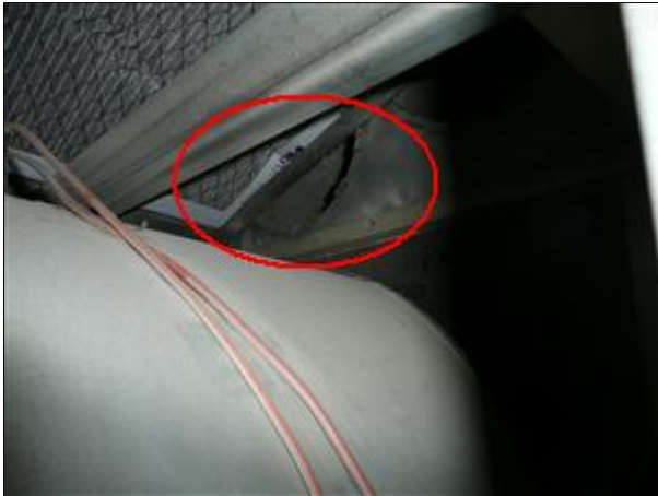
E. Picture 17 large return bypass of filter, 2nd fl furnace
