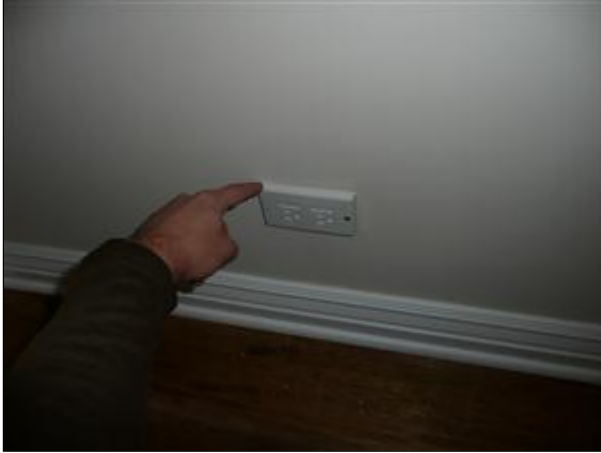
D. Picture 6 align and secure child safety covers
