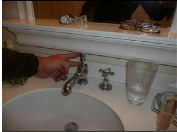
G. Picture 3 adjust 2nd fl pop up and drain assembly
