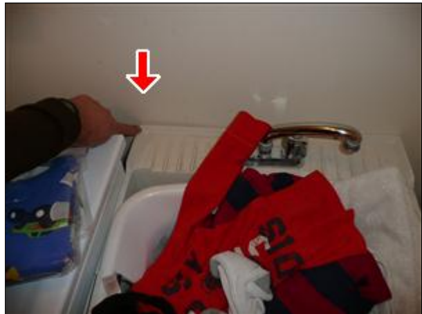
G. Picture 5 secure utility laundry sink to wall
