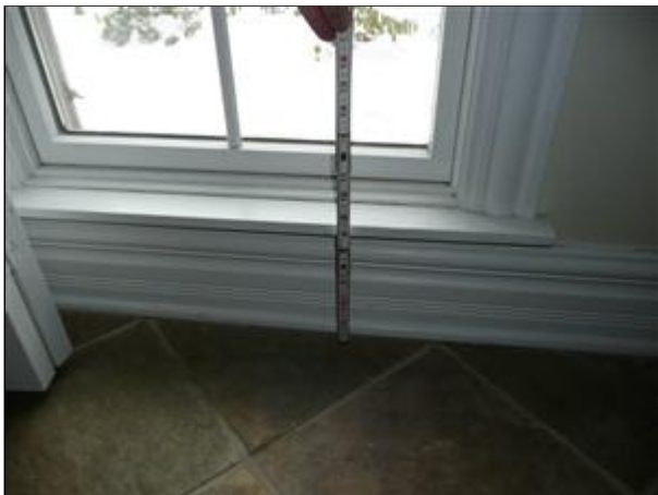
J. Picture 11 repair glass for safety purposes
