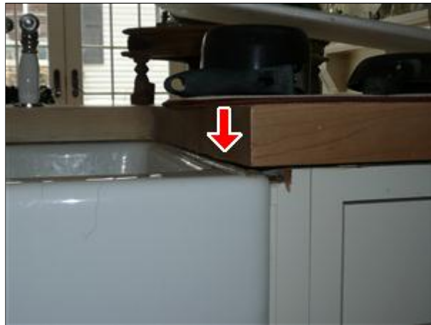
H. Picture 8 seal kitchen sink to counter gaps
