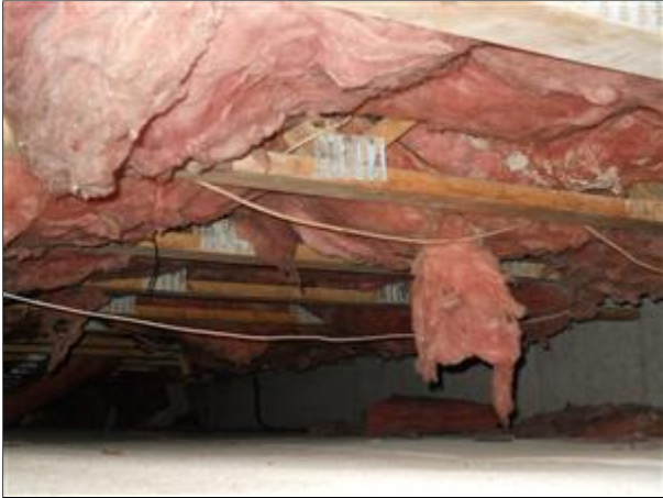
L. Picture 1 ineffective insulation
