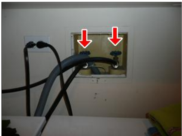
I. Picture 2 upgrade hoses
