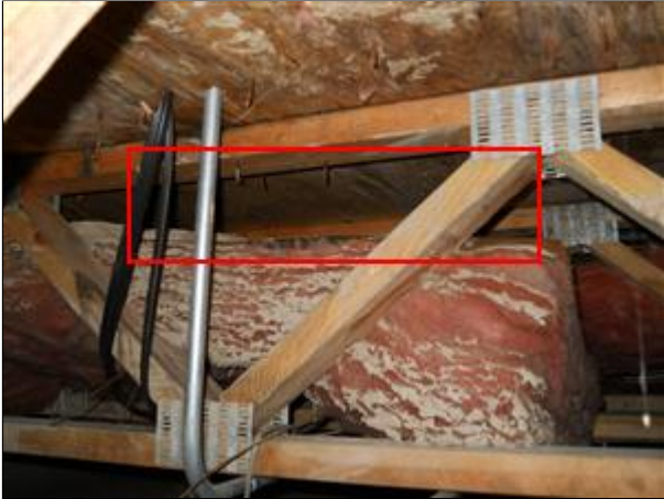
L. Picture 2 large gaps, no insulation contact
