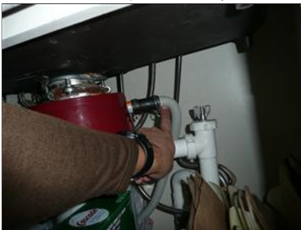
I. Picture 6 install DW drain in high loop
