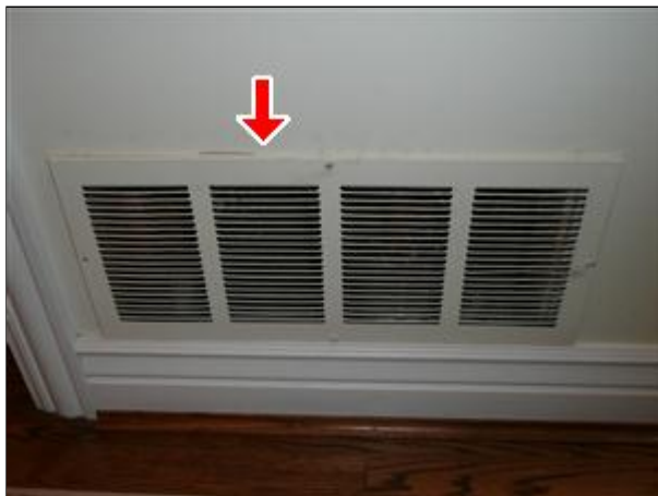
E. Picture 23 central hallway, 1st fl
