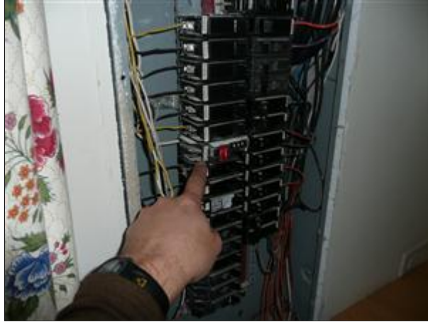
D. Picture 11 breaker in OFF position
