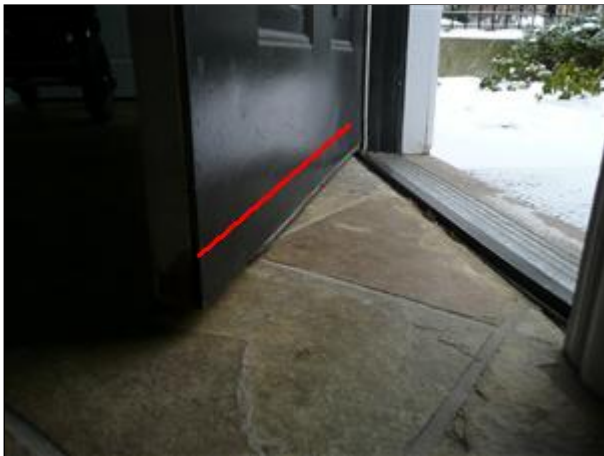
J. Picture 4 front entry door, install drip cap
