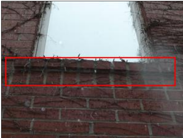
A. Picture 9 no flashing evidence below sills
