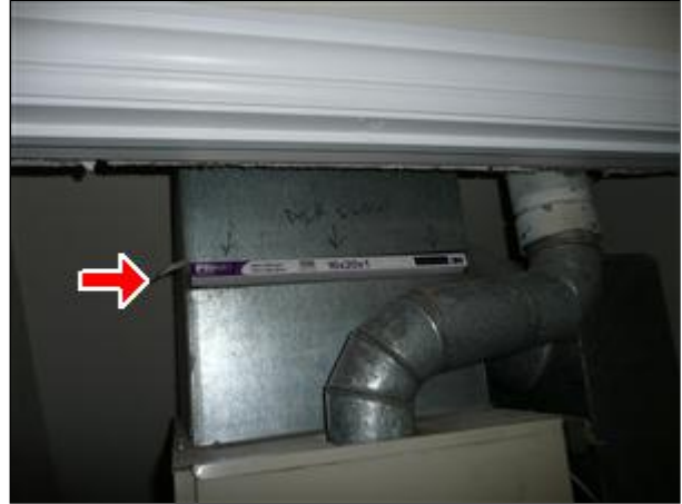
E. Picture 2 install filter cover for 2nd fl furnace
