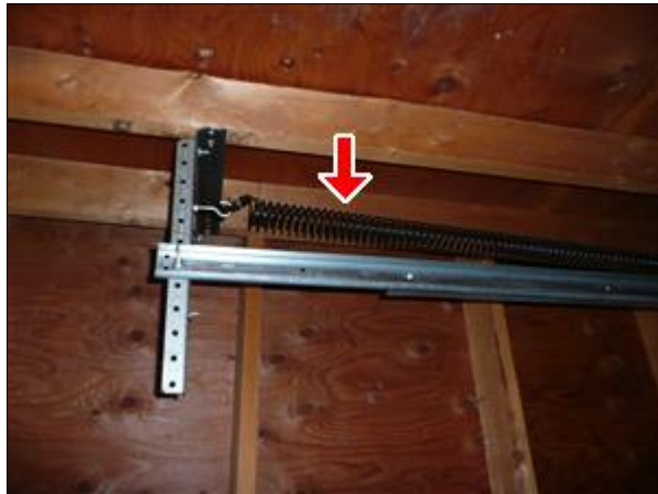
B. Picture 9 missing containment cables
