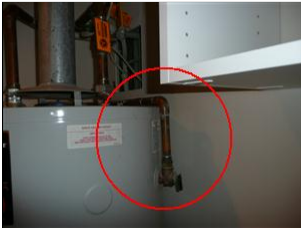
G. Picture 18 TPR piping should NOT route upward G. Picture 19 hidden TPR termination at south side of heater
