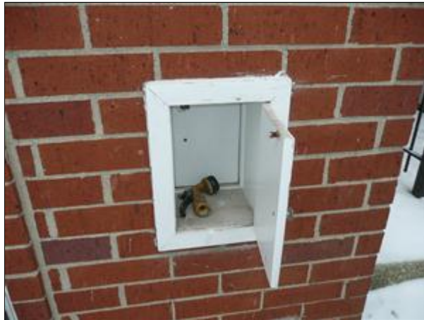
G. Picture 21 insulate access box with rigid foam
