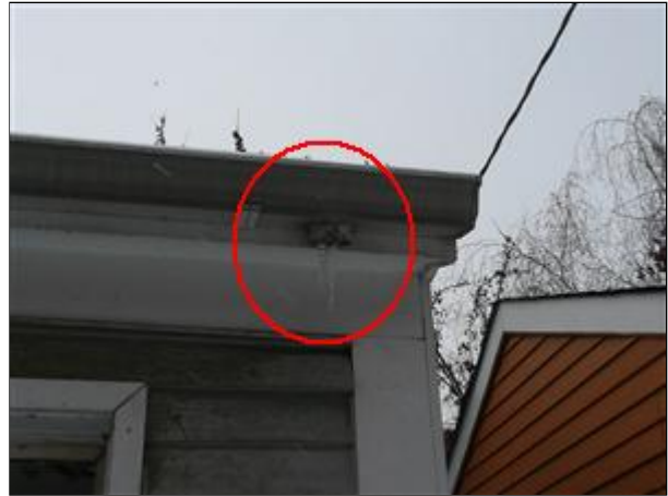
B. Picture 8 missing east downspout(s)
