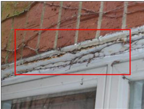
A. Picture 11 rusting lintel, north kitchen window
