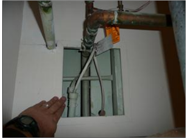
E. Picture 10 seal opening in HWH closet
