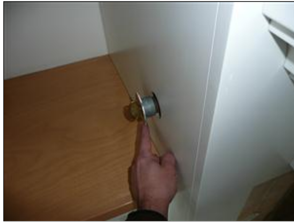
G. Picture 10 repair kitchen fireplace gas escutcheon
