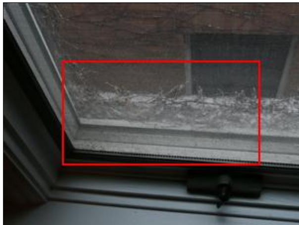
J. Picture 7 ivy growth prevented safe operation, trim or remove
