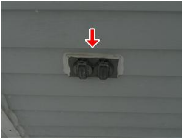
D. Picture 1 upgrade aged exterior outlets
