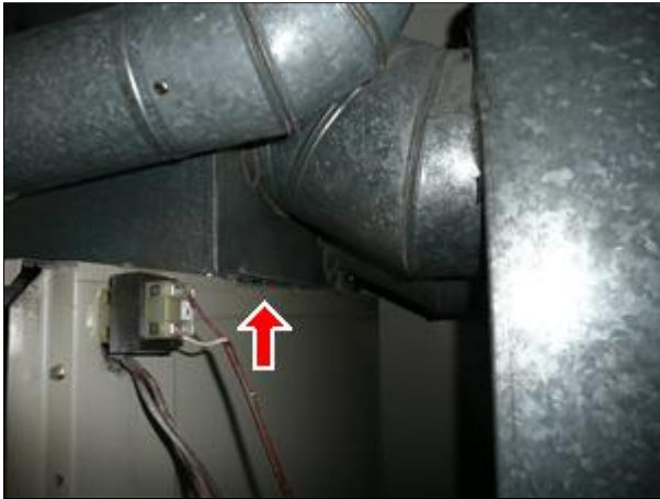
E. Picture 3 large plenum gap @ 2nd fl furnace
