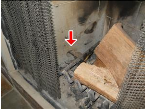
F. Picture 1 seal all log lighter openings
