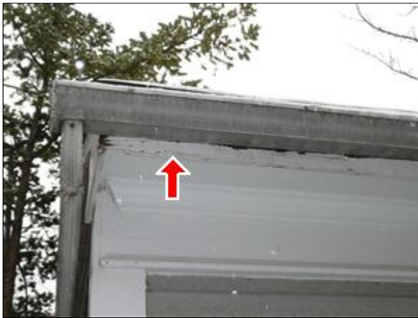
B. Picture 3 aged alley side fascia board
