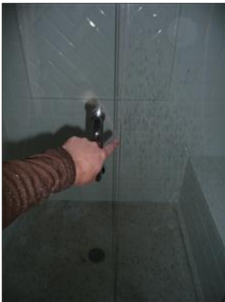
H. Picture 3 install astragal gasket at 2nd fl shower
