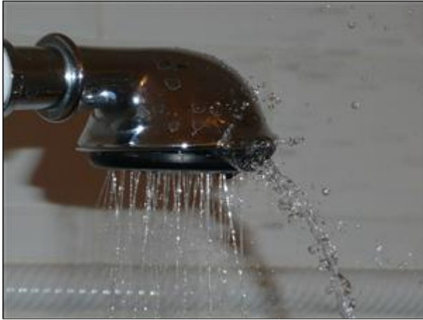
G. Picture 2 leaking 2nd fl showerhead
