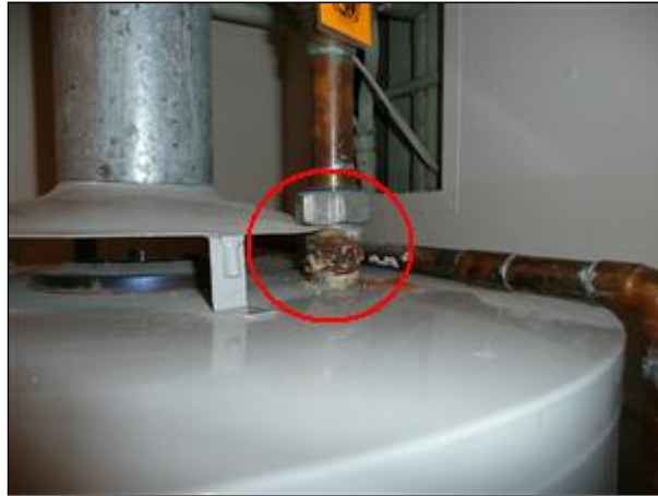
G. Picture 17 corroded union; may also be larger indication of poor draft due to lack of combustion air
