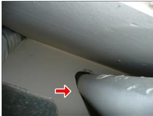
E. Picture 14 B vent clearance needs 1" airspace from combustibles
