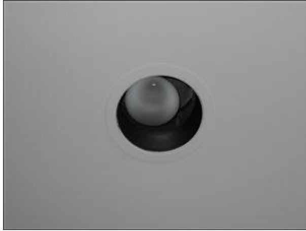
D. Picture 4 recommend air tight inserts
