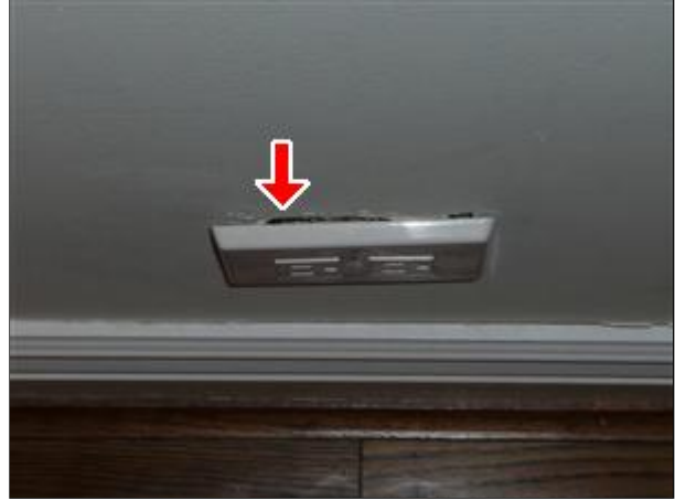
D. Picture 7 hallway outlet outside childrens' bath
