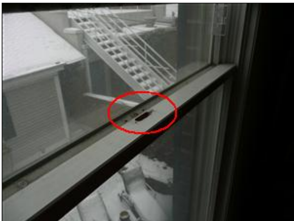
J. Picture 8 missing hardware, east BR
