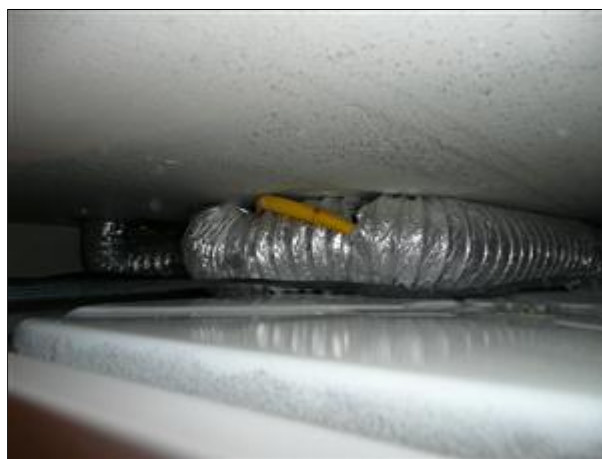
I. Picture 4 replace venting and gas supply routing
