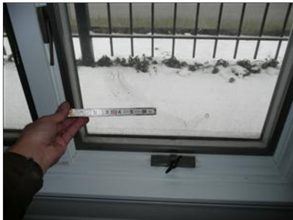
J. Picture 12 south windows along gangway
