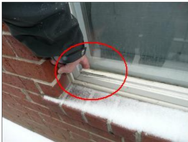
J. Picture 10 loose trim, south window @ gangway
