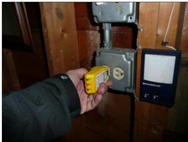
D. Picture 3 upgrade garage outlet(s)
