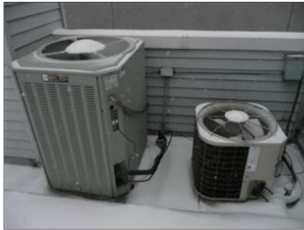
E. Picture 20 unable to test air conditioning; cover units when not in use
