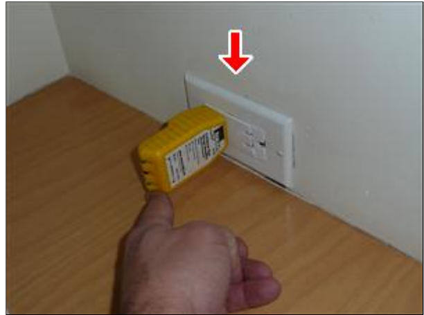
D. Picture 2 upgrade kitchen 'nook' outlets
