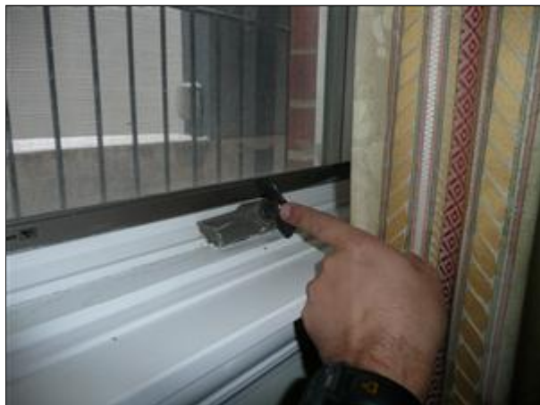
J. Picture 9 stripped casement operators
