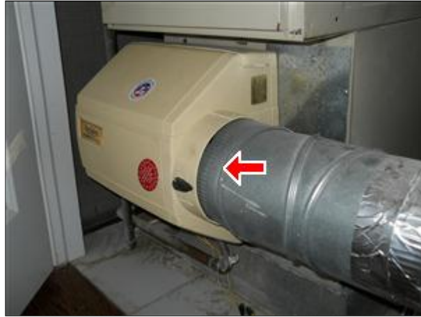
E. Picture 5 large gap at 2nd fl furnace
