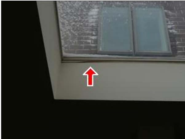
H. Picture 1 skylight trim buckling
