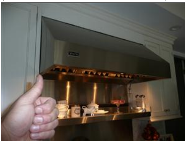
E. Picture 24 loud hood operation
