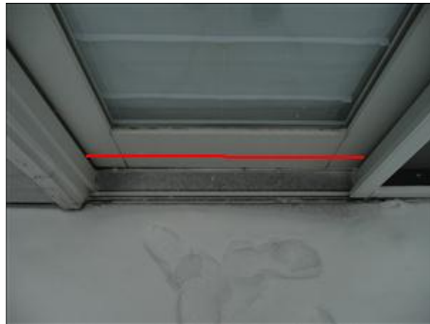
J. Picture 3 recommend drip caps
