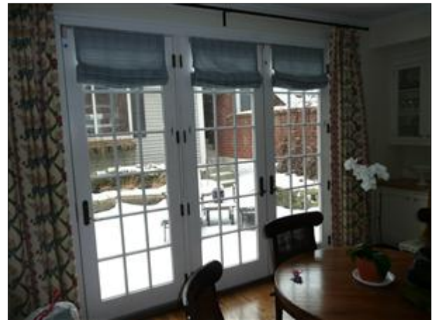
J. Picture 5 loose weatherstripping and fitment 1st fl rear
