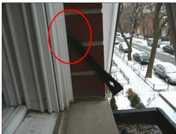
A. Picture 5 seal window trim gaps
