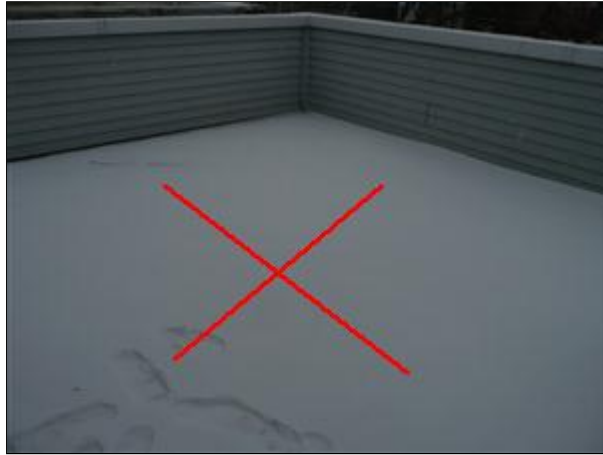
C. Picture 2 snow covered roof
