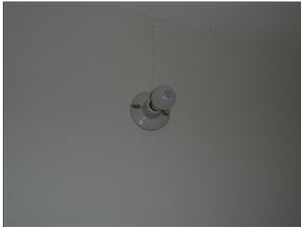
D. Picture 5 upgrade bare bulb fixtures @ closets
