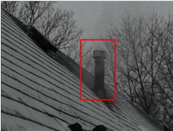
E. Picture 21 2nd fl furnace vent
