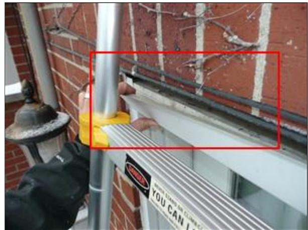
A. Picture 12 east door system header improperly installed/flashed; repair
