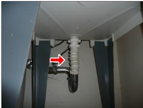
G. Picture 15 replace corrugated drain pipe
