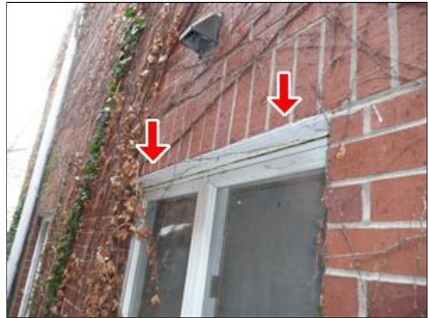
A. Picture 10 sealed lintels increase risk of moisture retention, structural damage
