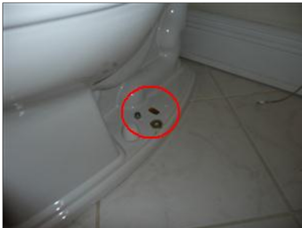
G. Picture 12 not seated toilet bolt
