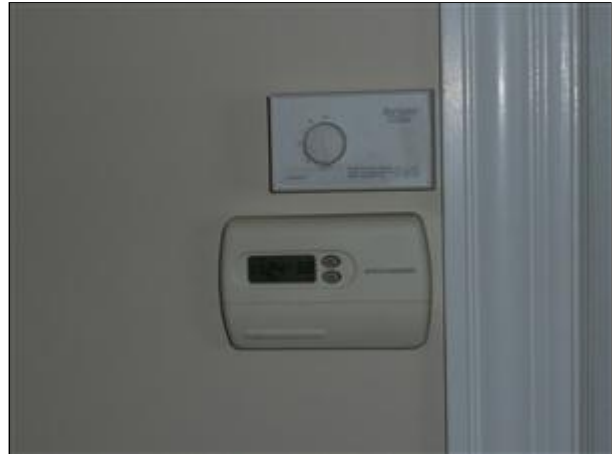
E. Picture 18 relocate t-stat of 2nd fl
