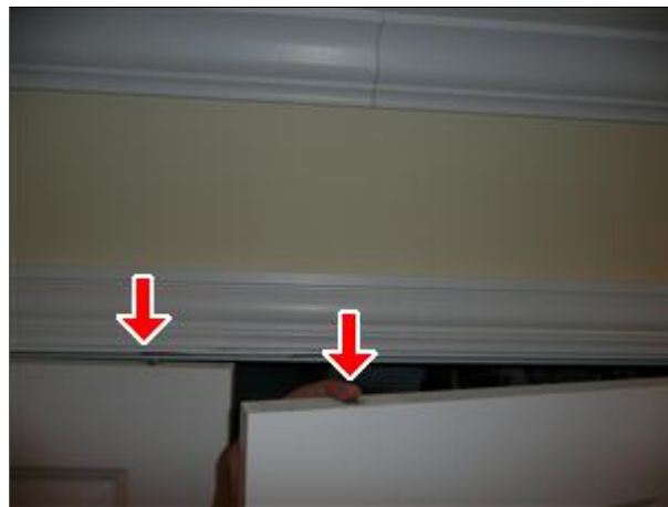
H. Picture 4 adjust closet ball catches for door fitment
