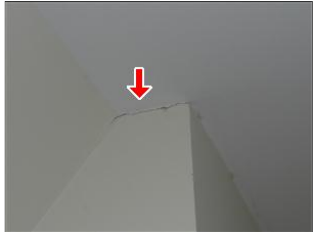
H. Picture 2 top floor drywall junction repairs required
