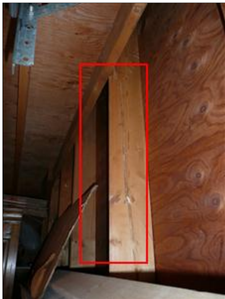
B. Picture 10 split and rotated stud, north wall
