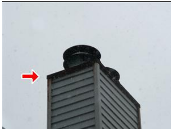
C. Picture 4 heavy rust of west metal crown
