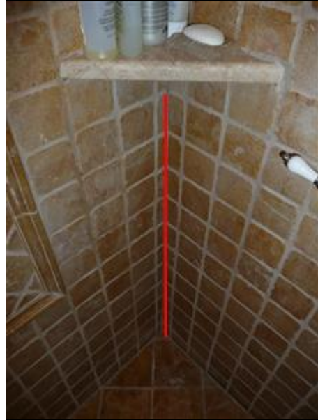
H. Picture 6 seal tile intersections, master shower
