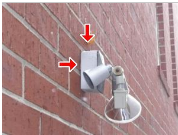
A. Picture 16 seal tops and sides of fixtures and outlets
