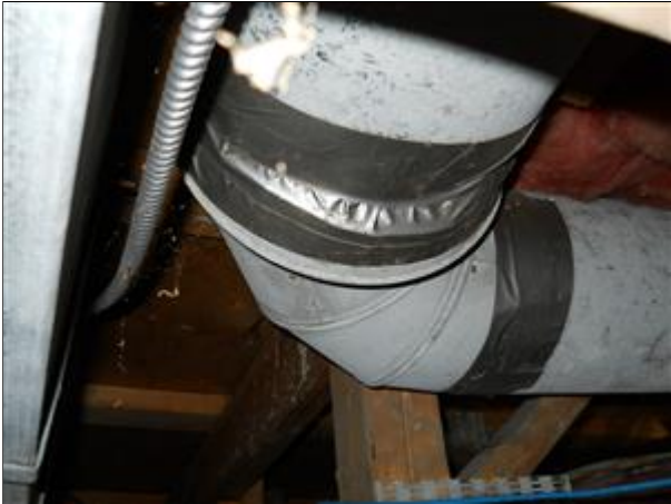
L. Picture 3 seal all duct joints with mastic or UL approved foil tape (spray foaming eliminates this step fyi)
