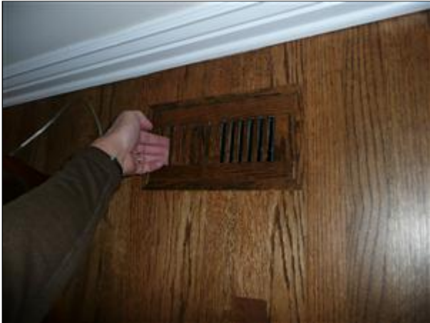
E. Picture 7 registers should be readily removable
