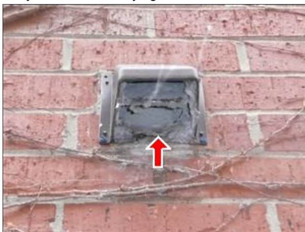
I. Picture 7 clean lint passages
