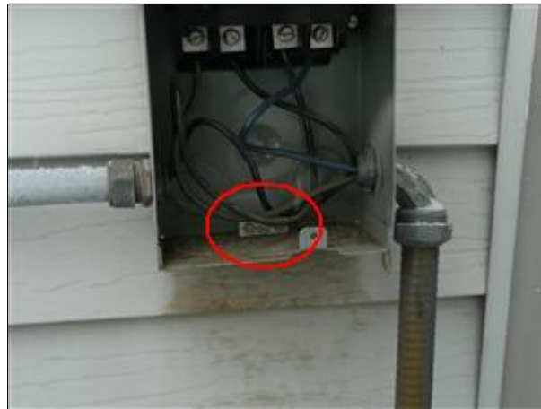
D. Picture 9 recommend grounding conductor
