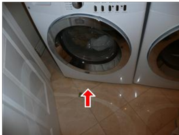
I. Picture 3 recommend drain pan
