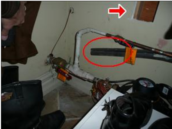
G. Picture 20 install well fitted pipe insulation, seal gaps/openings
