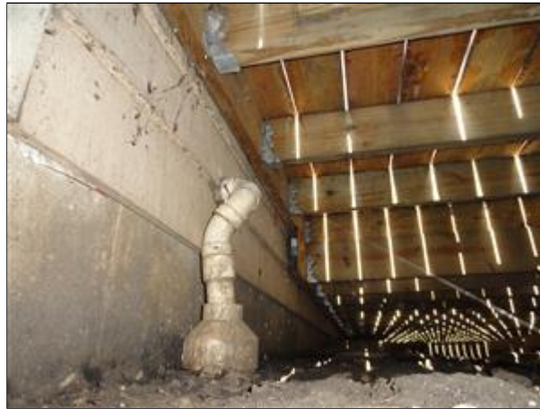
Item 17 - Picture 1 inconclusive view from gap at South
