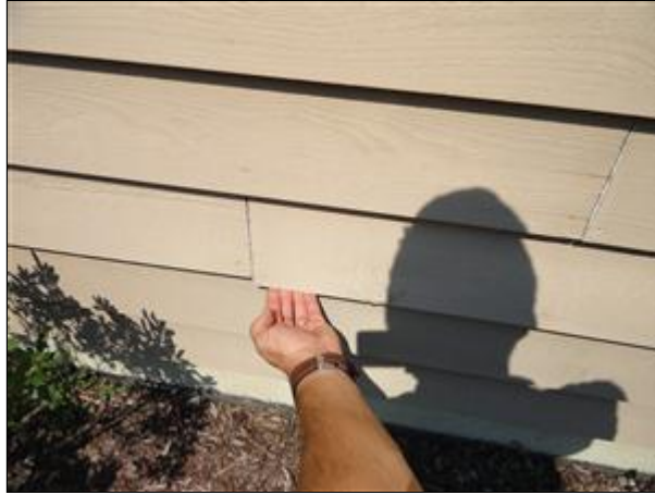
Item 1 - Picture 7 South siding near gas meter,
