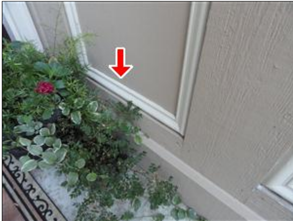
A. Picture 1 periodically inspect inset trim for water collection
