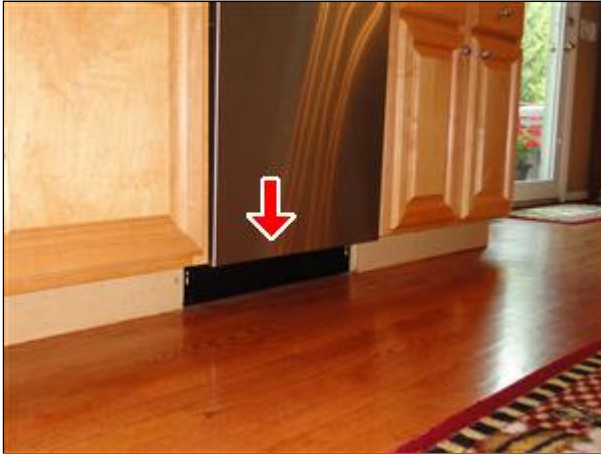
H. Picture 3 color matched toe kick for appearance recommended
