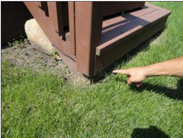
A. Picture 16 stringer termination not on concrete or stable surface
