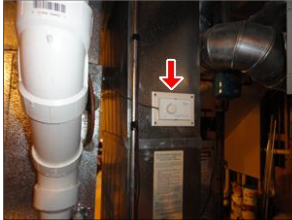
F. Picture 13 recommend relocation
