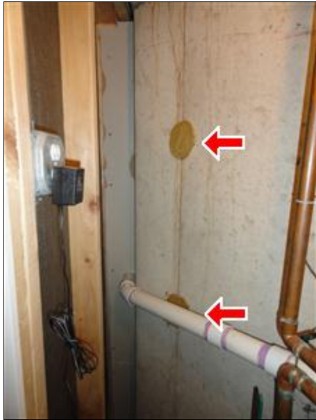
Item 19 - Picture 1 West basement
