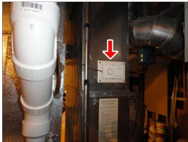
Item 33 - Picture 1 recommend relocation
