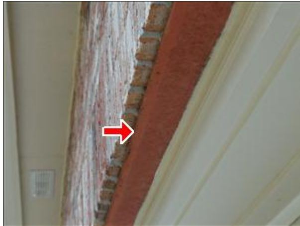
A. Picture 11 prep and finish paint lintels
