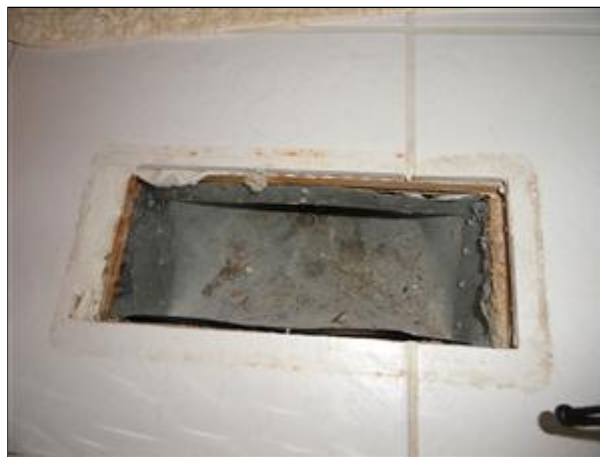
Item 27 - Picture 1 clean ductwork
