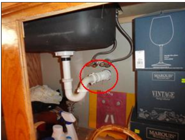
G. Picture 6 recommend replacing corrugated drain pipe with smooth wall metal, wet bar
