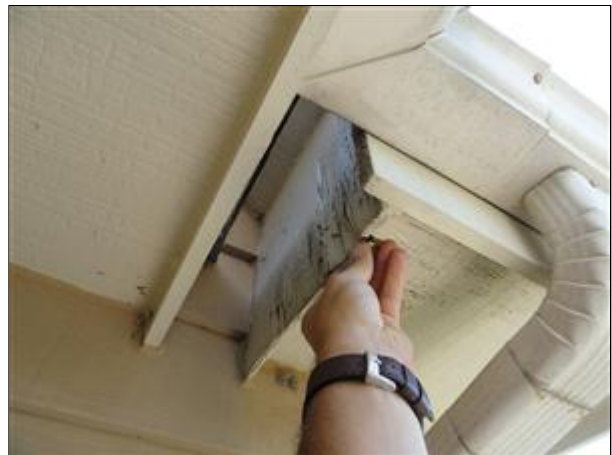
A. Picture 19 awkward routing of roof drainage
