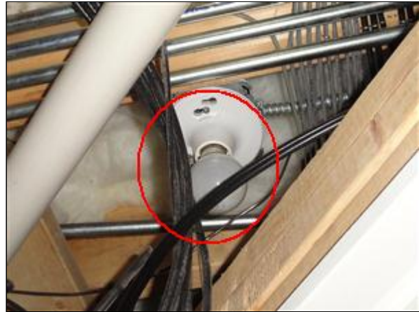
Item 22 - Picture 2 avoid bare bulb fixtures, risk of fire--upgrade to covered or low profile fluorescent (sump closet here)
