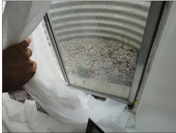
Item 55 - Picture 1 inefficient windows
