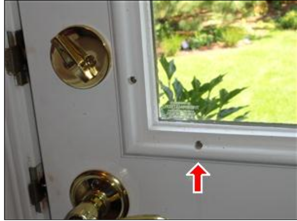
Item 42 - Picture 4 install button caps for appearance
