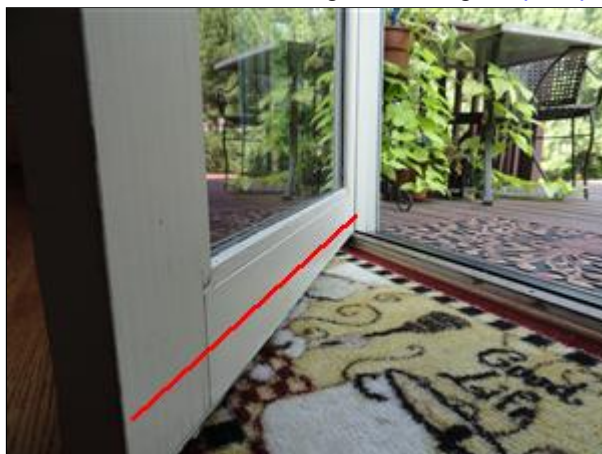
J. Picture 3 recommend drip cap
