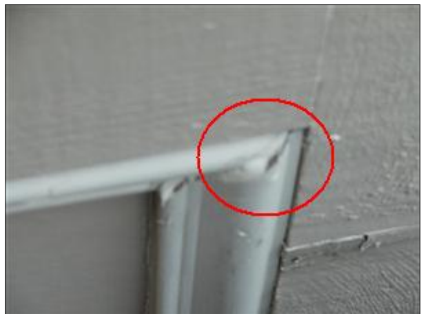
Item 1 - Picture 4 trim collections areas prone to moisture
