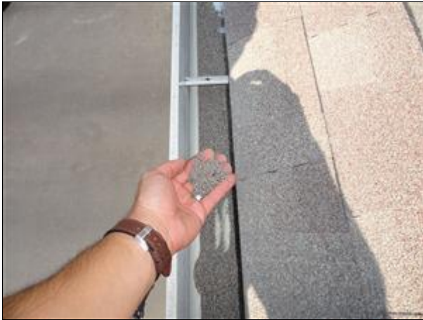
Item 13 - Picture 1 loss of protective granules, exposed fiberglass
