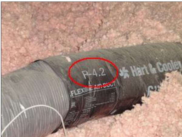
Item 26 - Picture 1 increased insulation and LESS flex duct use is recommended
