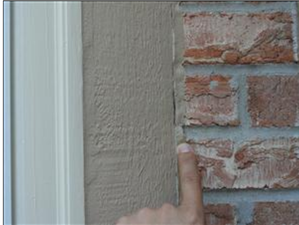
A. Picture 10 repair sealant joints as needed
