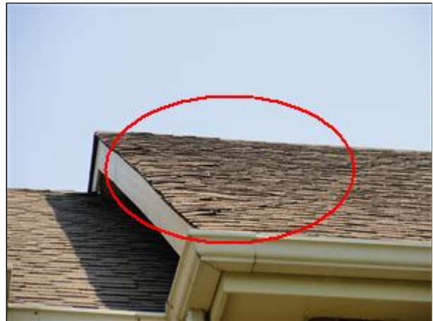
Item 13 - Picture 4 beginning shingle curling, indication of 'dying' shingle
