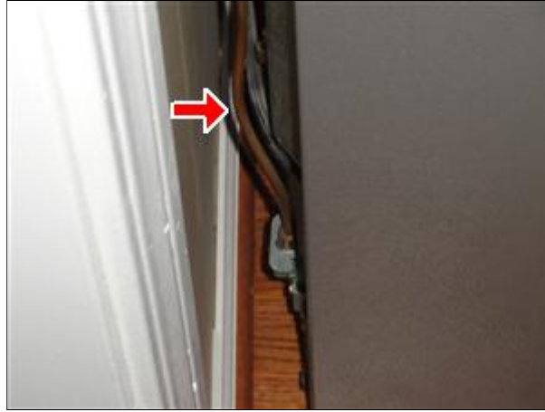
Item 49 - Picture 1 upgrade fridge supply
