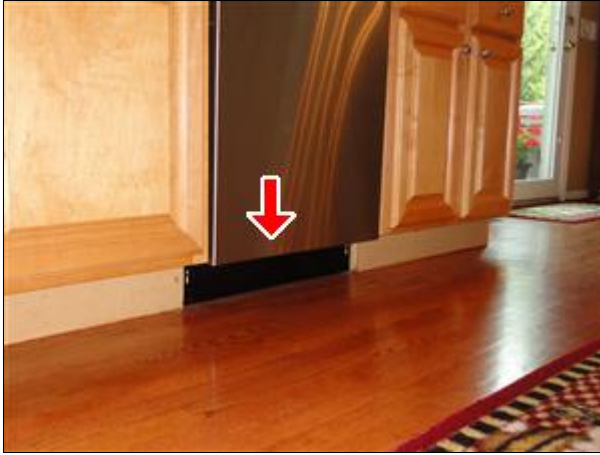
Item 42 - Picture 3 color matched toe kick for appearance recommended
