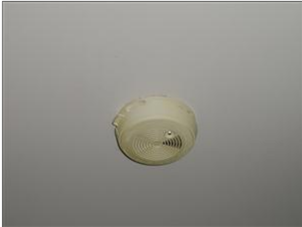
L. Picture 1 aged detectors, replace due to low cost vs critical function
