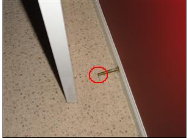
H. Picture 2 add rubber caps to avoid door damage
