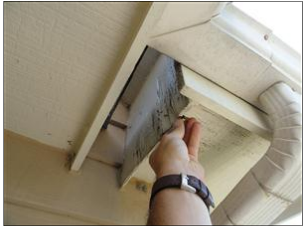
Item 8 - Picture 2 awkward routing of roof drainage
