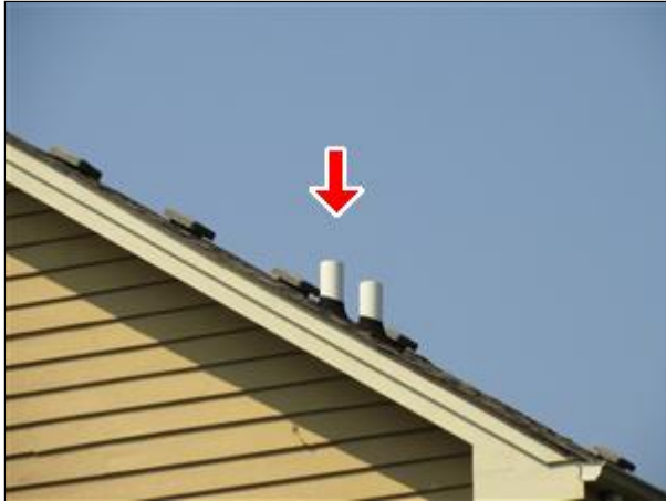
H. Picture 10 flashings may have degraded
