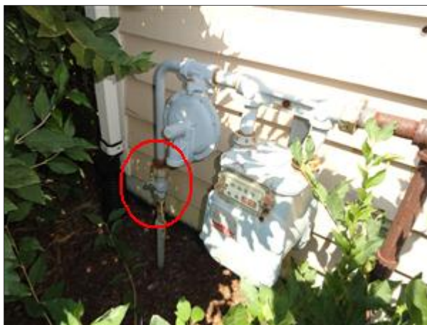
Item 35 - Picture 1 main gas shut-off
