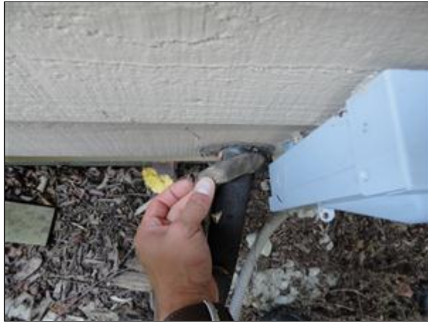
Item 6 - Picture 1 loose putty at a/c lineset
