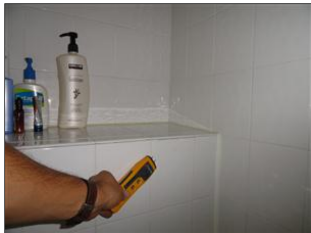
Item 43 - Picture 2 buried meter indicating saturation
