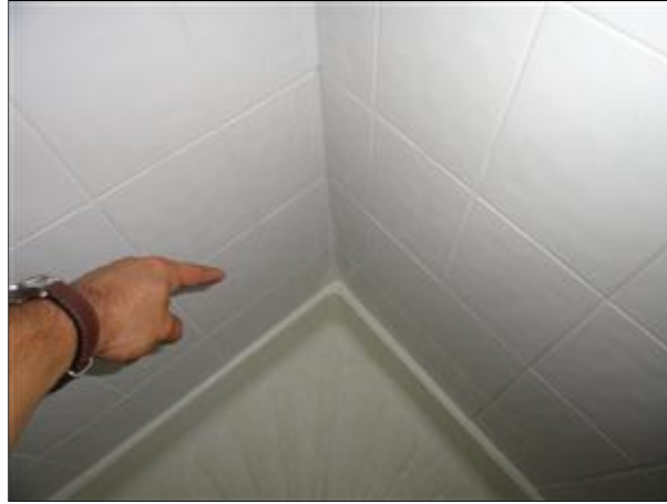
Item 43 - Picture 3 reseal shower junctions
