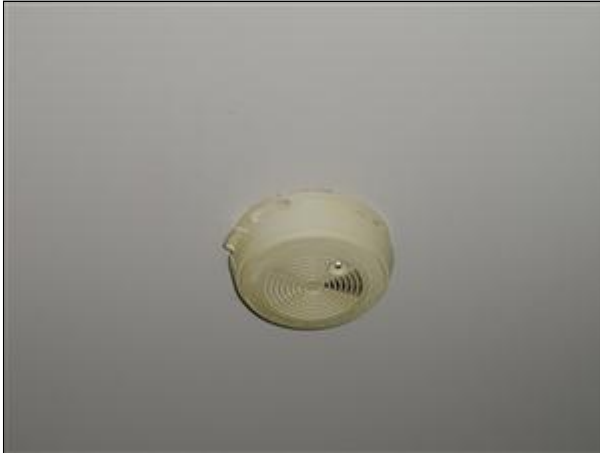
Item 57 - Picture 1 aged detectors, replace due to low cost vs critical function
