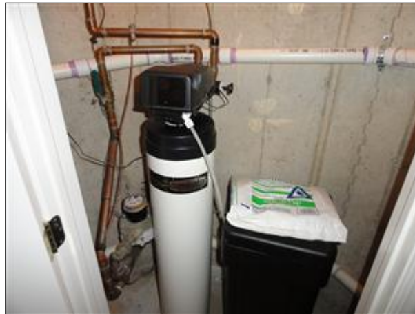
Item 39 - Picture 1 water softener
