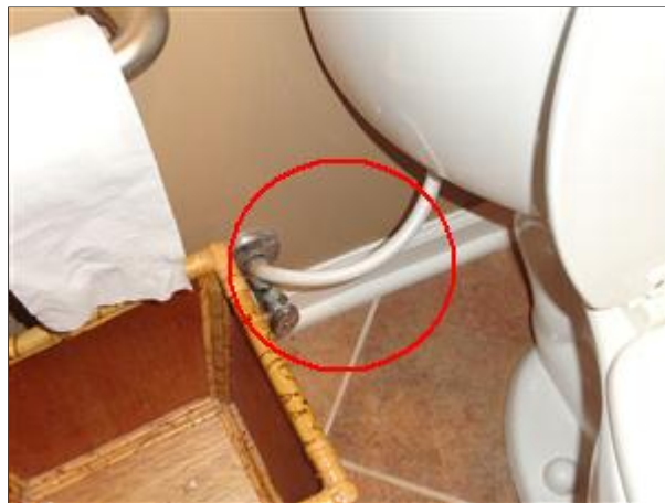
Item 40 - Picture 1 basement toilet line
