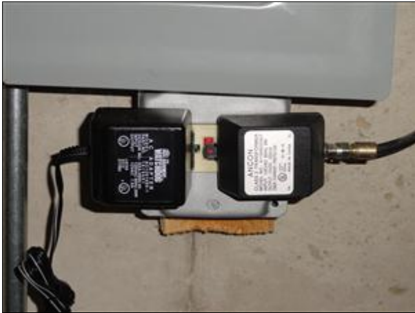
E. Picture 5 sump pump GFCI
