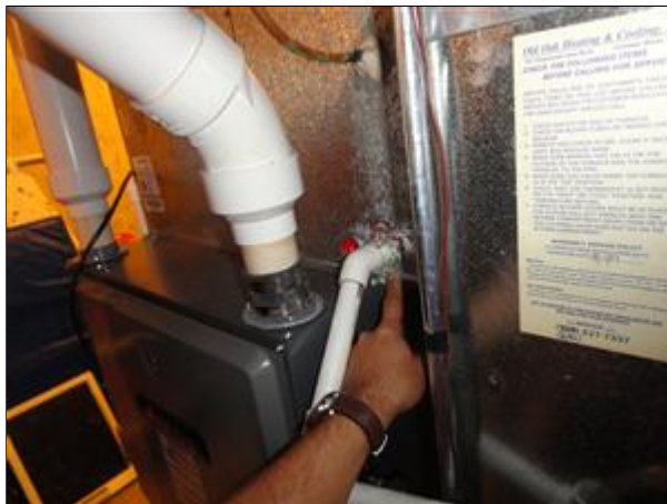
Item 34 - Picture 1 seal entry points
