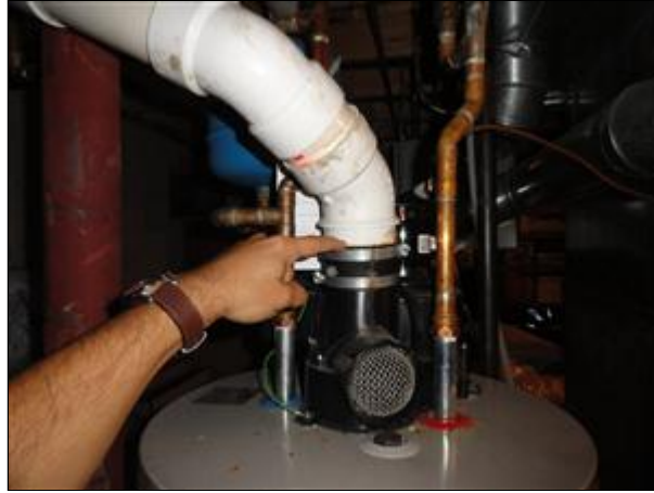
G. Picture 8 condensate 'roll back' after exhaust operation, not threatening
