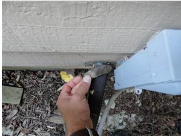
A. Picture 13 loose putty at a/c lineset
