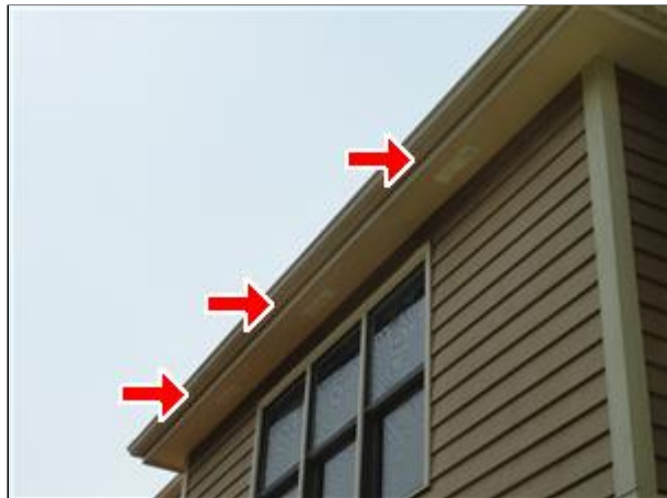
Item 16 - Picture 2 recommend increased soffit ventilation
