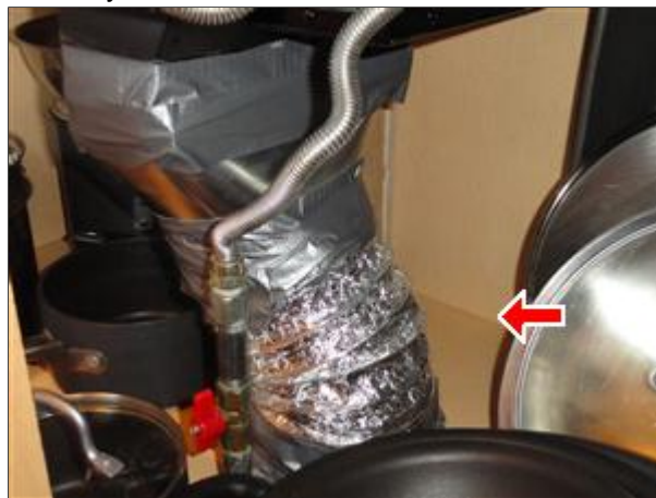
Item 48 - Picture 1 upgrade venting
