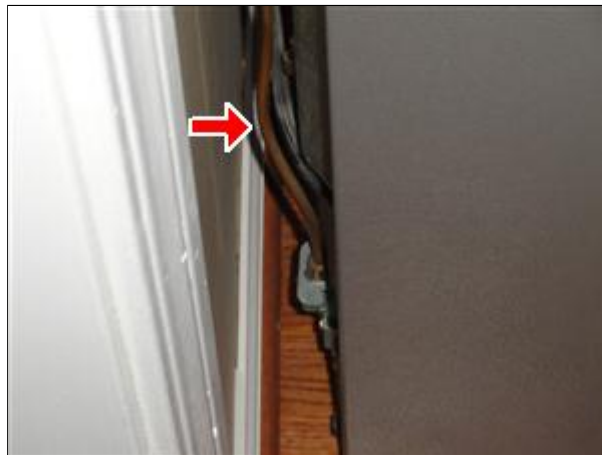
I. Picture 2 upgrade fridge supply
