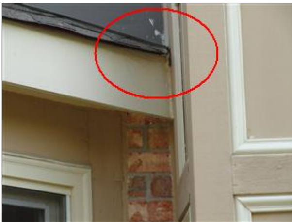
A. Picture 3 recommend diverter flashing and/or modified gutter and downspout to avoid splashing/saturation at front bay
