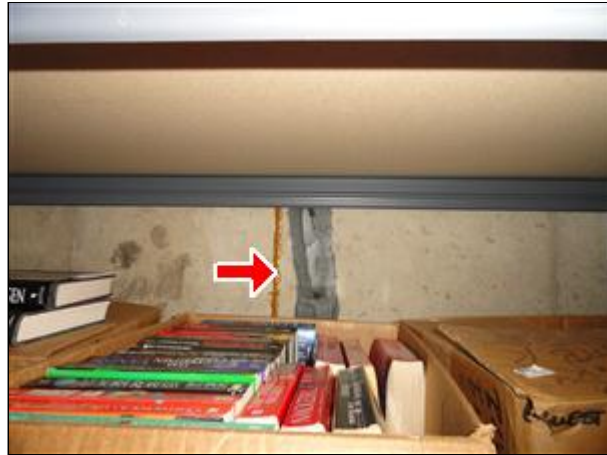
Item 19 - Picture 2 East basement foundation repairs
