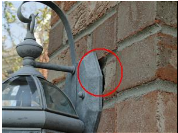
Item 2 - Picture 2 North garage
