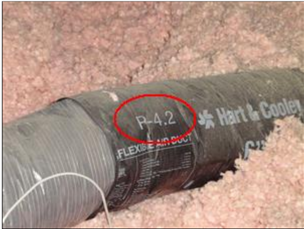
F. Picture 6 increased insulation and LESS flex duct use is recommended
