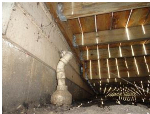
D. Picture 1 inconclusive view from gap at South
