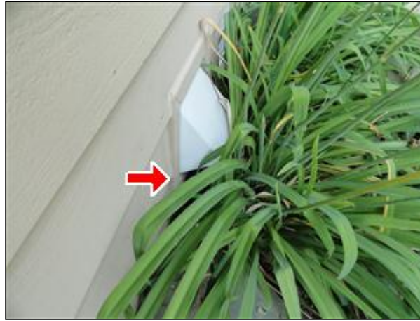
Item 25 - Picture 1 risk of choking off pathways
