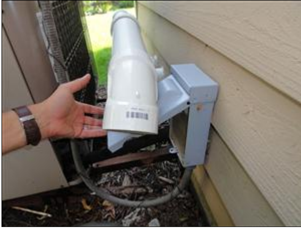
Item 24 - Picture 1 poor installation
