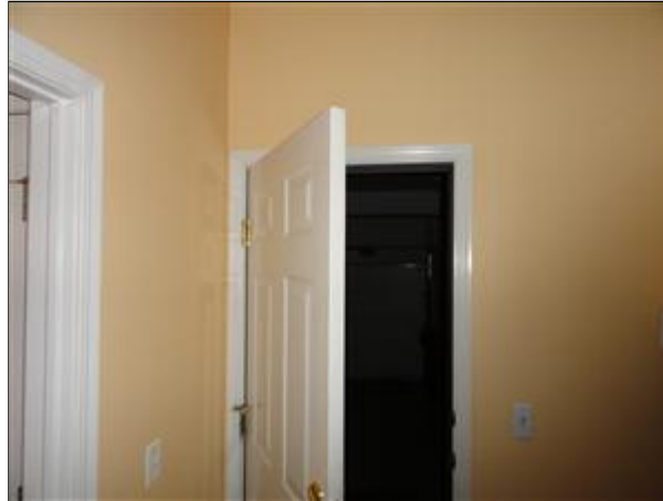
Item 11 - Picture 1 adjust already present spring loaded hinges
