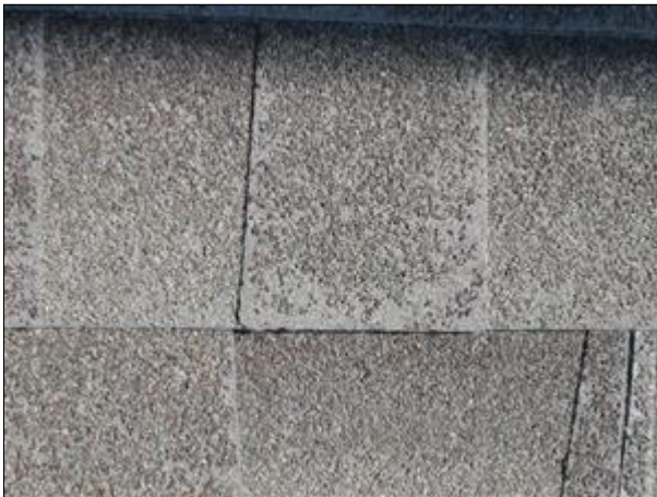
Item 13 - Picture 3 note shingle wear
