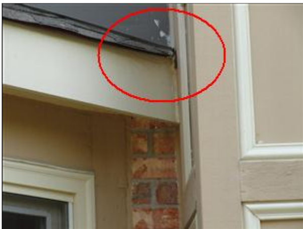
Item 1 - Picture 3 recommend diverter flashing and/or modified gutter and downspout to avoid splashing/saturation at front bay
