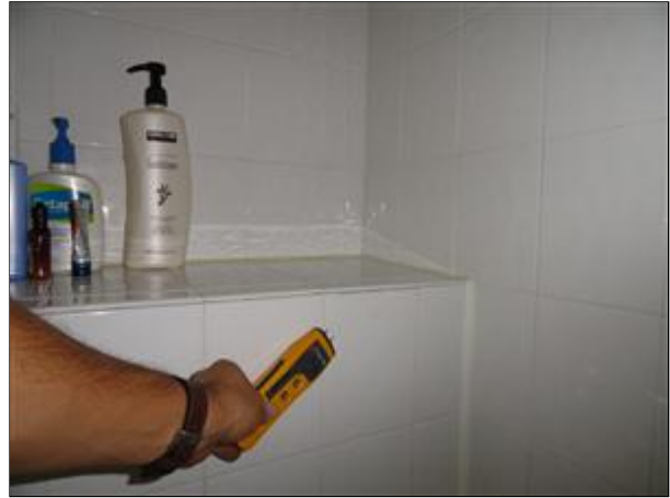
H. Picture 7 buried meter indicating saturation
