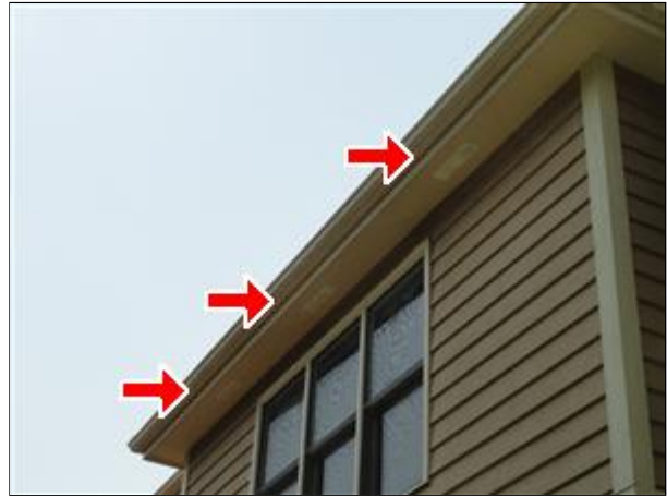
C. Picture 8 recommend increased soffit ventilation
