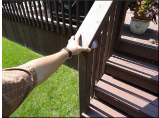
A. Picture 15 loose handrail
