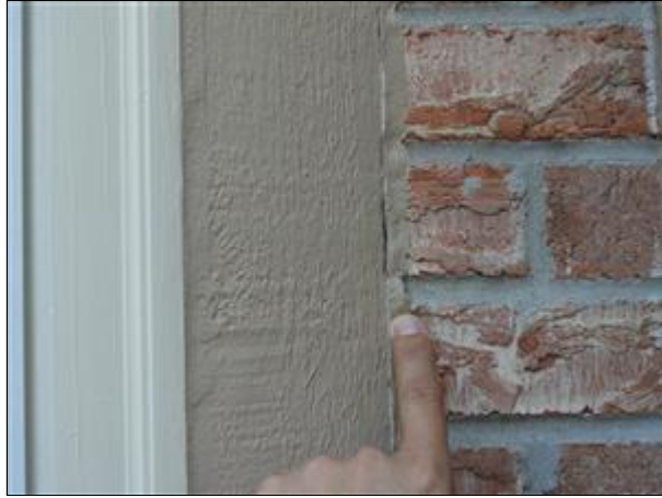
Item 3 - Picture 1 repair sealant joints as needed
