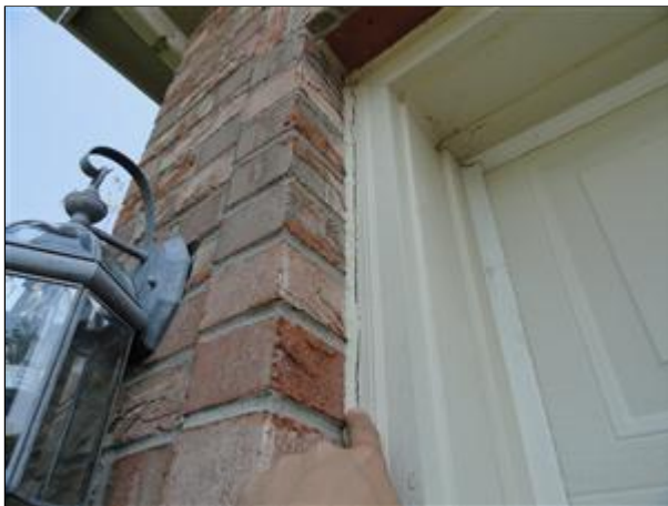
A. Picture 5 aged sealant, garage i.e.
