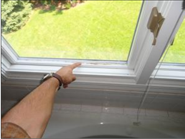
H. Picture 1 wood deterioration, master bath
