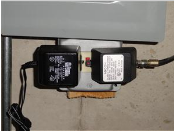
Item 22 - Picture 1 sump pump GFCI
