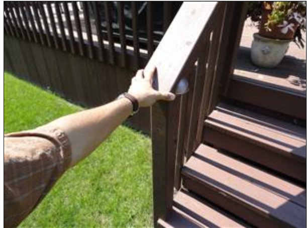
Item 7 - Picture 2 loose handrail
