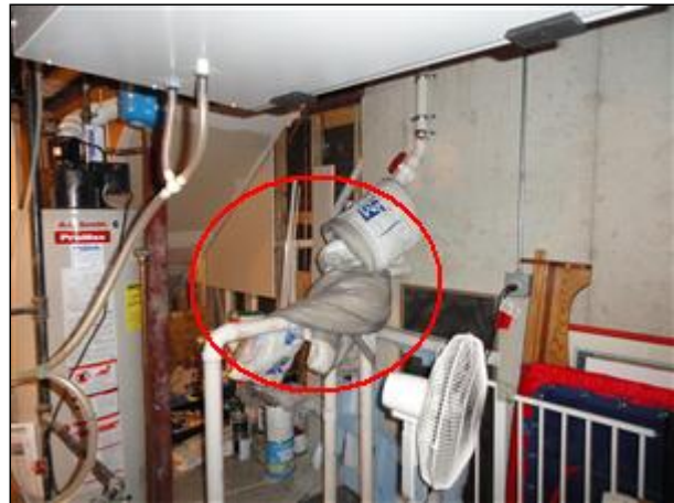
Item 36 - Picture 6 install add'l supports for ejector pit piping to avoid 'hammer' and risk of leaking
