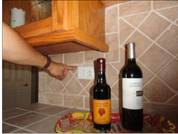
Item 20 - Picture 3 secure loose receptacle, wet bar
