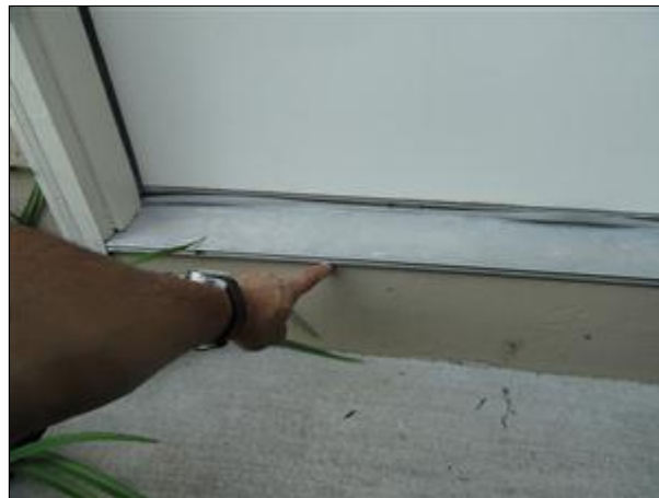
J. Picture 1 laundry door
