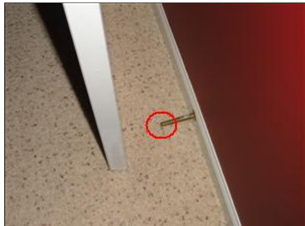
Item 42 - Picture 2 add rubber caps to avoid door damage
