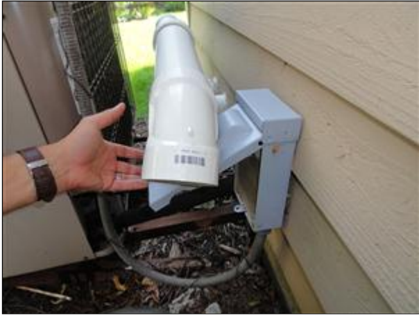
F. Picture 3 poor installation
