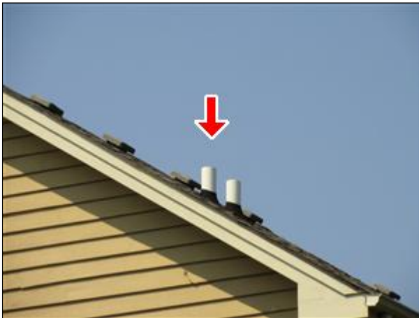
Item 45 - Picture 1 flashings may have degraded
