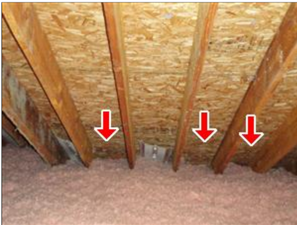
Item 16 - Picture 1 increase ventilation
