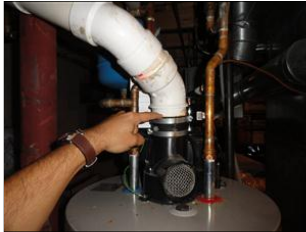
Item 36 - Picture 7 condensate 'roll back' after exhaust operation, not threatening
