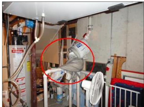
G. Picture 7 install add'l supports for ejector pit piping to avoid 'hammer' and risk of leaking
