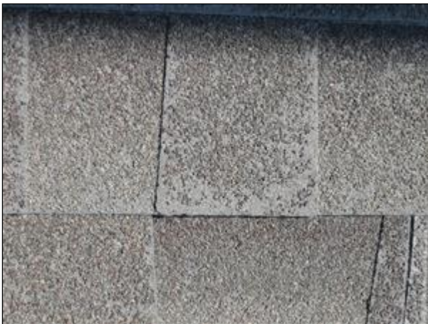
C. Picture 3 note shingle wear
