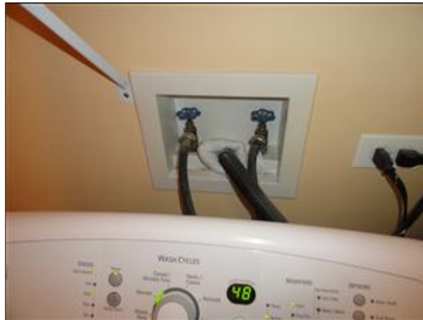
Item 51 - Picture 1 upgrade washer hoses
