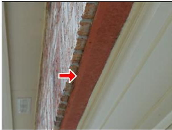
Item 4 - Picture 1 prep and finish paint lintels
