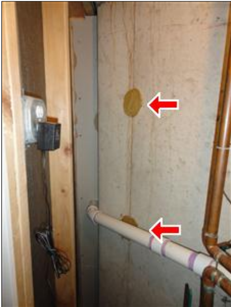
D. Picture 3 West basement
