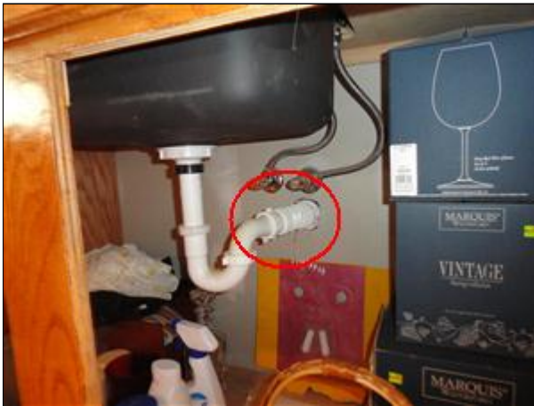
Item 36 - Picture 5 recommend replacing corrugated drain pipe with smooth wall metal, wet bar
