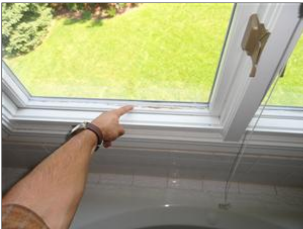
Item 42 - Picture 1 wood deterioration, master bath
