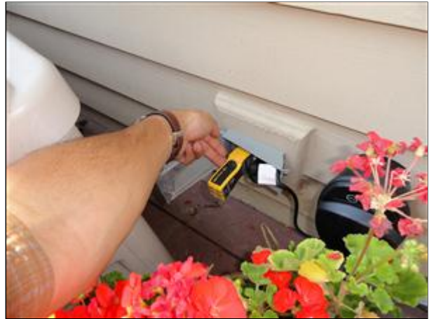
E. Picture 2 deck, improper horizontal cover orientation
