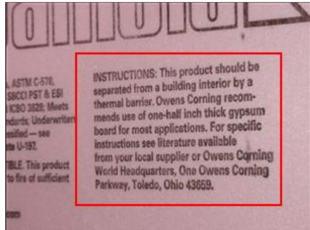
Item 56 - Picture 2 required fire suppression (typ. 5/8' drywall)
