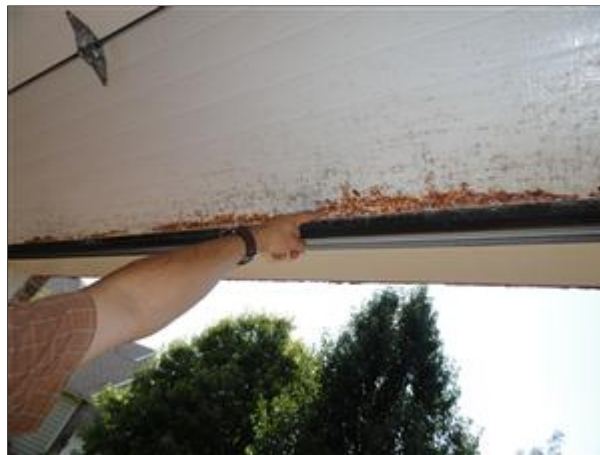
Item 12 - Picture 1 door rust at bottom panel
