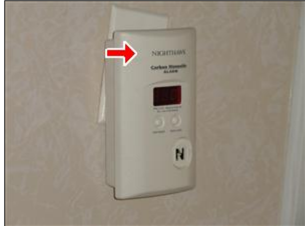
Item 57 - Picture 2 manufacturer/model with high rate of failure
