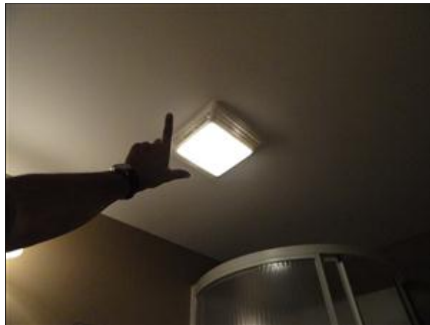
F. Picture 12 repair/replace bath fan
