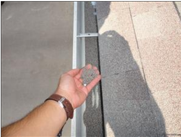
C. Picture 1 loss of protective granules, exposed fiberglass
