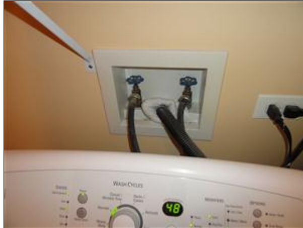
I. Picture 4 upgrade washer hoses
