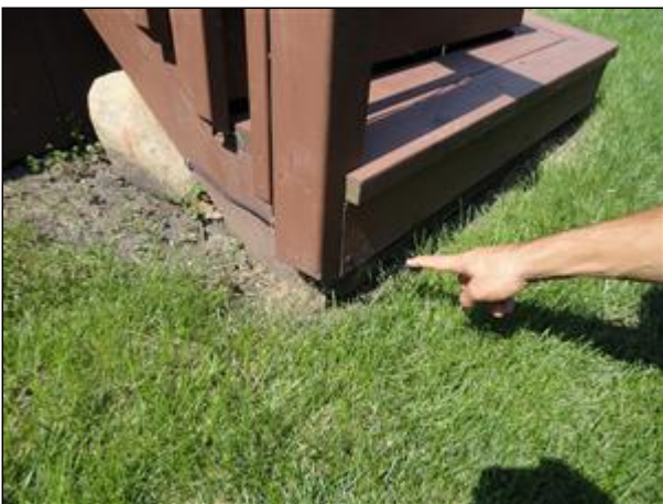
Item 7 - Picture 3 stringer termination not on concrete or stable surface
