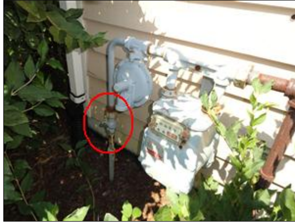
G. Picture 1 main gas shut-off
