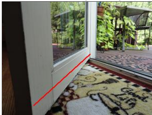
Item 54 - Picture 1 recommend drip cap
