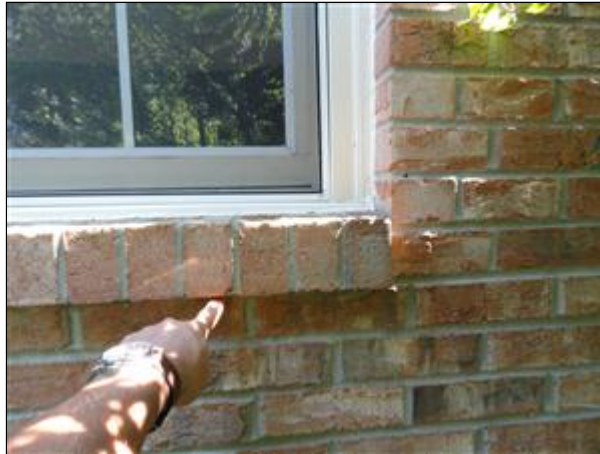
Item 9 - Picture 1 minimal pitch sills
