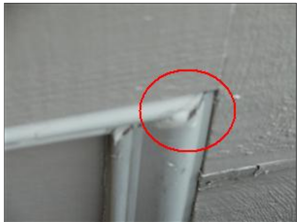
A. Picture 4 trim collections areas prone to moisture
