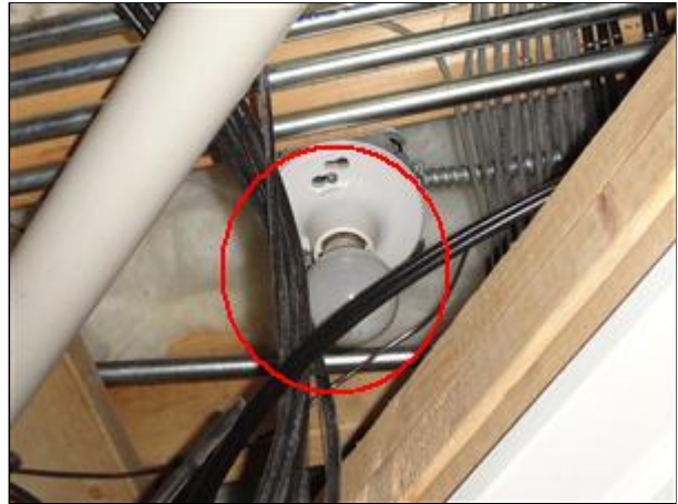
E. Picture 6 avoid bare bulb fixtures, risk of fire-- upgrade to covered or low profile fluorescent (sump closet here)
