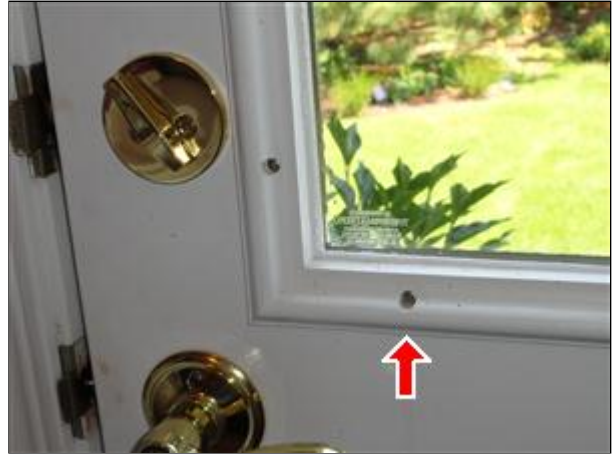
H. Picture 4 install button caps for appearance
