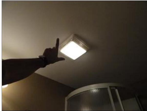
Item 32 - Picture 1 repair/replace bath fan
