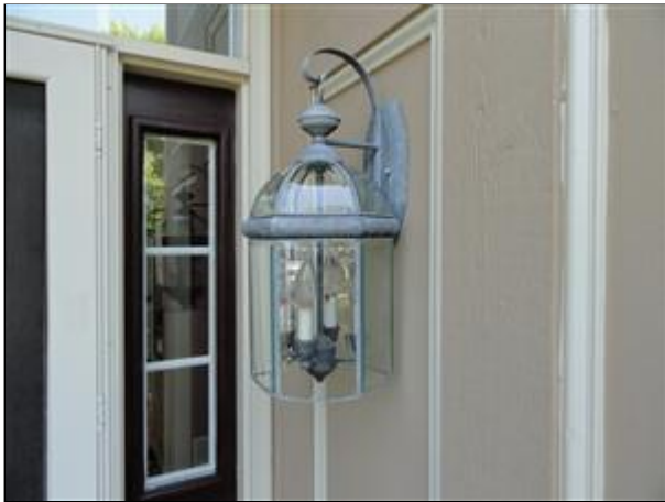
Item 2 - Picture 1 seal exterior electrical fixtures
