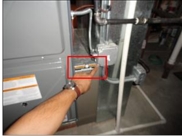
Item 24 - Picture 2 difficult to remove filter access panel
