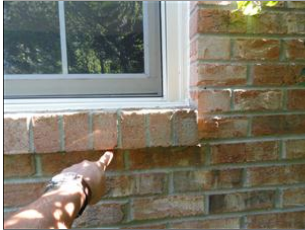
A. Picture 20 minimal pitch sills
