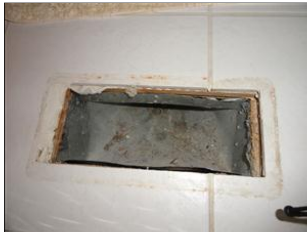
F. Picture 8 clean ductwork
