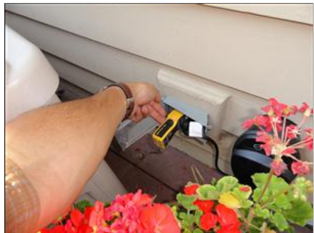
Item 20 - Picture 2 deck, improper horizontal cover orientation
