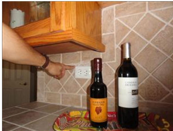
E. Picture 3 secure loose receptacle, wet bar
