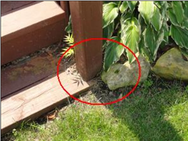
Item 7 - Picture 1 stringer/post/tread soil contact
