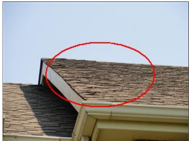
C. Picture 4 beginning shingle curling, indication of 'dying' shingle
