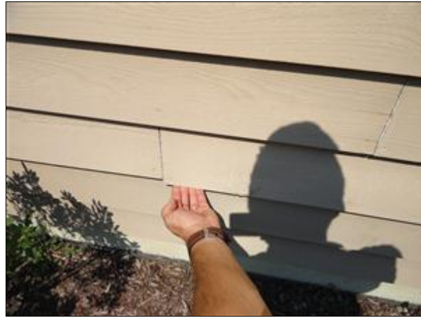
A. Picture 7 South siding near gas meter,
