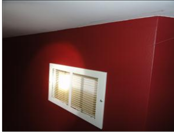
Item 30 - Picture 1 panned ductwork
