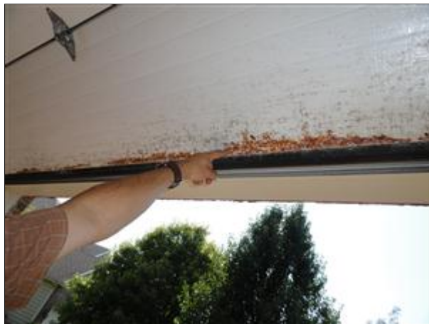
B. Picture 3 door rust at bottom panel
