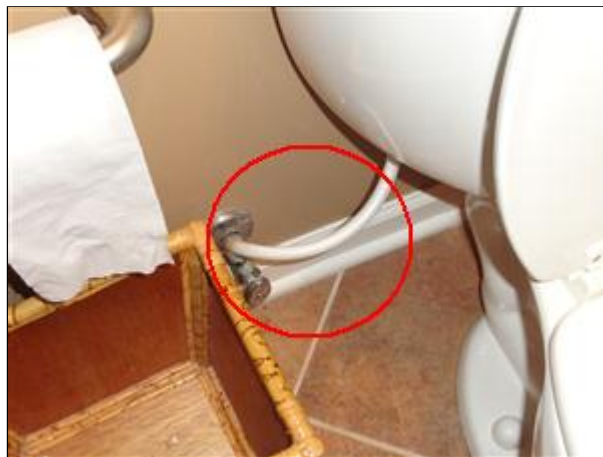
G. Picture 12 basement toilet line
