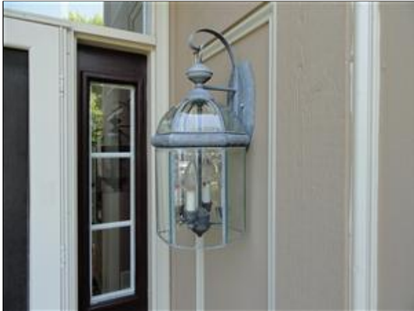
A. Picture 8 seal exterior electrical fixtures
