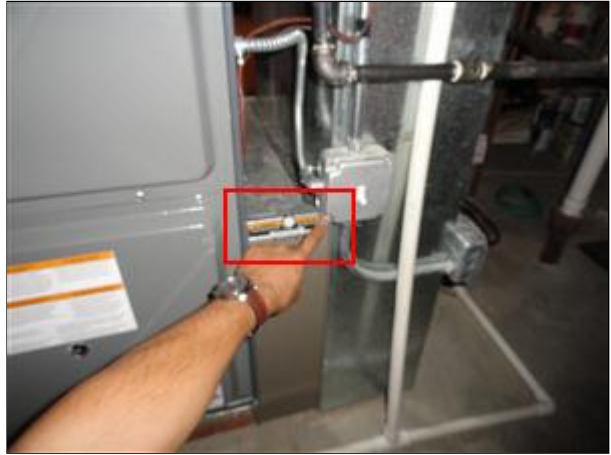
F. Picture 4 difficult to remove filter access panel
