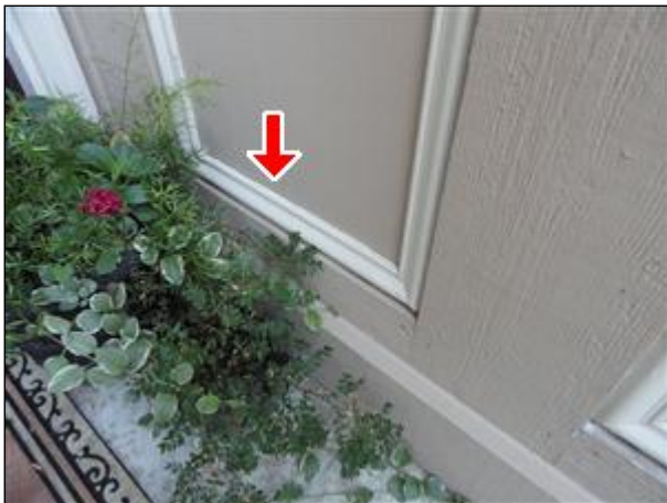
Item 1 - Picture 1 periodically inspect inset trim for water collection
