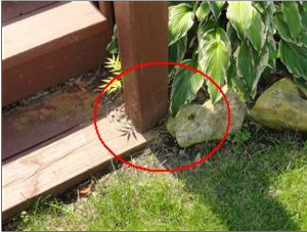
A. Picture 14 stringer/post/tread soil contact
