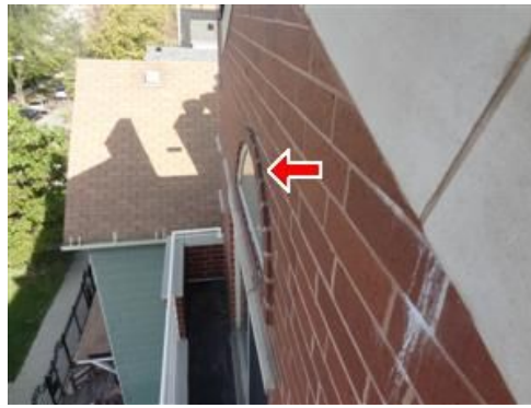
A. Picture 30 Projecting Soldier Course at Arch Top Window
