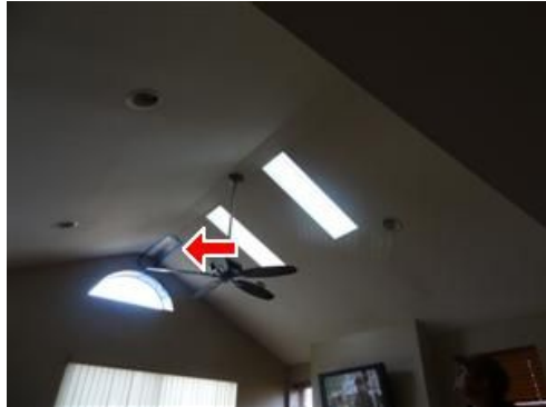
E. Picture 2 Cathedral ceiling at Unit 3N
