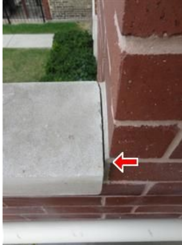
A. Picture 4 Limestone Mortar Joint
