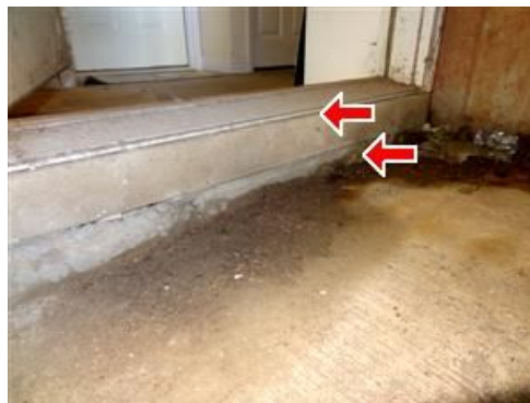
A. Picture 16 Rear Basement Entry Door
